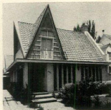
TUDOR ROOF brought up to date. House of Sr. Jorge Lake, Santiago.
