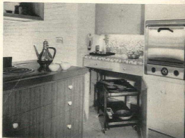
8. SWINGING DOORS ON CART GARAGE
