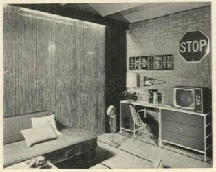
The dramatic sawtooth ceiling of a remodeled room for a boy is made of smooth steel panels precovered in a textured vinyl coating. No joists are needed; instead a steel "I" beam running across the window wall holds up the ceiling. Sliding glass doors are framed in metal with an enamel finish which needs no painting. The vinyl floor requires only a few hours to install over plywood.
