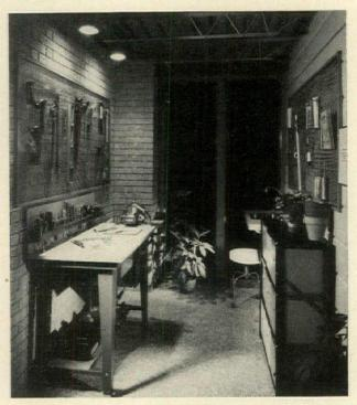
Like large-scaled tinker toys, these painted steel bar joists and vinyl-coated corrugated roof panels are bolted together to make both the ceiling and roof for a workshop addition to a house. The new wall is made up of 1/2-inch thick bricks composed of plastic and masonry granules; you merely nail them to a wood frame. Because of the wall's light weight, no heavy foundation is necessary.
