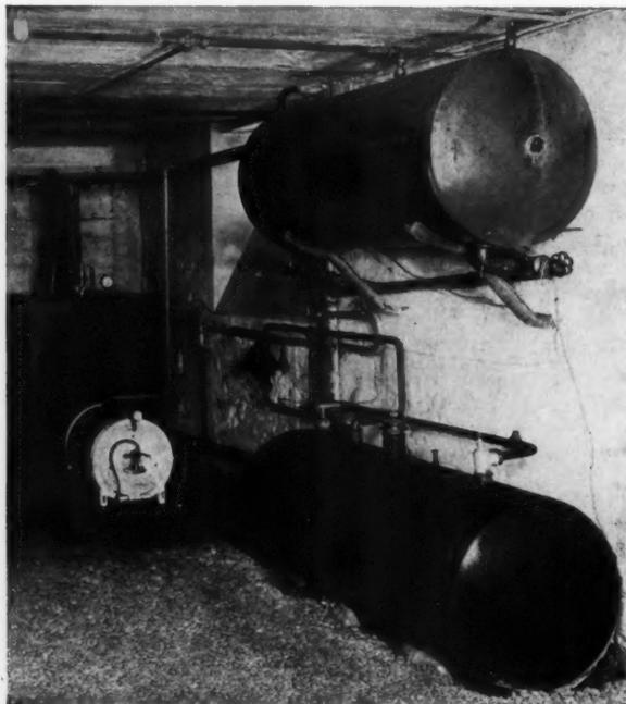
FIG. 2. CHAUFFERIE D'UN HOTEL PARTICULIER (PETITE CHAUDIÈRE AVEC BRÛLEUR SEMI-AUTOMATIQUE).
