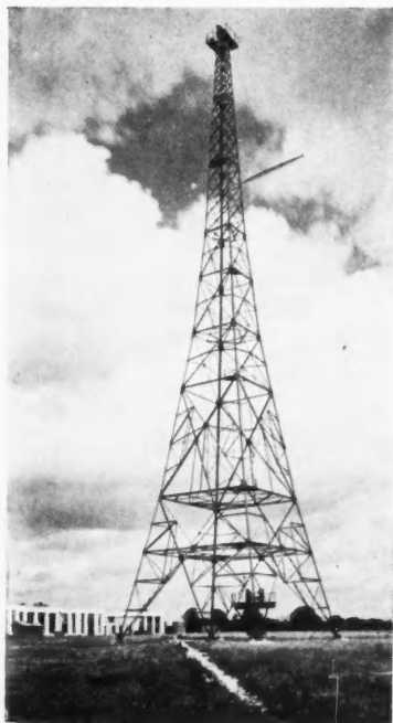
7. PYLONE DE BROOKMAN'S PARK (Londres)
