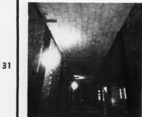
COFFRAGE DOUBLE PLANCHER.
