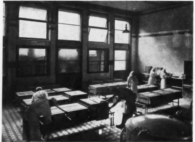
Photos: Arch. Assistance Publique Paris HOPITAL DE BROUSSAIS: CAISSES CHAUFFANTES
