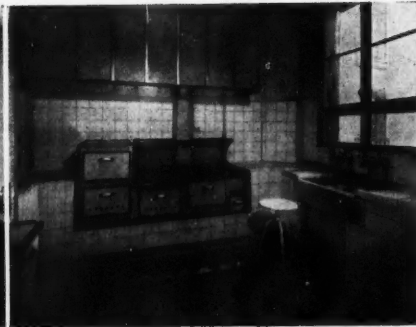
Grande cuisine. Install. Ch. BLANC
