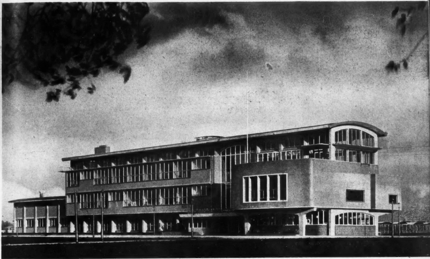
LE BATIMENT PRINCIPAL COTE ENTREE
