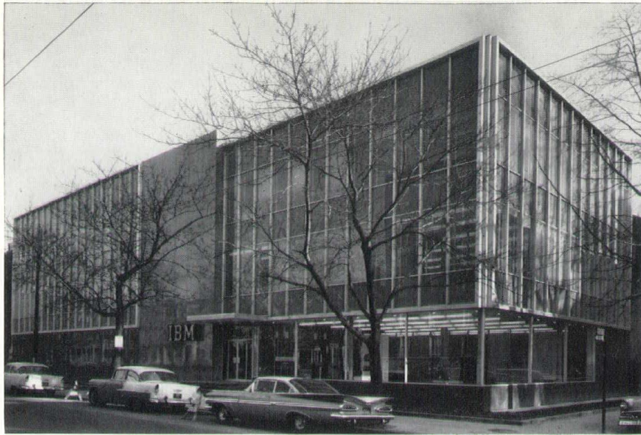
ALUMINUM AND GLASS CURTAIN WALL AT THE NEW IBM BUILDING, CAMBRIDGE STREET, CAMBRIDGE
