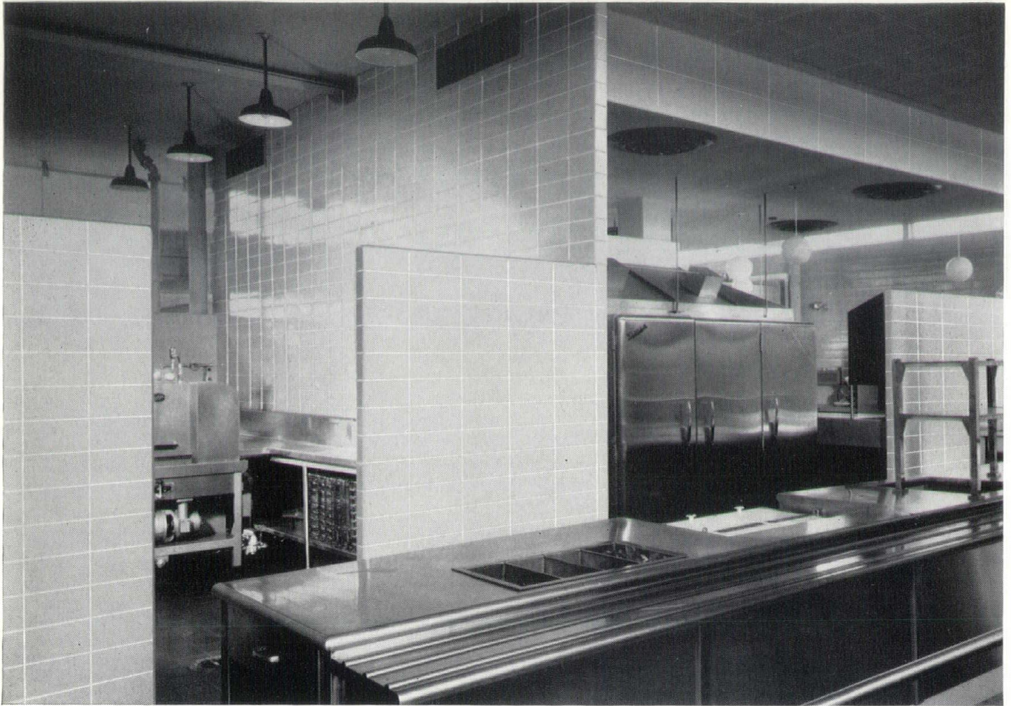
View of the new Westwood, Massachusetts, Senior High School cafeteria showing sanitary Natco Vitritile walls.
