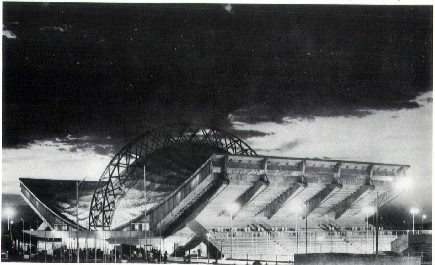
This 4,000-seat sports arena built in Barcelona, Venezuela, represents the first reported use of a suspended roof in that country.
