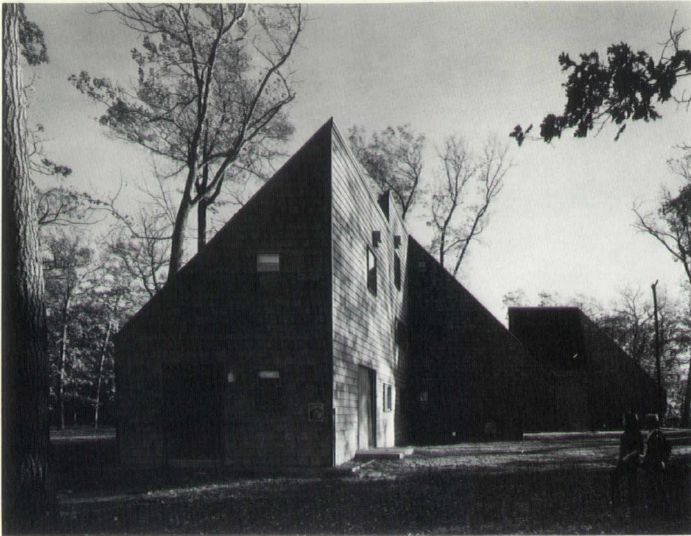
The 45 degree pitched roof proved a happy compromise, for both aesthetic and practical purposes. It utilizes the space above the ceiling line, or the floor line, which divides the triangular unit from the box unit at the base.
