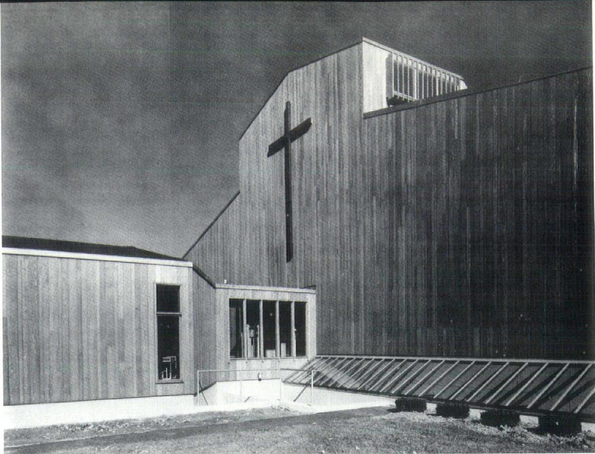
The lower level features a large social hall which is lit by a continuous skylight, which floods the space with sunshine. The ground-level skylight is visible (above) in this view toward the glassed-in bridge between the Eucharist Hall and Chapel.
