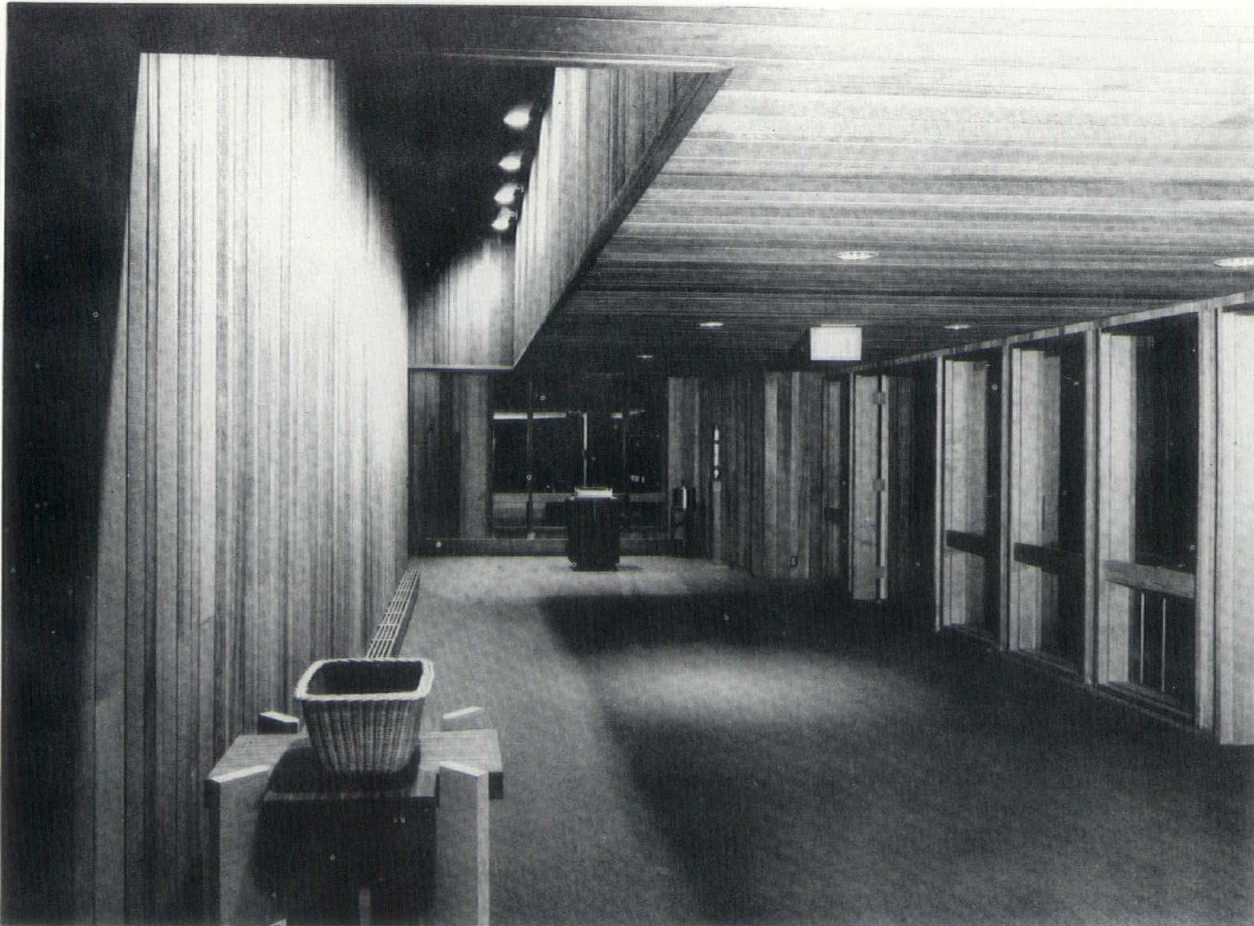
Vertical rough sawn random width cedar boards were used for interior paneling as well as for exterior sheathing. Varied brown colored carpet was used throughout the church, praised widely as "The cedar-scented shrine at the foot of Mount Katahdin."
