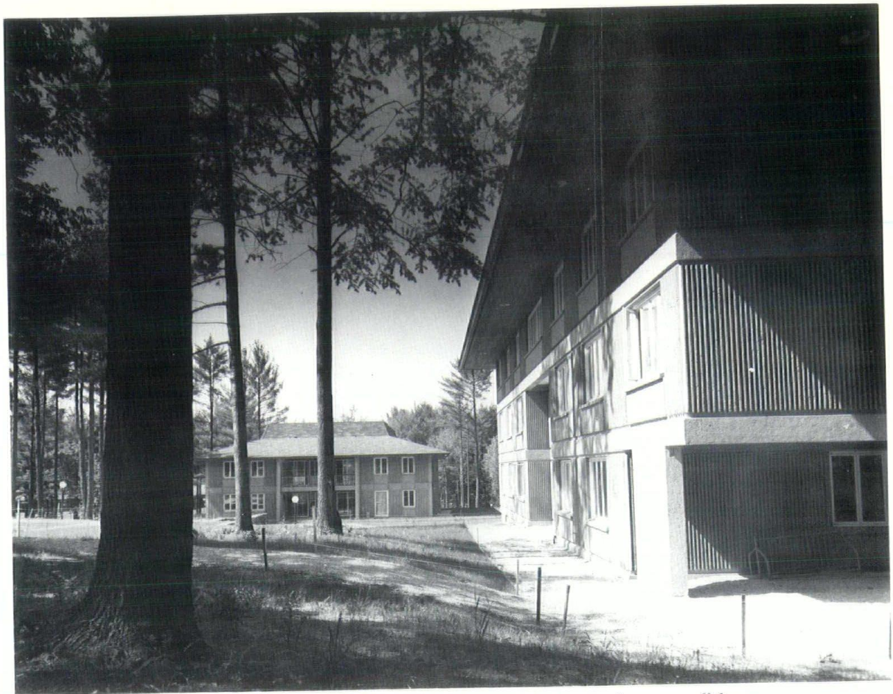
Identical formed, sand-blasted concrete bearing walls permitted successive re-use of custom wall forms.
