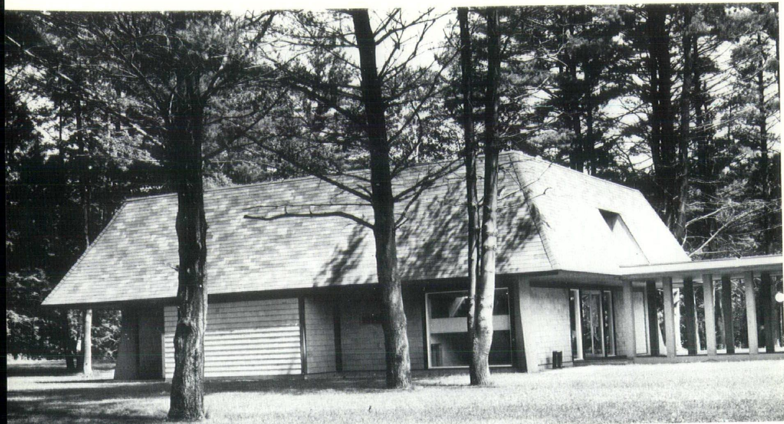
Construction last year of the Recitation Hall (above) marked the official completion of Phase I.
