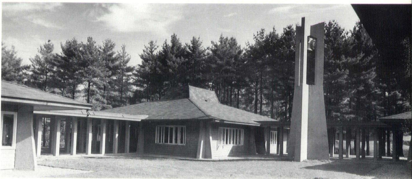
The Bell Tower between the Library Building (right) and Classroom Building One (center) is actually a stack, a vent for the gas furnaces in the library complex.
