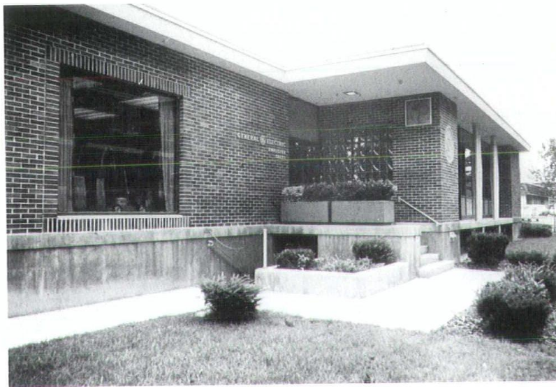
The exterior of the building is a chocolate colored wirecut brick.
