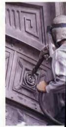
Because of its hardness, cast iron is one of the most appropriate surfaces for blasting.
