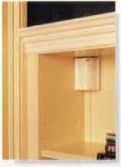
The motion detector's plastic case can be painted, but do not cover the lens.
