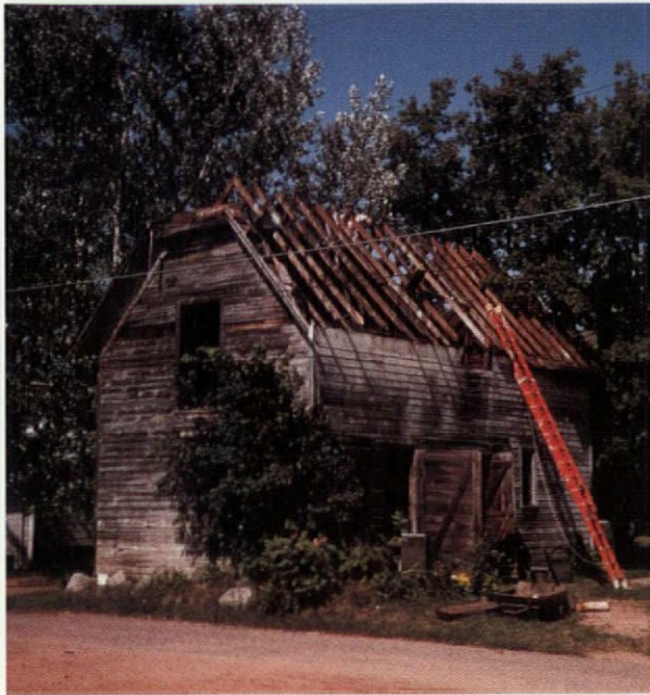
We disassembled the dormer piece-by-piece, so that we could put it back together in its original form.
