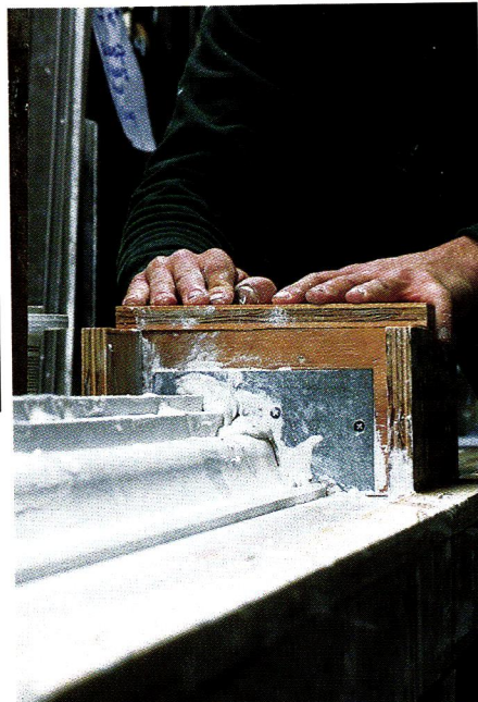
Top right: To fill the surface for the final runs, Dave points out minor blemishes and craters while Frank brushes them with soupy plaster. Another pass or two of the knife with a "baptizing" of water give the moulding its finished polish.
