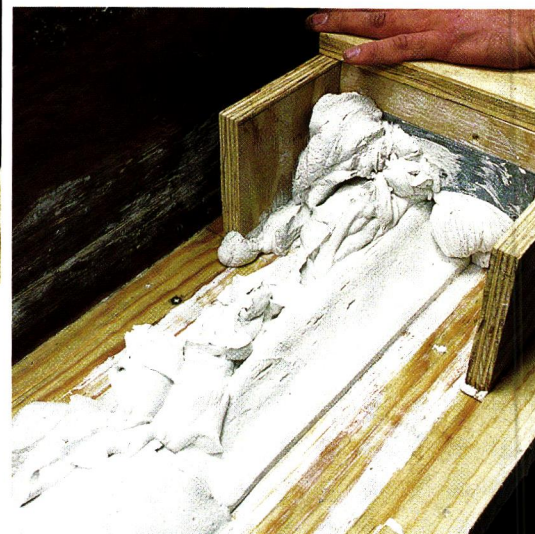
Below: Even after only one or two runs, the rude form of the moulding starts to take shape along the bottom parts of the profile. The higher features will be filled in before the next run with supplementary plaster—some of it from the mould.
