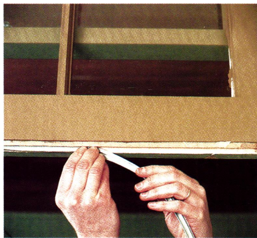
Rubber bulbs and seals are effective for sash window bottoms, but may require power tools to cut the kerf that holds the barbed flange.
