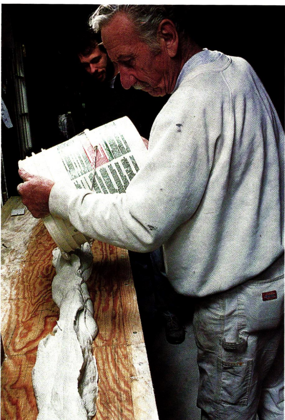
Left: As Frank lays the first batch of plaster, it pours out of the bucket at roughly the consistency of cake frosting. Above: Part of the skill of running the mould is keeping the two vertical slippers in constant contact with the bench and tight against the lattice (right in photo) while it pushes through the slippery plaster.
