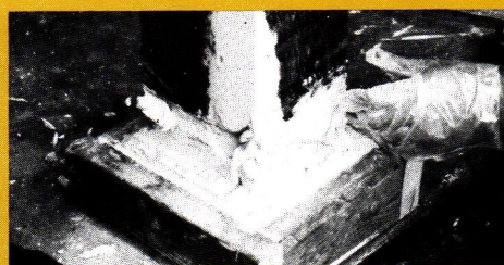
...were completely sawed off and replaced with...
