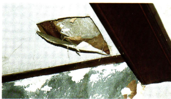
Through the tear in the fabric, you can see the original plaster inches above this balloon ceiling. The mouldings along the wall keep the canvas stretched like a drumskin.
