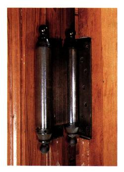
This original double-action hinge allows the door between the dining room and the kitchen to stand at attention in either room.
