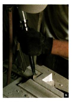
Above (left): After chipping away most of the material on the diagonal, Wright uses a curved chisel to carve the basic inverted S-shape of the moulding profile (2). Right: Using a toothed chisel, he cuts an L-shaped ledge above the profile (3).
