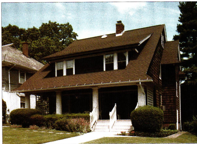
Top: The room behind the gable dormer may have started as attic space. Above: This relatively big house, with its shed dormer, would qualify as an über-bungalow.
