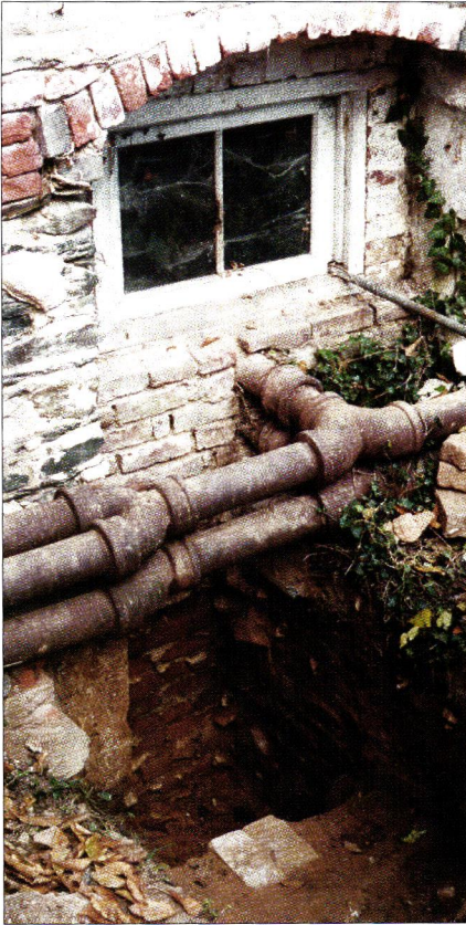
The original floor of the 1810 greenhouse at Oatlands Plantation is 3 1/2' below the current grade. Like many greenhouses of that time, it was heated via a captive brick flue, but theirs also warmed an unusual masonry heat bench, above right. The pipes, above left, are from a 1903 remodeling in which wooden roof supports with tiny panes were replaced with iron frames and larger sashes, and the heat came from a coal-fired hot water system. Below is the Oatlands greenhouse before its extensive restoration.
