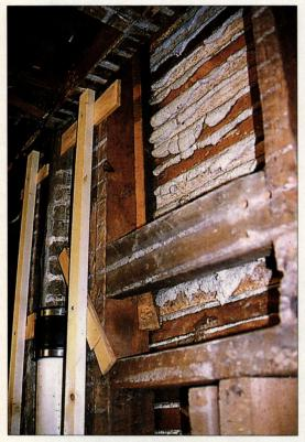
Here, furring strips ripped from 2x4 lumber are applied to studs to build them out enough for drywall to clear the piping. Shimming and nailing at strategic spots can be part of the process.
