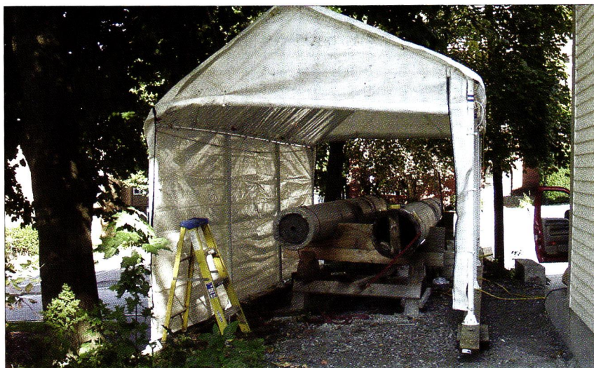
Sawing from the hole along the scribed line completed the cut. The scheme of 24" and 12" cuts was planned to take advantage of existing joints in the staves.
