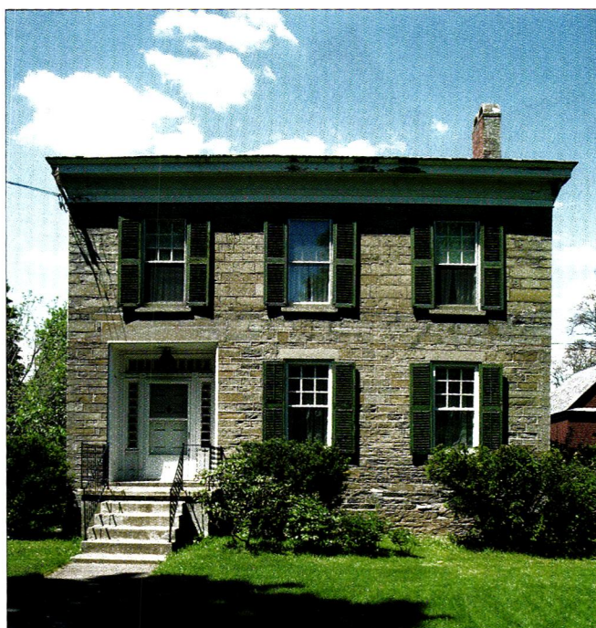
A plain, square, low-roofed stone Greek Revival in Unadilla, New York, has the entrance on the left side of the façade, usually indicating a side-hall plan within. Construction of the Erie Canal helped carry the Greek fashion westward to Ohio as well as provide skilled masons to build many stone examples along the way.
