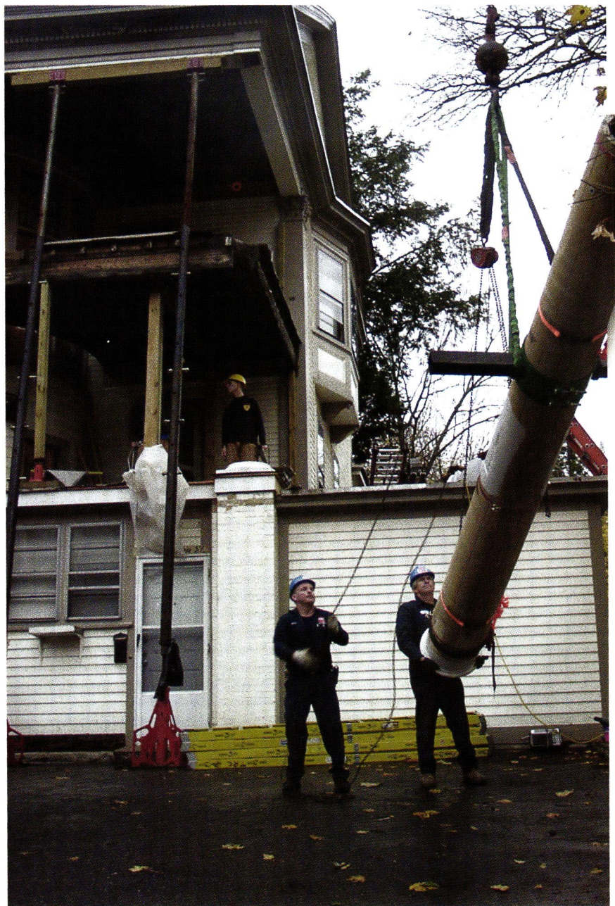
While a screw-jack system supported the porch, Toupin Rigging of Lowell, Massachusetts, re-installed the 18' columns using a crane and a custom-made collar, basically the reverse of the removal process.
