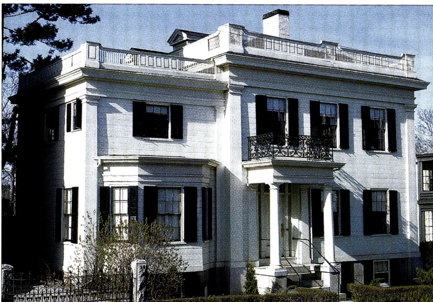
A portico isn't needed for elegance, as this example from Newport, Rhode Island, shows. The pilasters, cornice, and columned entry porch produce a fine house.
