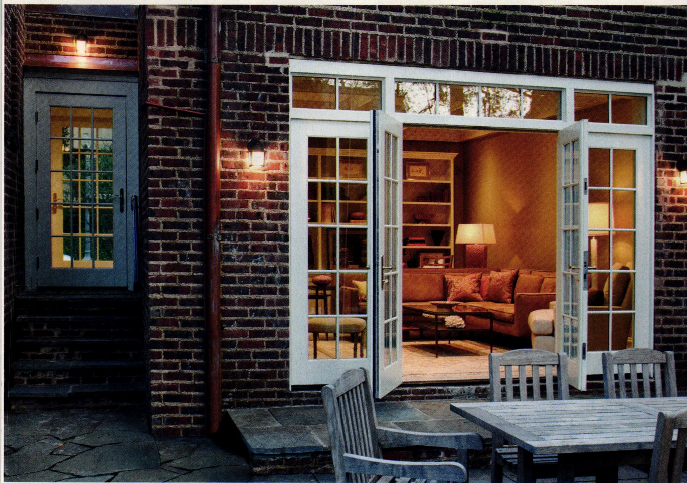
New French doors with sidelights and a transom afford an expansive view of the garden from the new family room—something that was distinctly lacking in the house's original configuration. Doors on either side of the breezeway provide access to the garden and the street.
