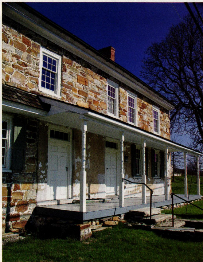
OPPOSITE: The 1725 John Chad House has traditional pent eaves between the stories. TOP: Recalling local building traditions, architect R. Brognard Okie remodeled this 19th-century house to expose the stone wall beneath stucco around the door and window. RIGHT: The Ashbridge House near Downingtown was built in three stages circa 1709, 1755, and 1810; the porch is a 19th-century addition.
