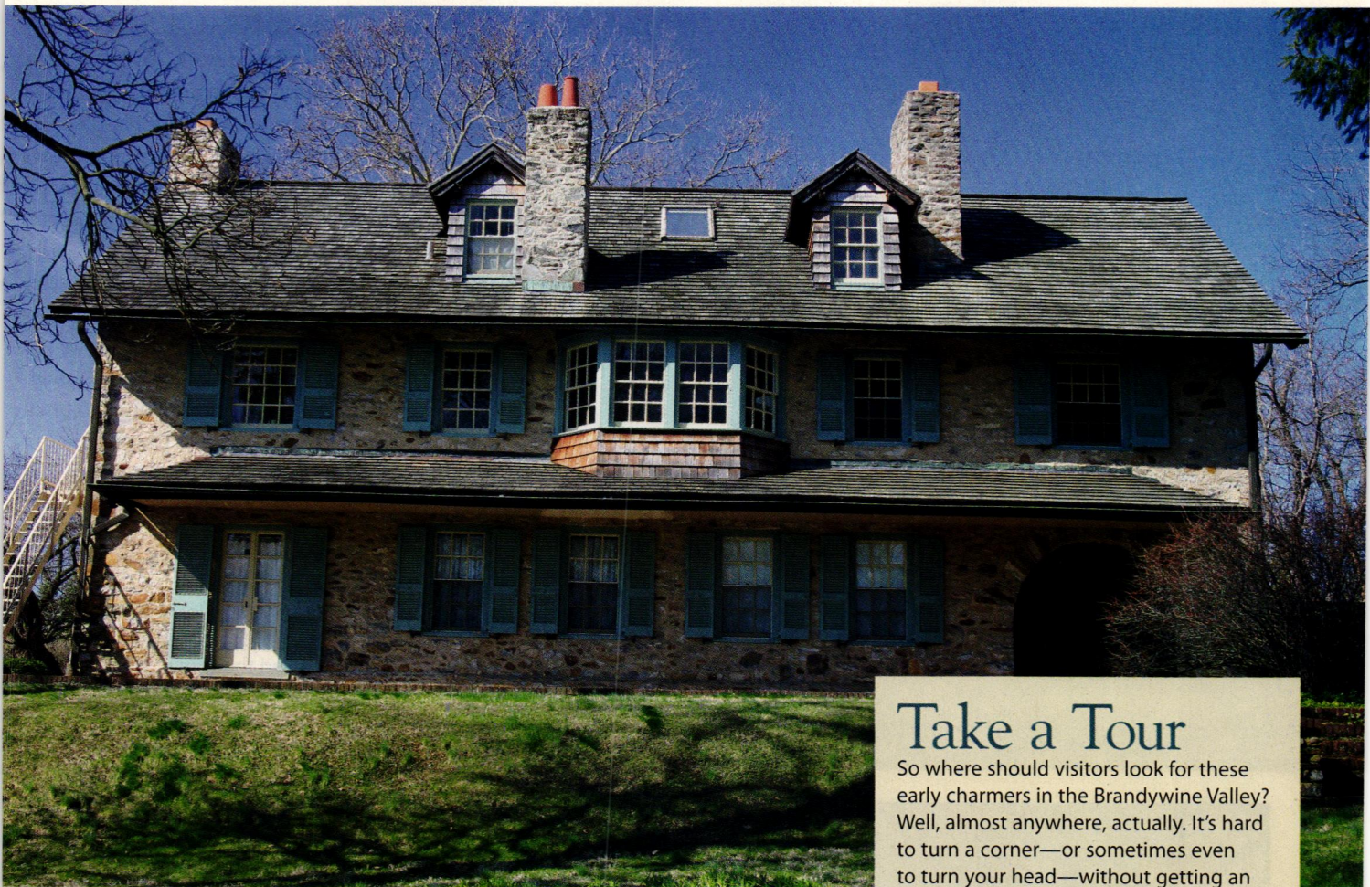
Bridging the centuries, the 1909 Breesy Court in Downingtown blends early 20th-century architectural features—such as the second-floor oriel window—with earlier building traditions, like the pent roof popular during the 18th century.
