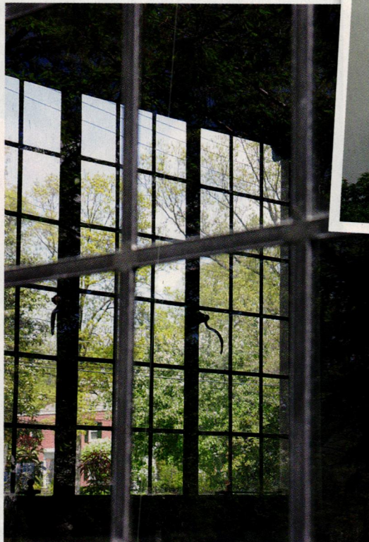
ABOVE: The "before" view of the house shows a mixup of modern replacement windows with no divided lights. LEFT: The newly installed steel casements provide a vintage view both into, and out of, the house.
