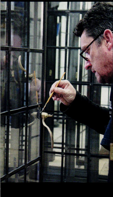
LEFT: Windows are painted by hand using Benjamin Moore's Bronzestone, a shade complementary to many old houses. Here, Ralph Whitehead fills in paint around the handle. ABOVE: The finished windows are loaded into a truck, ready for delivery.
