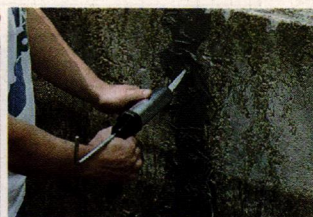
Abojet bonds structural walls.
