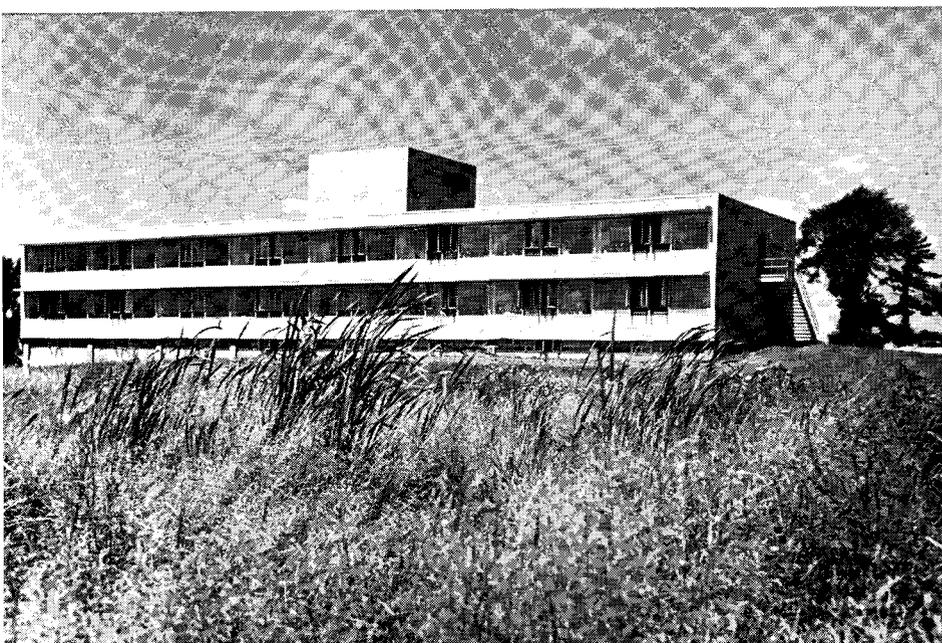
The main entrance to the hospital (above) faces due north. Most patients' rooms are lighted by continuous window strips along the south side of the building (left and across-page). Unusual is the plan scheme of delivery room and operating room on separate floors, immediately adjacent to the pertinent nursing units. Notice that there is no laundry in the building, as laundry for all three hospitals is handled at the central unit in Gouverneur.
