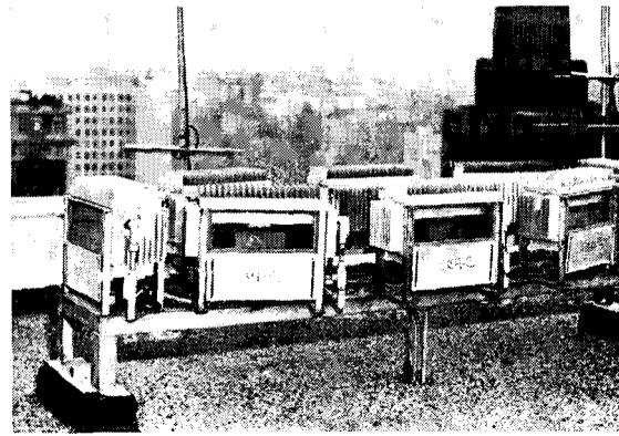
Eight electrical "watchdogs" installed on the roof of the new Los Angeles Statler Center hotel and office building automatically vary the cooling capacities of the building's air-conditioning system according to changes in the angle and intensity of the sun's rays. Each unit of the solar compensator faces a direction corresponding to one of the major exposures of the building's wings. Carrier Corp., Syracuse, N. Y.
