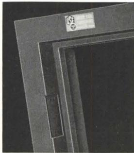
All hinge and strike reinforcements are mortised, drilled and tapped on both doors and frames.
