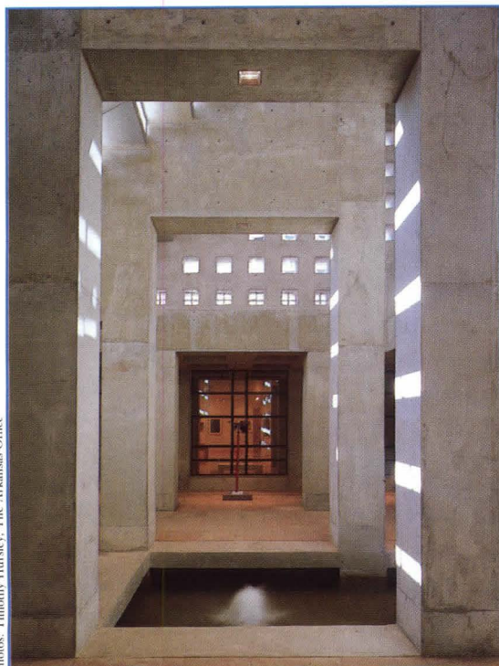
Twelve-inch glass block grid from the interior.
