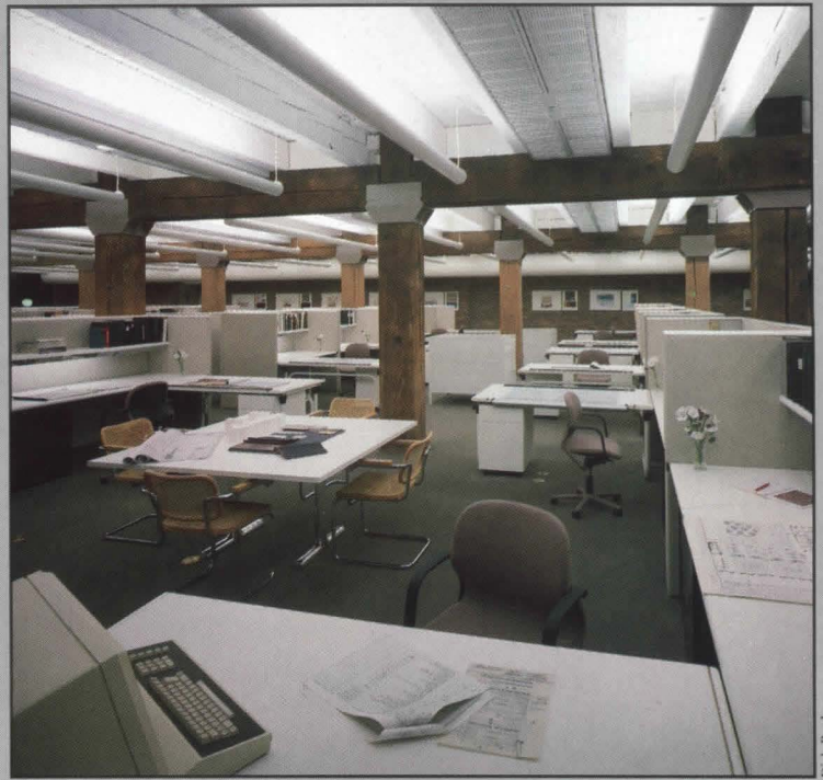
Post caps on the columns are load-bearing and absorb shaking forces.
