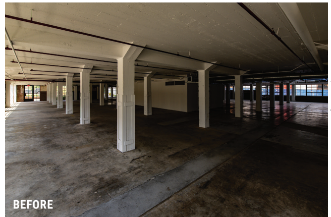
BEFORE PHOTO: Cooper Carry
