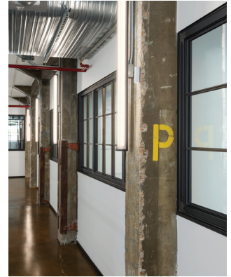
Historic features were preserved as subtle tributes to the building's past.
