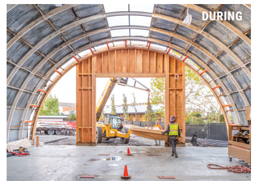
BEFORE, DURING PHOTOS: courtesy Skylab Architecture
