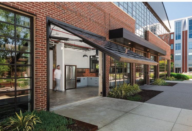
Full-sized windows maximize natural light, which reduces the need for overhead lighting and boosts worker morale. Garage doors open to the outside, bringing in fresh air and sunlight.
