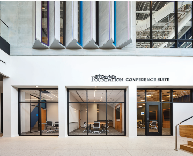
A community room that can be used for classes and meetings is available for rent, and technology used throughout the public spaces communicates the facility's role in fostering dialogue.
