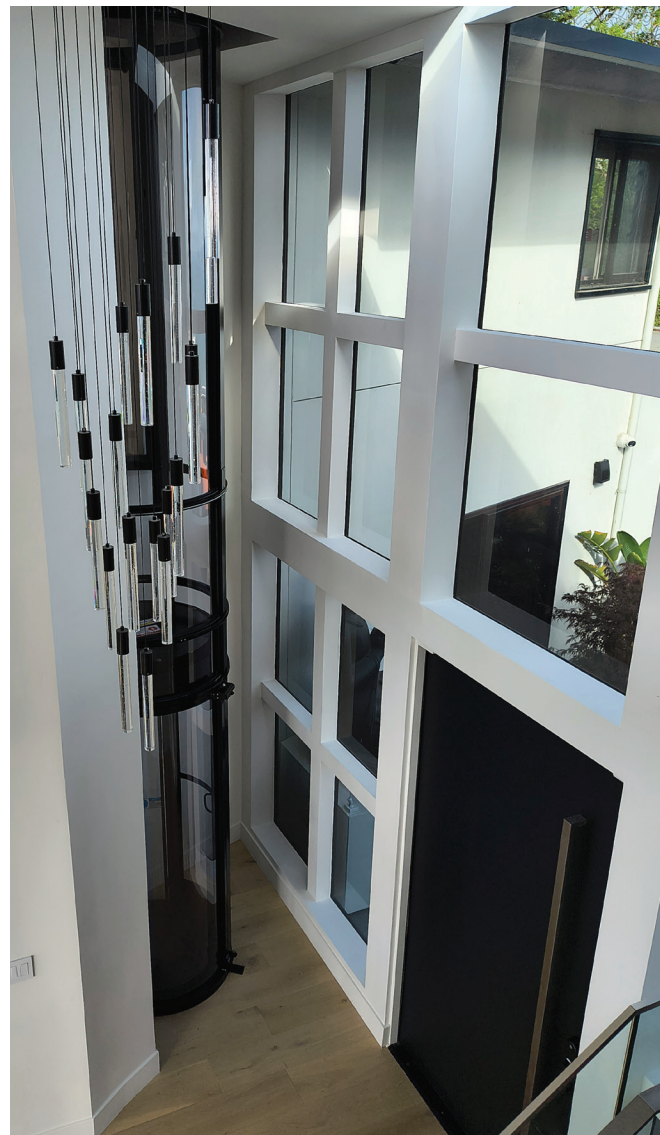
In the entry, in preparation for aging-in-place, a pneumatic vacuum elevator was installed to connect the upper and lower floors.
