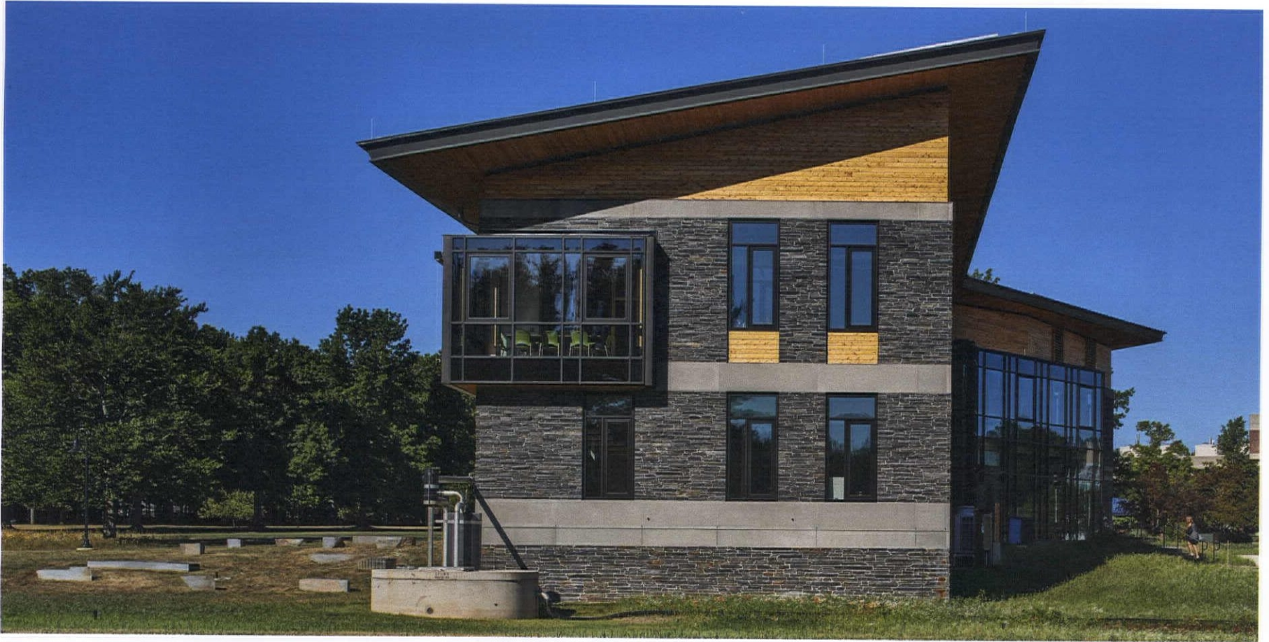
FULL CYCLE Rain collected by the Kern Center's roof (above) is stored in concrete cisterns. All site water is treated and reabsorbed into the landscape through rain gardens or a graywater treatment system (right).
