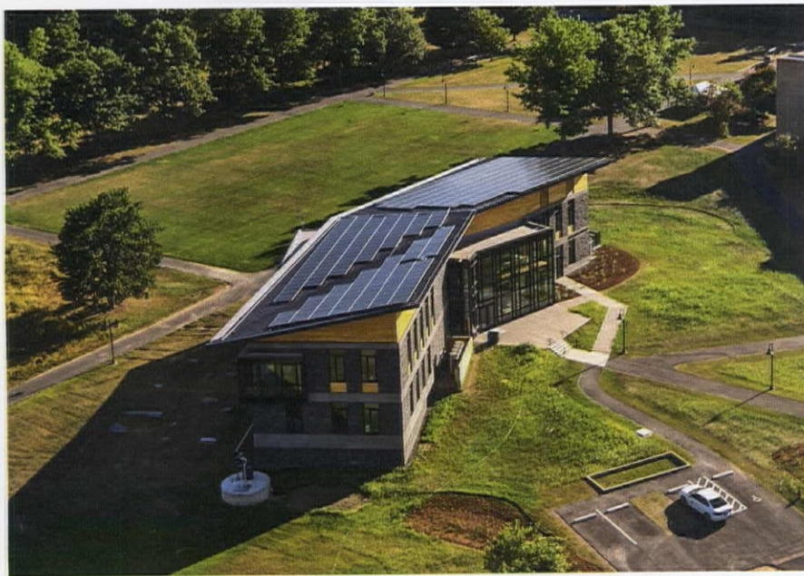
FINE-TUNED For the R.W. Kern Center at Hampshire College in Amherst, Massachusetts (from top), Bruner/Cott and Berkshire Design closely studied the roof and gutter details to optimize the performance of the rainwater-harvesting system.
