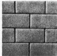
Brick running bond ungrouted
