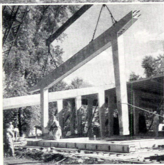
Large photo shows one wing of the Linton-Stockton School. Small photo above shows a close-up view of one of the precast concrete bents while photo below shows method of stockpiling concrete bents before erection. Designed by Thomas C. Dorste and Spiros G. Pantazi of Indianapolis. Structural engineer was Floyd E. Burroughs, also of Indianapolis.
