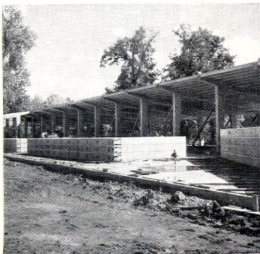
Large photo shows one wing of the Linton-Stockton School. Small photo above shows a close-up view of one of the precast concrete bents while photo below shows method of stockpiling concrete bents before erection. Designed by Thomas C. Dorste and Spiros G. Pantazi of Indianapolis. Structural engineer was Floyd E. Burroughs, also of Indianapolis.
