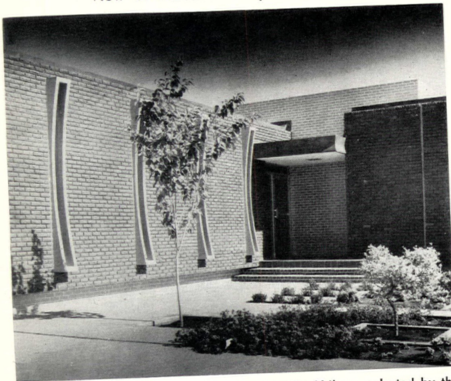
An exterior view of The Barber Building in Abilene, selected by the new Abilene Chapter, AIA as representative of recent architectural work in the area. Shown are vertical glass slits in the brick walls, enclosed with curved porcelain enamel frames. The blue porcelain frames glow at night, reflecting interior light. Architects: Tittle & Luther, TSA-AIA, of Abilene.
