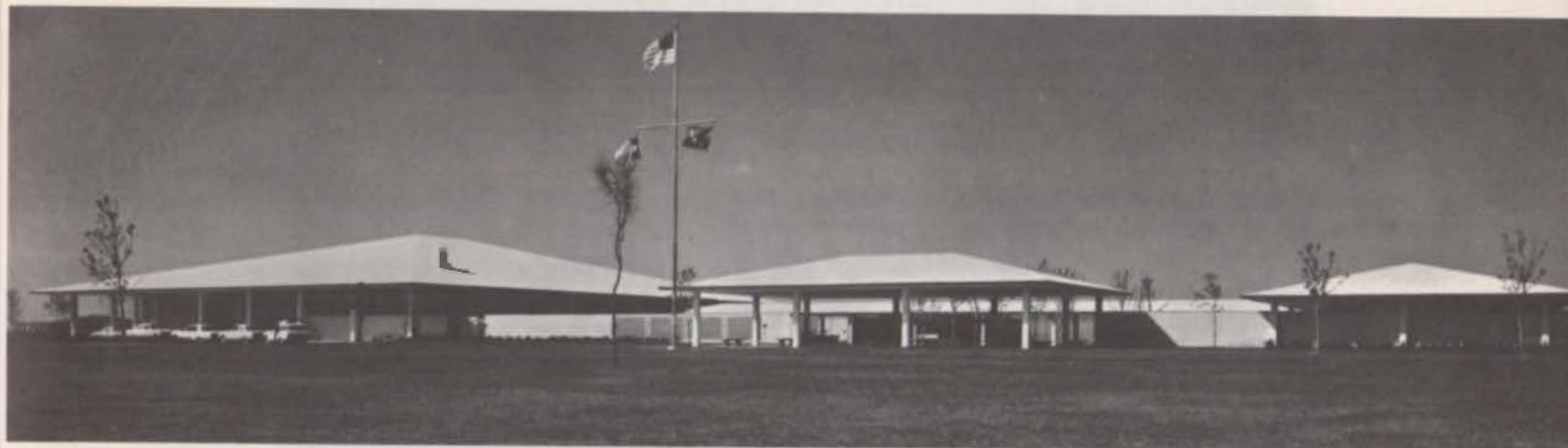
Seen from the main drive adjacent to the Center, the four basic elements of the program are apparent in the roofs: the large hip of the auditorium, the small roof of the activities building on the right, the playshed-entry pavilion representing outdoor activities, and the long, low roof defining the pool area beyond.
