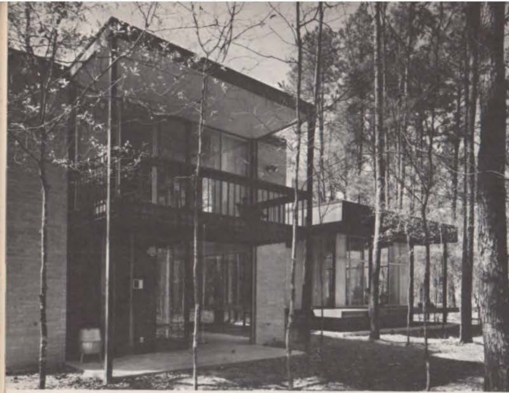
The steel frame of the cubes repeat the verticals of the trees and blend with the nature-forms of the site.
