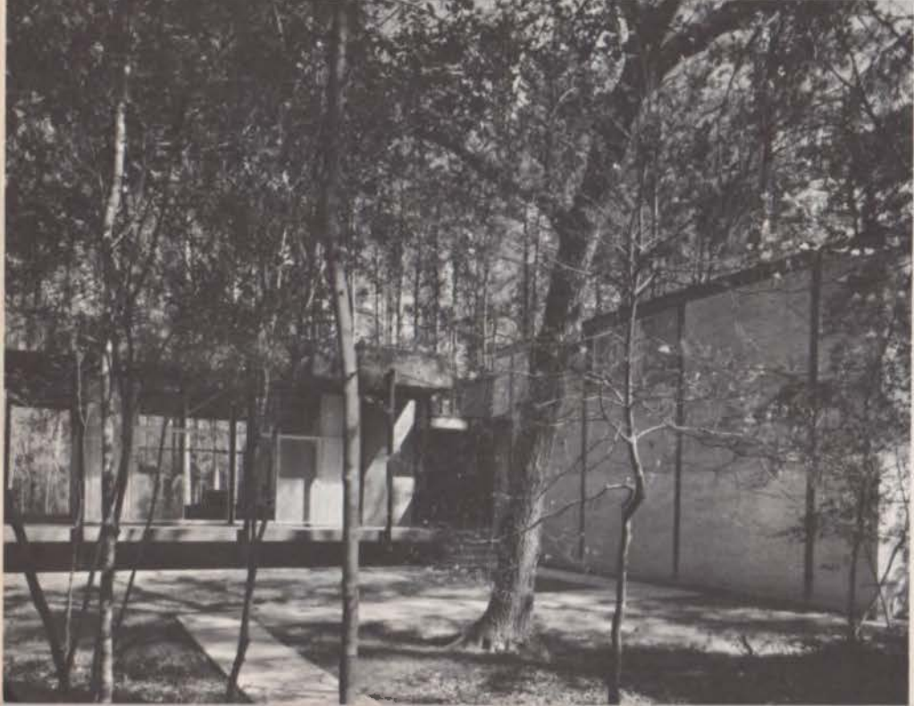
The entry walk twists angularly through the densely wooded site and approaches in a way to show the building blocks in different aspects.
