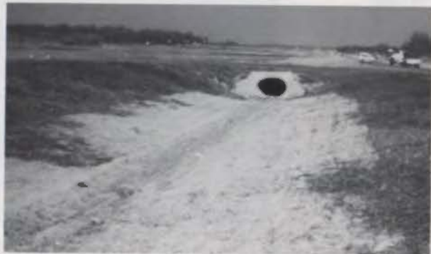
Top Photo: Curlex Blankets protect this ditch on Highway 121 in North Texas. The photo was taken in the fall of 1982.
