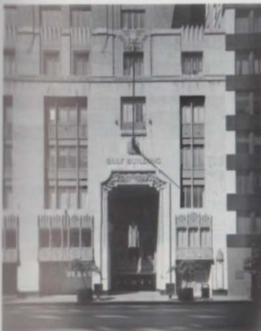
Stone, metal, and terra-cotta details articulate the base of Finn's Gulf Building.
