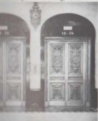
Niels Esperson Building, lobby detail
