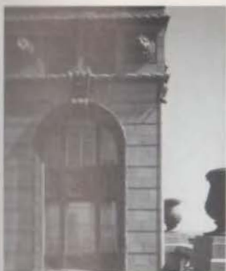
Niels Esperson Building, detail
