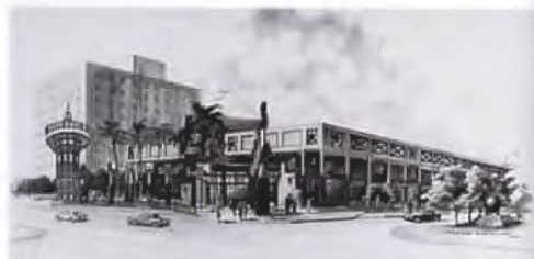
The Albert Thomas Convention Center, vacant since 1988, is being redeveloped into
