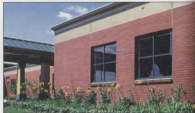
Bowen Elementary School Bryan, Texas Patterson * Architects, Bryan
