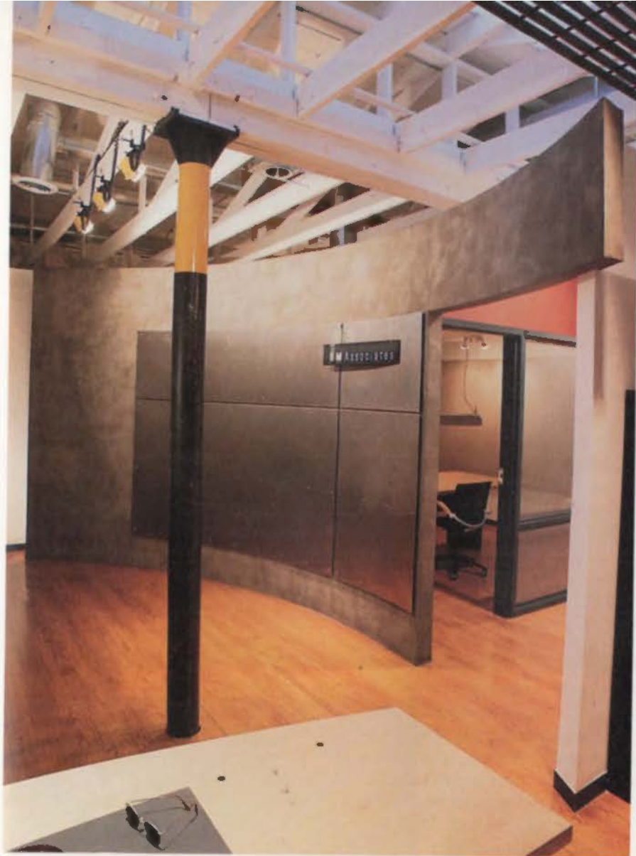
3 A curved wall of steel plates serves as a divider between the reception desk and a conference room; the plates are bolted to a wood stud wall coated in hand-troweled mortar.
