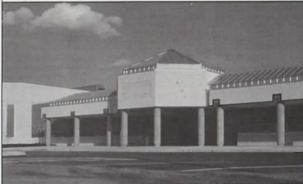
SATIN FINISH GALVALUME BERRIDGE TEE-PANEL STANDING SEAM ROOF PANELS HIGHLIGHT THE ENTRY OF CEDAR PARK MIDDLE SCHOOL. PANELS WERE SITE-FORMED WITH A BERRIDGE PORTABLE ROLL FORMER.
