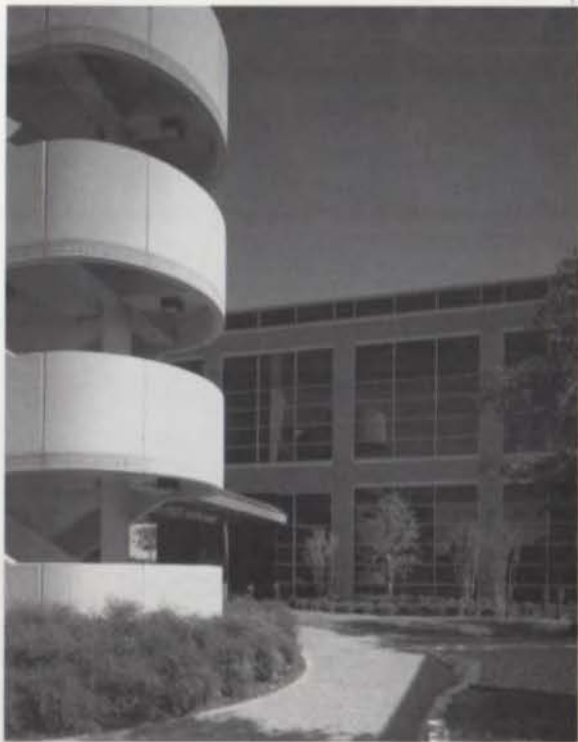
2 Ventilation systems required for baking and etching processes provide a defining image.
