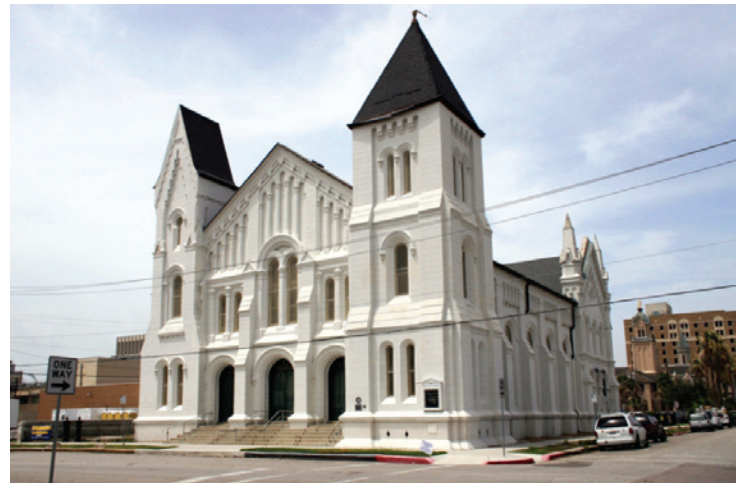
First Presbyterian Church, 1903 Church Street
