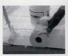
PRESERVATION PRODUCTS' "Acry-Max," a weatherproofing system for roofing and masonry, combines multiple layers of acrylic coatings with a high-strength fabric for additional durability. Write in No. 8180
