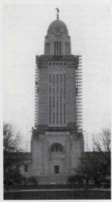
U.S. HERITAGE GROUP created replacement mortar for the restoration of the Nebraska State Capitol, using lime putty and sand from the nearby Platte River, as was used in the original construction. Write in No. 852
