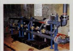
The water-filtration systems offered by DIAMOND WATER SYSTEMS are used primarily to remove heavy loads of suspended solids in recirculating fountain water. Write in No. 2350
