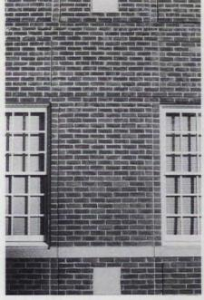
The waterstruck-brick method used by VERMONT BRICK MFG. involves water and sand in the molding process, resulting in a uniquely textured brick suitable for renovation and restoration, as well as new construction with a traditional look. Write in No. 765
