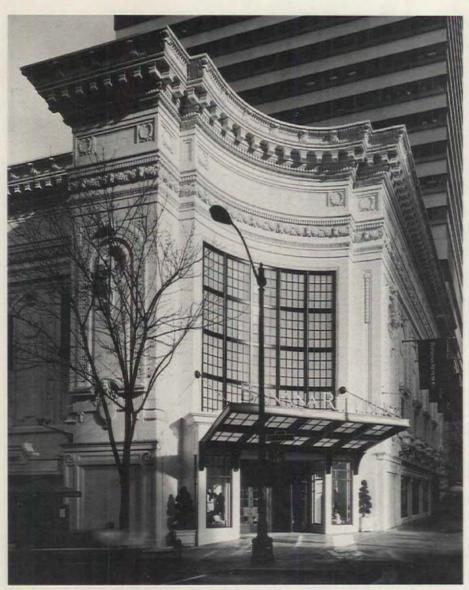
The terra-cotta replacements for Seattle's Coliseum Theater renovation included AR-CHITECTURAL REPRODUCTIONS' individual precast-concrete units and larger moldings in multiple block assemblies, using glassfiber-reinforced thinshell techniques. Write in No. 6130
