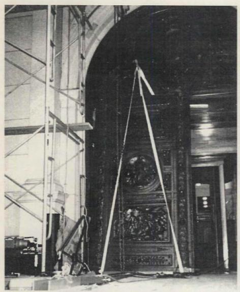
F.E. CICCONE & CO. specializes in monumental doors and entries, and restored and reengineered bronze doors at the Pennsylvania State Capitol Building. Here is one step in the process of hydraulically moving the door out of the building. Write in No. 525
