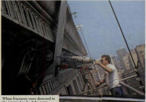
When fractures were detected in the internal web of the terracotta units, the elements were stabilized with the installation of stainless-steel anchors: rods, plates, and angles. This required drilling holes into the face of the terra cotta with a custom-designed set-up capable of drilling several feet into the structure — while workers were standing on special cantilevered scaffolding suspended from the roof.
