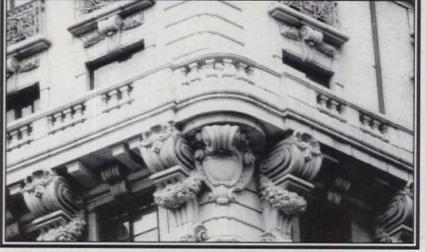
1,500 units of cast stone and GFRC were fabricated to restore the terra-cotta balcony and consoles of the landmark Ansonia Hotel, New York, NY.
