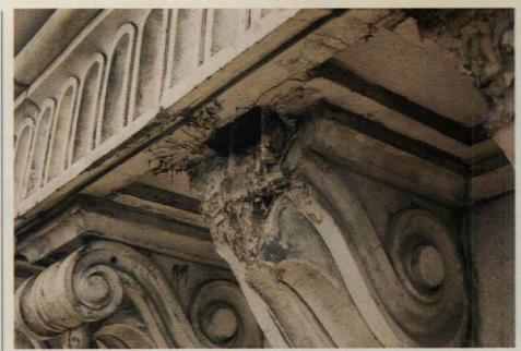
The major problems with the cornice were caused by water penetration, mainly through the roof deck. The water caused some of the steel fixings to rust; pressure from the expanding iron oxide fractured and pushed off portions of the terra-cotta units.
