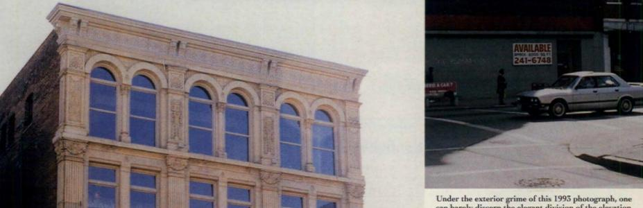
Under the exterior grime of this 1993 photograph, one can barely discern the elegant division of the elevation into three vertical bays by a series of articulated pilasters. One can only imagine what classical motifs might have once graced the street-level facade, now lost forever.
