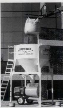
With each ingredient custom-mixed and weighed by factory computers, the use of Spec-Mix from PACKAGE PAVE-MENT eliminates the inconsistencies associated with some field-proportioned mortars. The company can also analyze the components of a historic mortar, and then provide a pre-packaged mix that will replicate the look and performance of the historic material. Write in No. 3121
