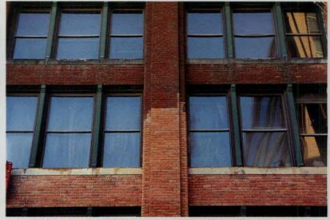
Grimy brick (upper section of photo) on the Boydel Building in downtown Detroit is being cleaned to its original light hue (lower section in photo) by soft abrasive cleaning with Armex, an environmentally safe cleaner based on baking soda.
