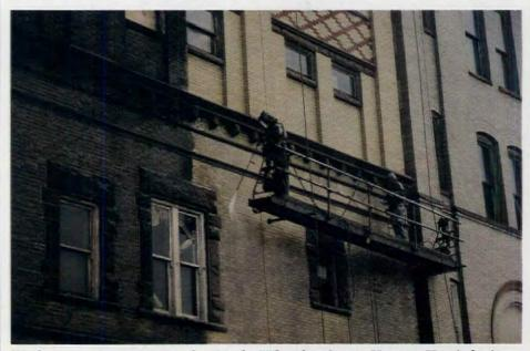
Workers on swing staging are cleaning the Milwaukee County Veterans Hospital using a diluted acidic brick cleaner, 101 Masonry Restorer from Diedrich Technologies. The hospital was originally built to serve Civil War veterans — and is still in use as a veterans' residence facility.
