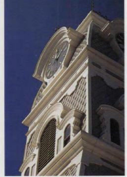
The original bell tower of Hill County Courthouse and its elaborate roof were destroyed in a New Years Day1993 fire. Both were reconstructed in their original material — pressed sheet metal — using stock elements from W.F. Norman and Berridge along with custom fabrication based on pieces salvaged from fire debris. (All Photos: Gary Skotnicki unless noted)
