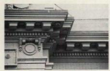
These ARCHITECTURAL FIBER-GLASS CORP. dentils and corbel brackets are integrally molded into this cornice on the Yonkers City Hall in New York. The integral color molded into the cornice matches the existing terra cotta on the building. Write in No. 6400
