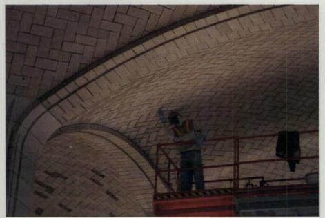
Good scaffolding was an intrinsic part of Graciano's job. In areas that required extensive tile replacement, wooden molds were created to apply the pressure needed to keep the remnant tile in place and intact. (All photos courtesy Graciano Corp.)
