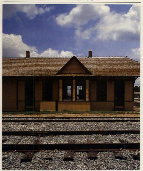
Restoring the Cotton Belt depot, c. 1890, required a little cut and paste. Surviving portions of the depot were identified in two different locations. ARCHITEXAS provided the preservation and architectural services needed to move them back to their original site, restore the "missing link," and reconstruct new elements. In addition to functioning as a station for daily steam-train service, the depot currently houses a museum and visitors center.
