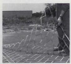
ARTCRETE, INC., creates durable faux brick paving from stencil-finished con-crete in a wide variety of styles, colors, and patterns. Write in No. 2140
