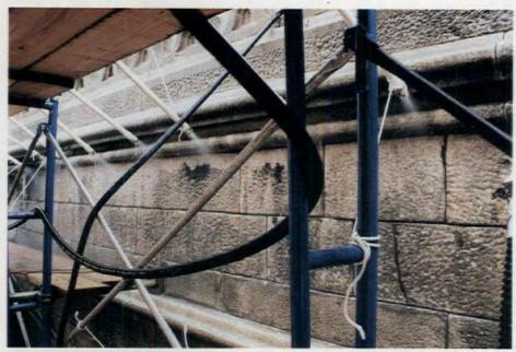
After extensive testing, preservation technologists at Wiss, Janney, Elstner decided to clean the Marble Collegiate Church, New York City, with a two-step water-washing process: (1) A 12-hour water soak, followed by (2) rinsing with low-pressure 500- to 600-psi wash water. In the photo, water is being applied through a multi-nozzle manifold. *Photo: Diane S. Kaese*
