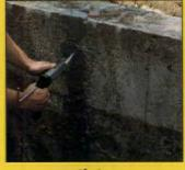
AboJet series for structural crack-injection
