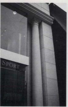
BALL CONSULTING takes advantage of new technology using GFRC thinshell composite systems to replicate architectural terra cotta and simulate a wide range of terra-cotta finishes and glazes. Write in No. 7260
