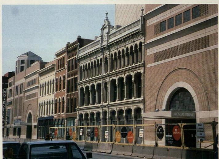
Everything new is old again at Circle Centre Mall in Indianapolis, which features components from demolished landmarks. Robinson Iron used the facades and ornamental details of two sister buildings to create a single shell for the mall's Vajen Building.
