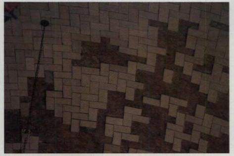
Over 28,000 tiles needed to be replaced, having been irreparably damaged either by water or from the vibration of traffic on the bridge above. In one area the ceiling was permanently lowered to prevent further harm.
