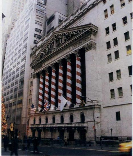
As part of its 3-year exterior restoration program at the New York Stock Exchange, Nicholson & Galloway cleaned, patched, and repointed all 115,000 sq.ft. of exterior Georgia marble. For the marble cleaning phase, the contractor used a combination of water washing plus selective soft abrasive and chemical cleaning. The newly cleaned Exchange building is shown here decked out in its Christmas decorations.
