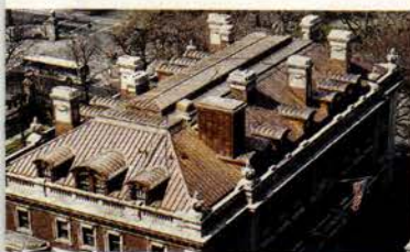
Duplicated the original copper design to complete the restoration of the roof of the Regie Mansion in New York City.
