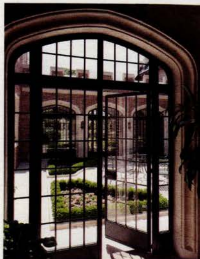
Crittall Windows offers traditionally styled windows and doors made with recycled and recyclable-steel content.
