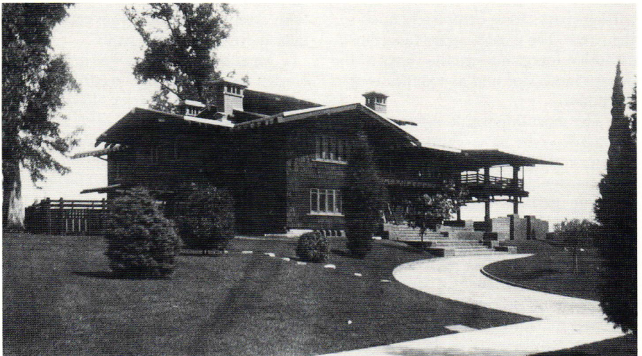
The David Gamble house in Pasadena (1908) is one of the best examples of the Greens’ use of Japanese themes. The house is lifted up on a terrace that surrounds the bulk of the house and extends the space of the living rooms out toward the garden. Documents Collection, University of California, Berkeley.
