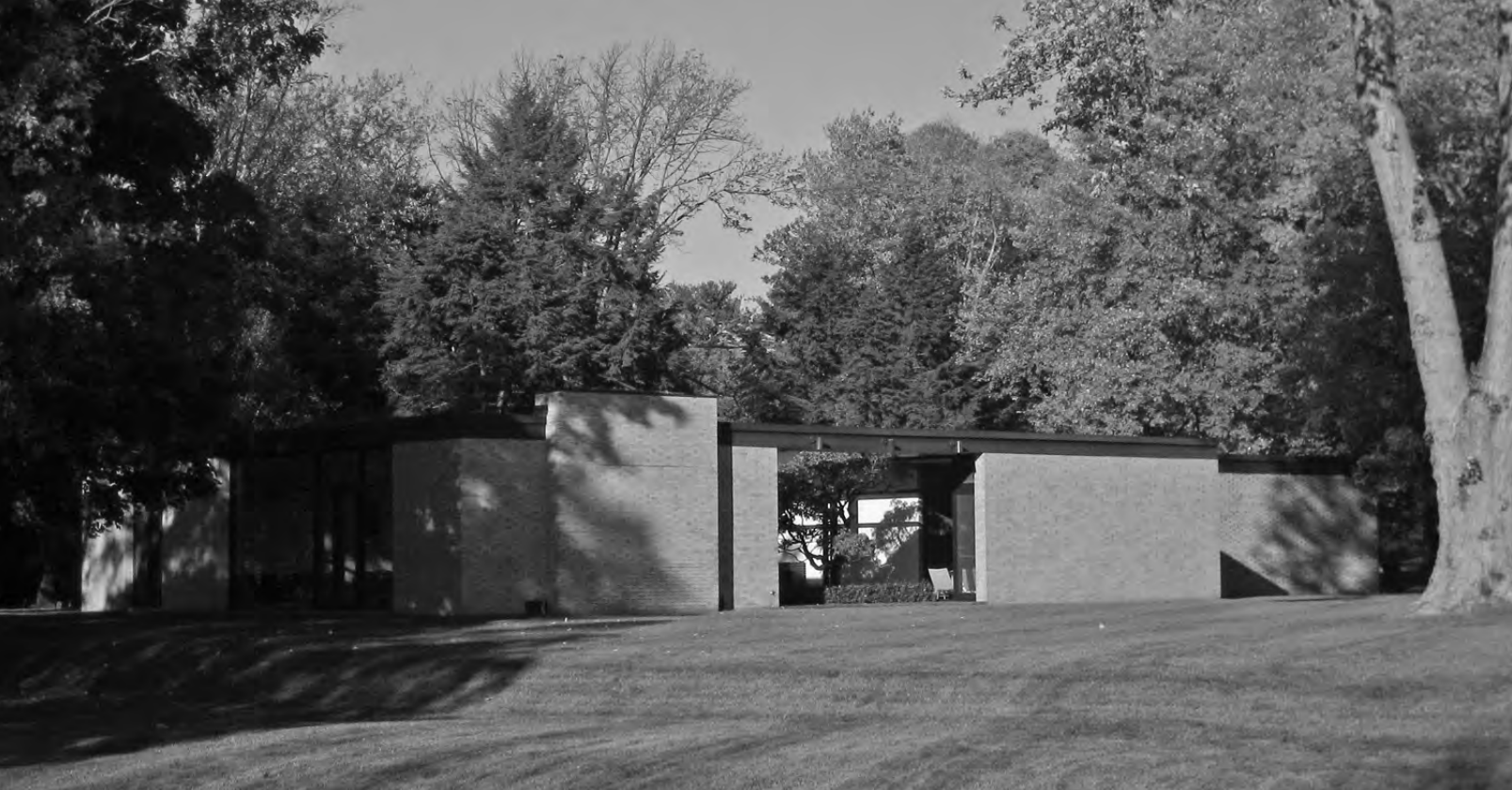
Hodgson House, rear and side façades, October 2007 (photographer: Eileen Brackenbury)
