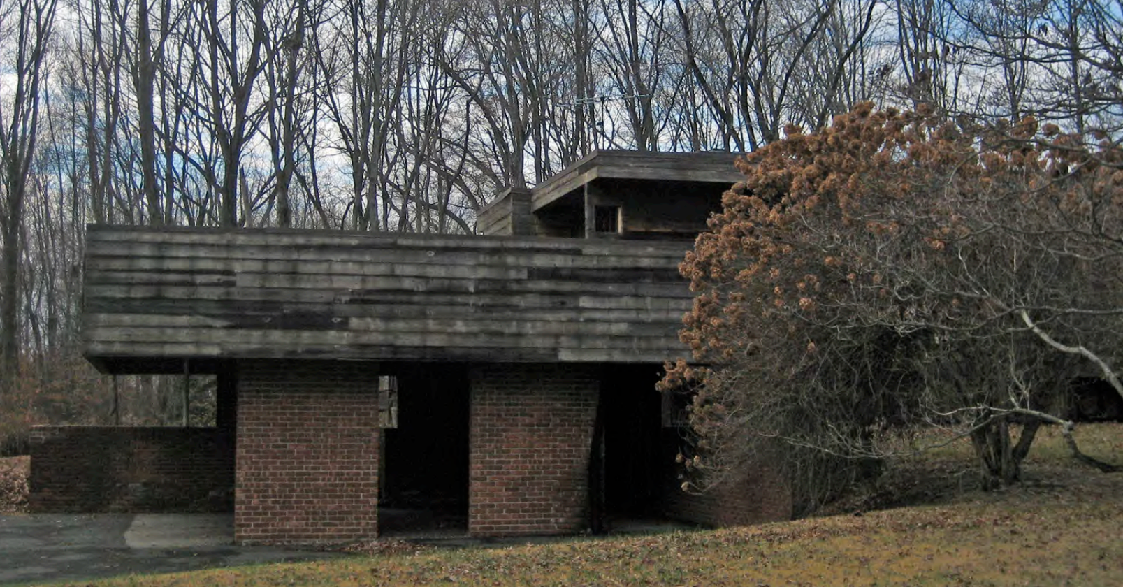
Waxberg House, carport and primary façade, December 2007 (photographer: Heather McGrath)
