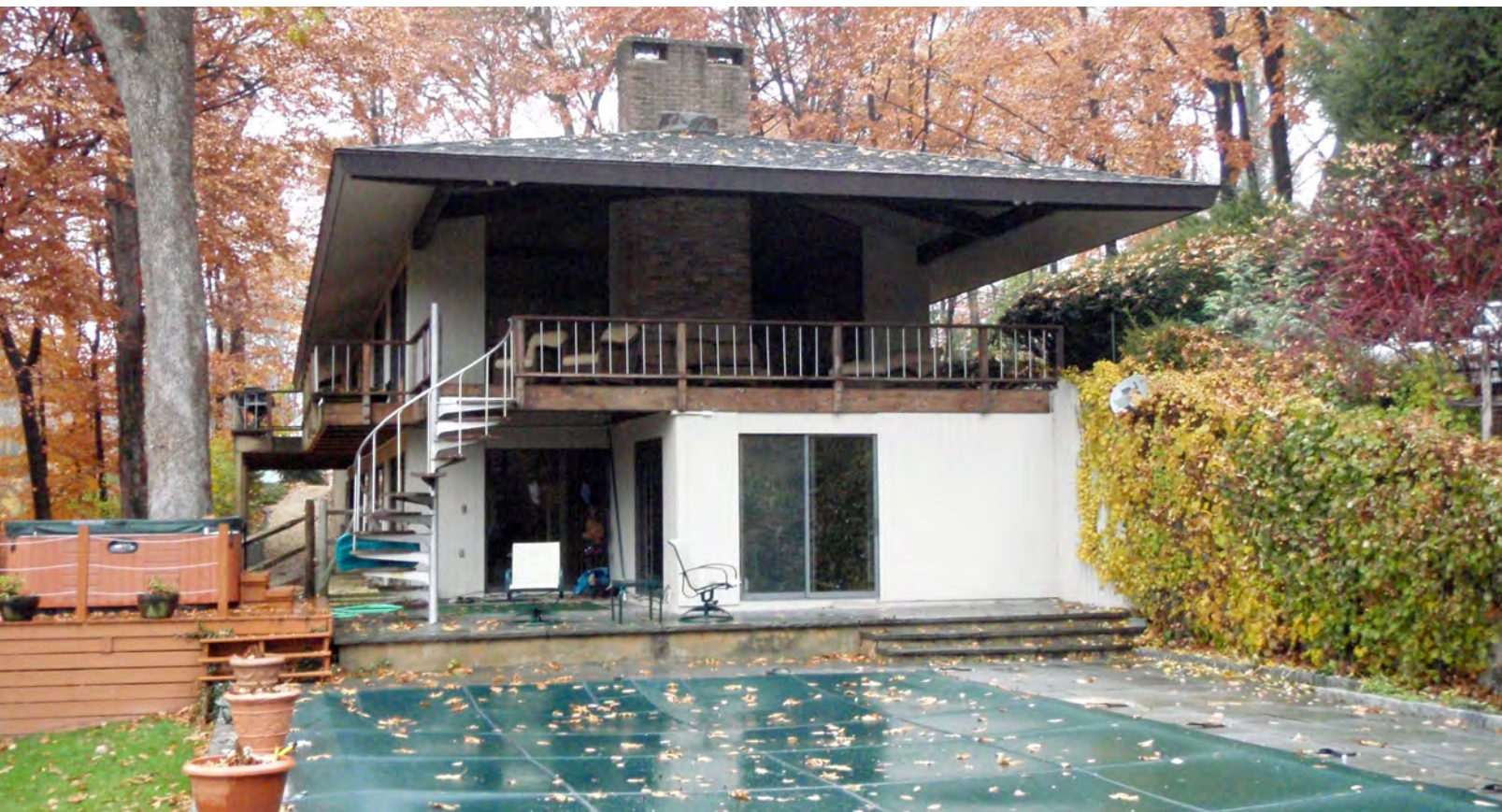
Monroe House, side façade and swimming pool, November 2007 (photographer: Martin Skrelunas)
