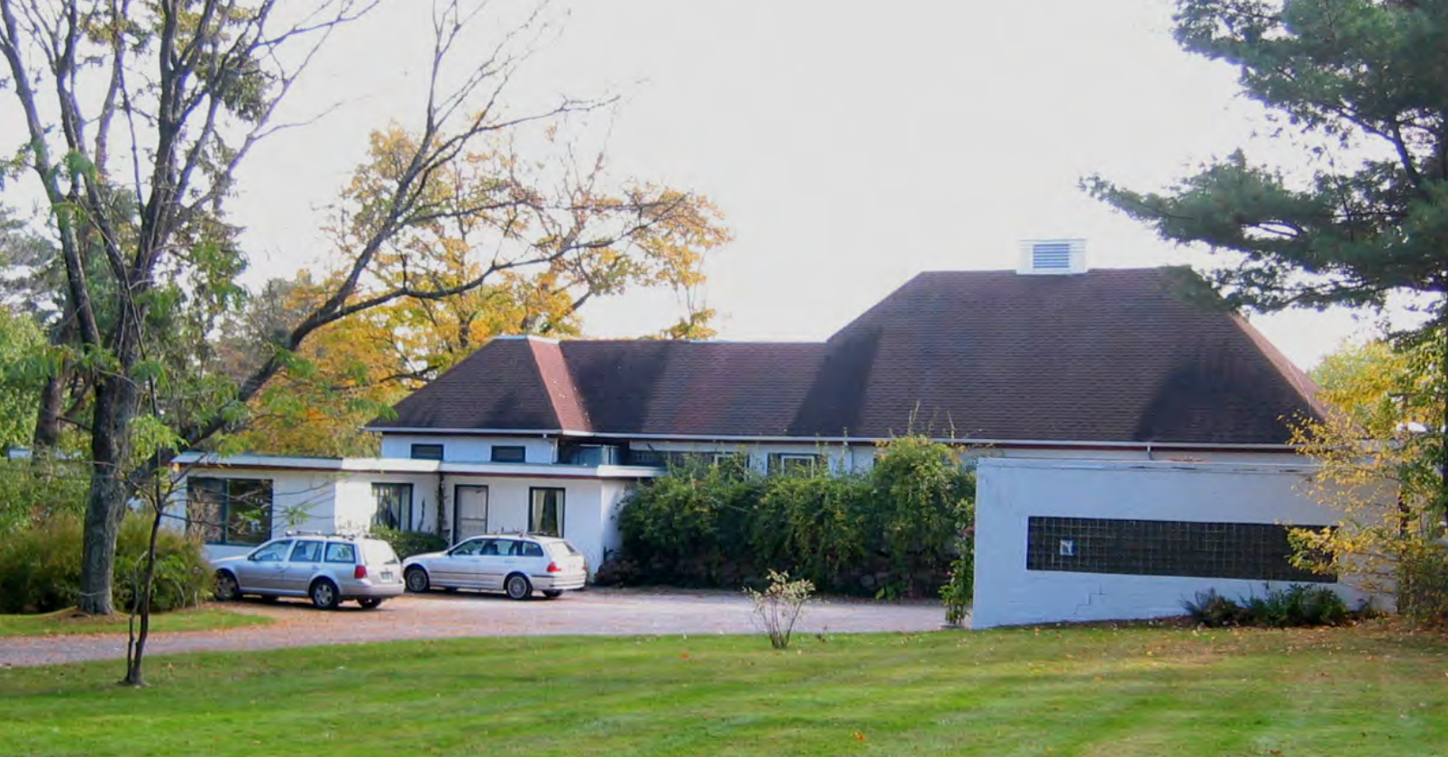
Goldmark House/Salant House, front façade, November 2007 (photographer: Eileen Brackenbury)
