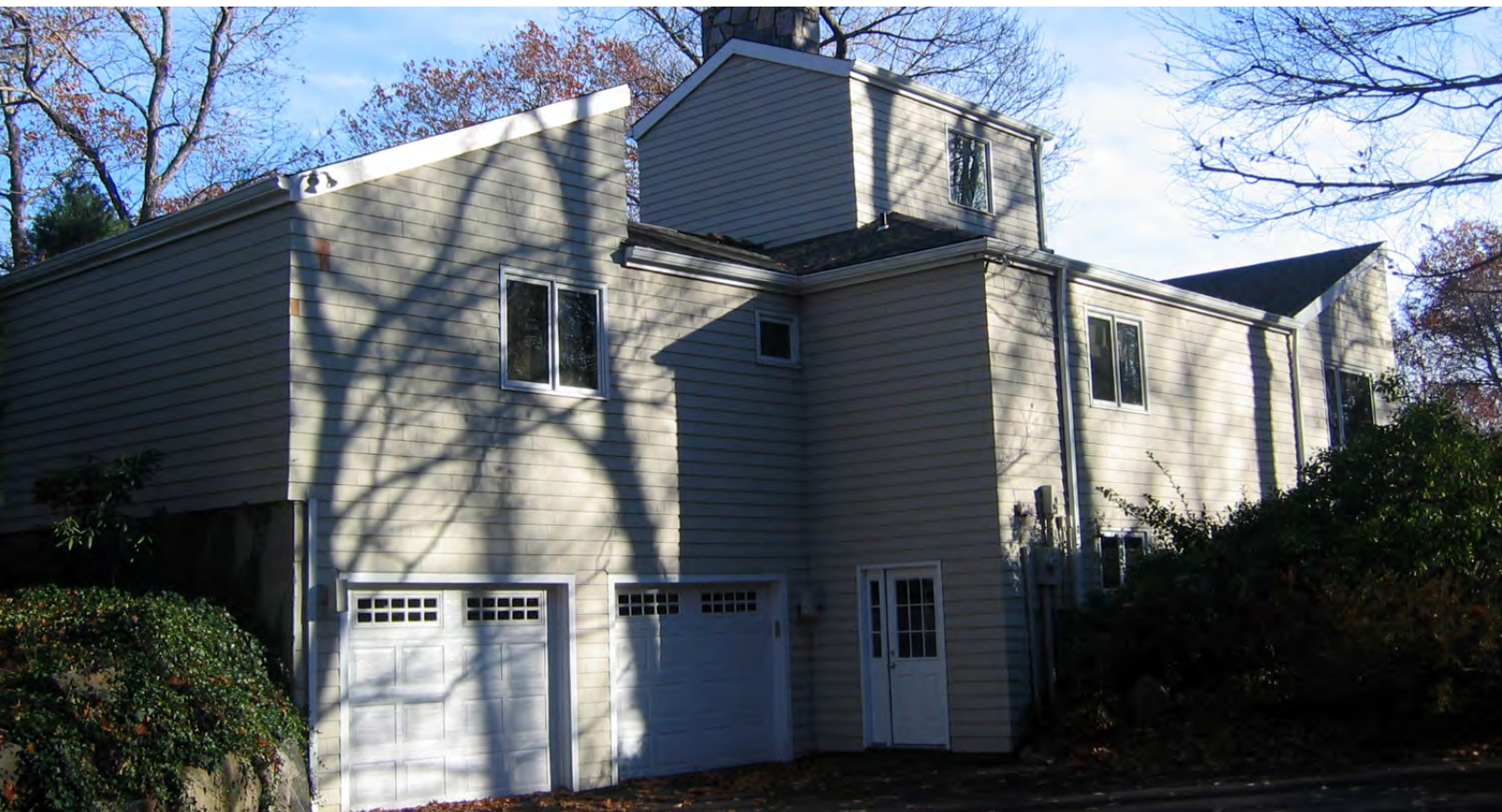
Branch House, rear (west) façade, November 2007 (photographer: Eileen Brackenbury)
