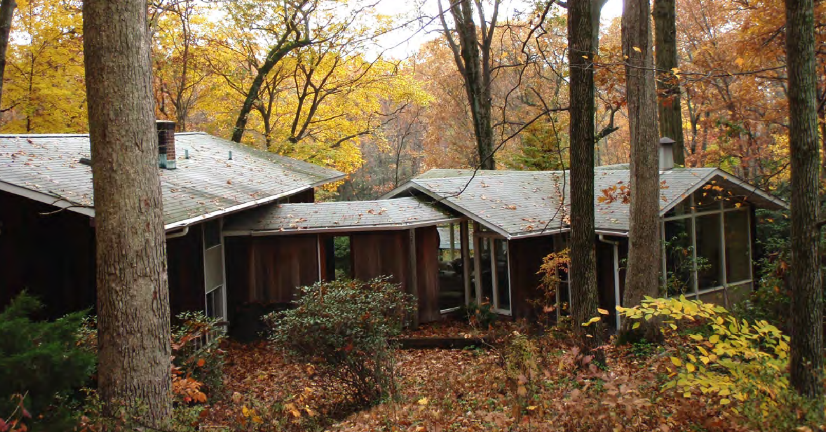
Techbuilt House/Swallen House, rear façade and addition, November 2007 (photographer: Martin Skrelunas)
