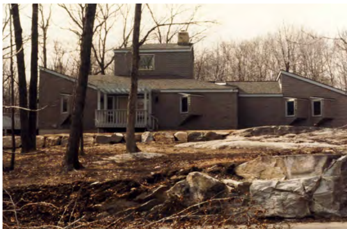
Figure 13. Branch House (1979-80, Christ-Janer), ca. 1981 (photographer: Branch family, source: New Canaan Historical Society). Victor Christ-Janer used solar principles in the Branch House for energy efficiency. The angled bay windows were designed to bring light and heat from the south while blocking cold from the north. The bay windows have now been removed.
