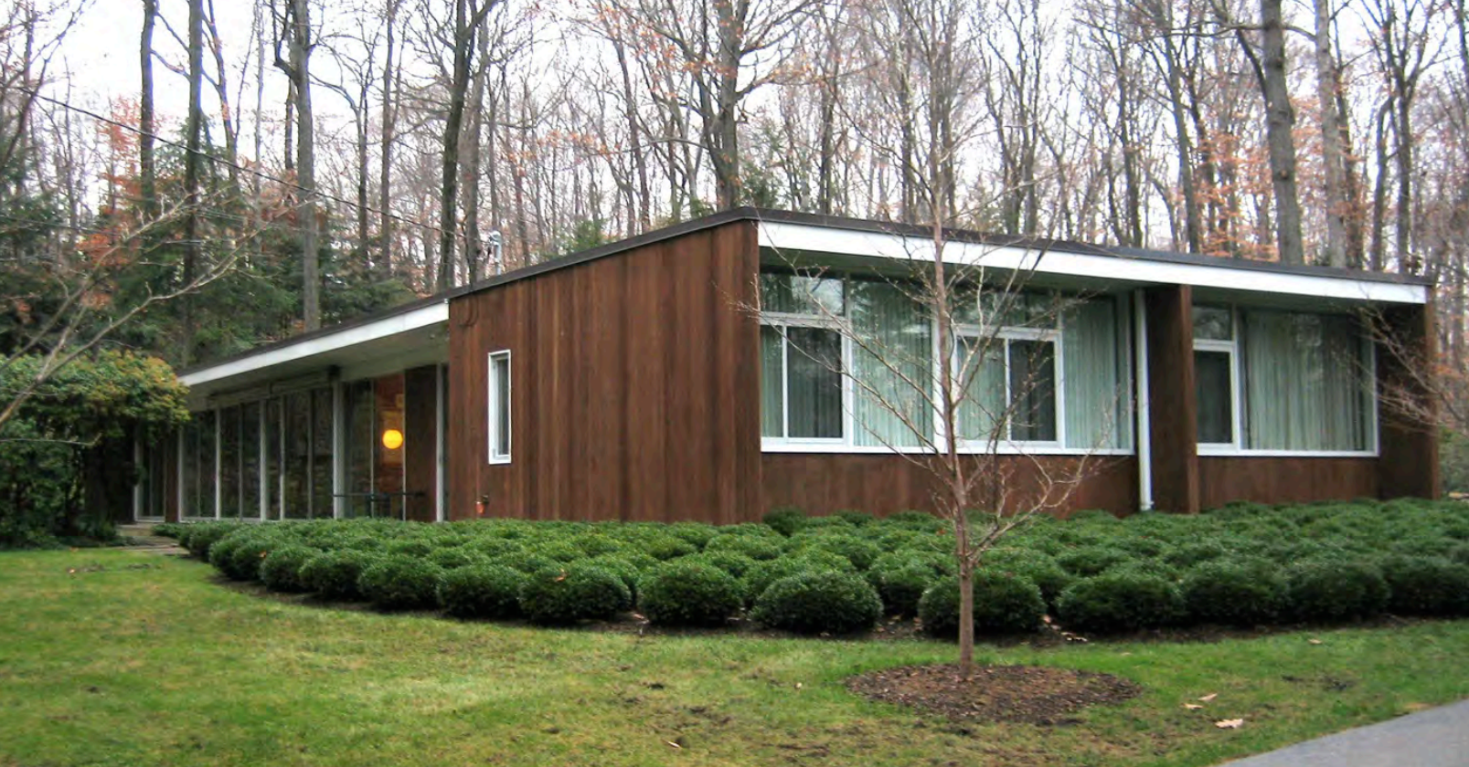
Crichton House, side and rear façades, December 2007 (photographer: Heather McGrath)
