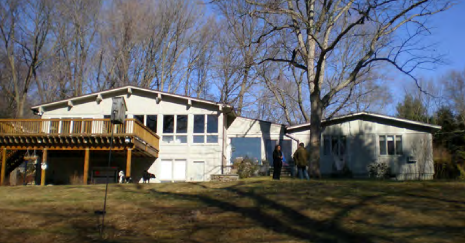
Zucker House, rear façade, February 2008 (photographer: Allyson Mehley)
