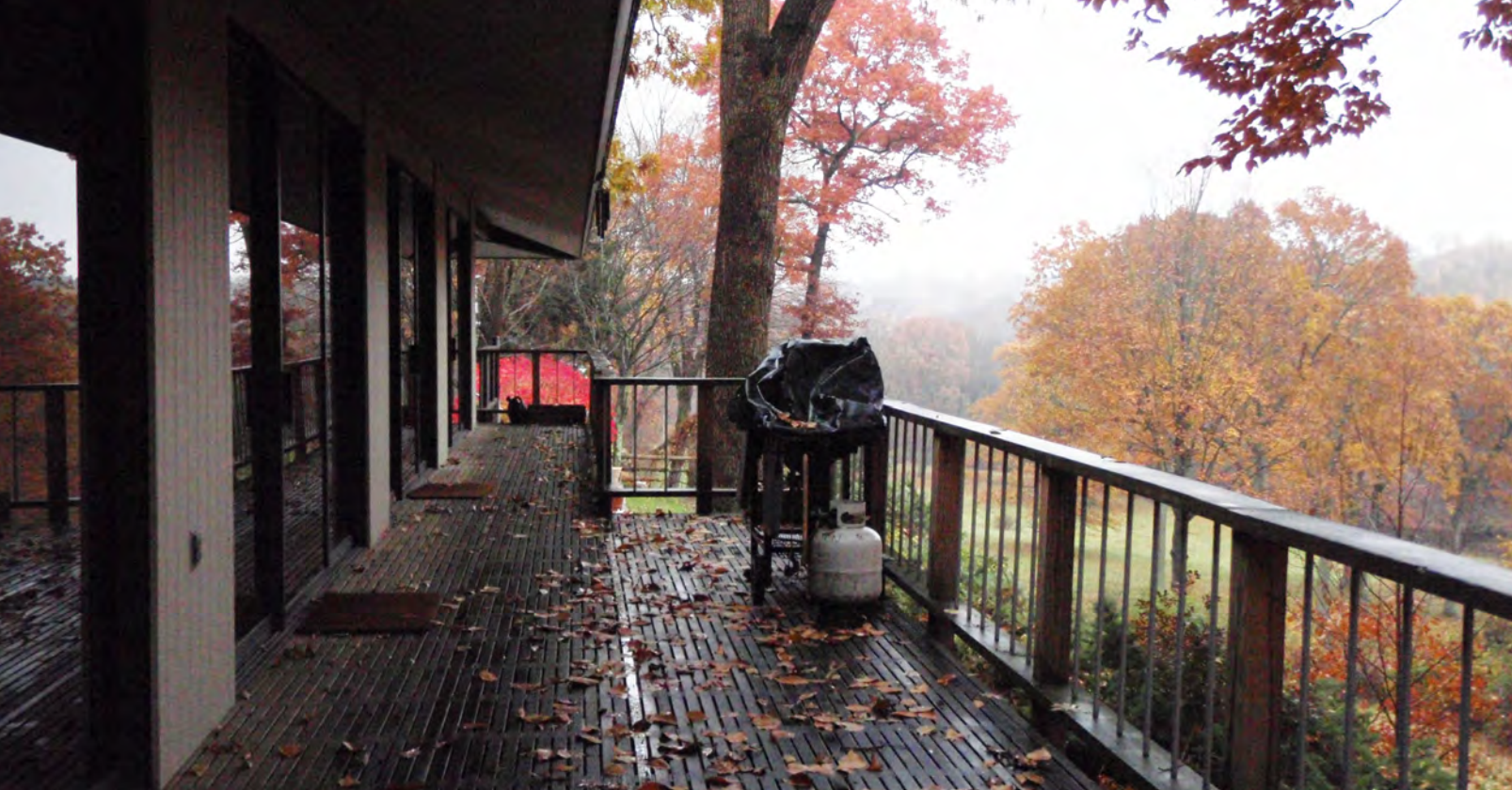
Monroe House, deck at rear façade, November 2007 (photographer: Martin Skrelunas)
