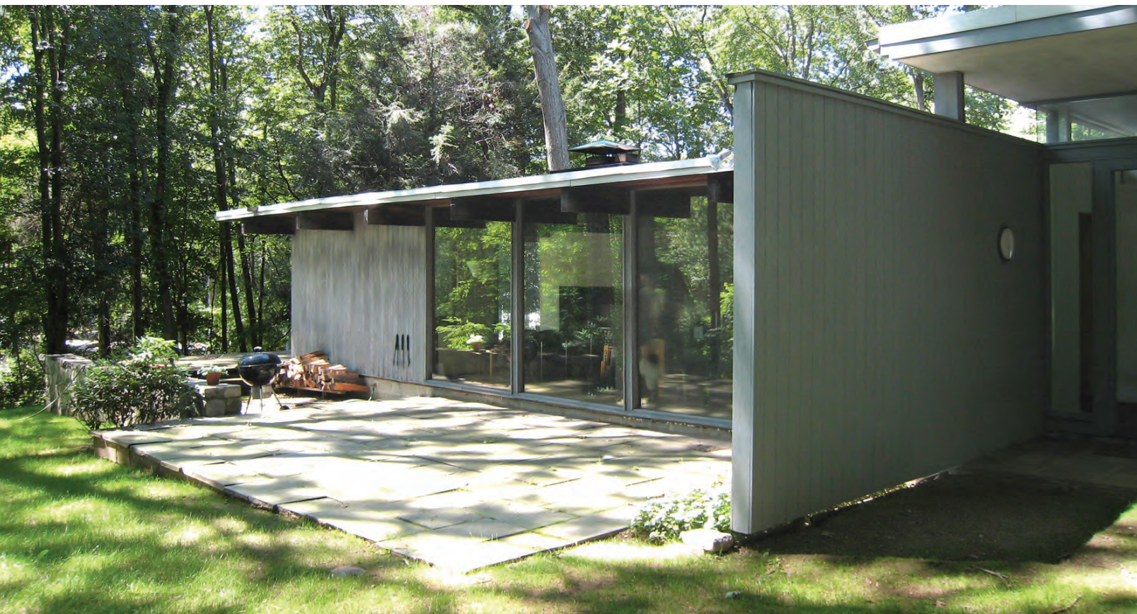
Gates House, side façade, December 2007 (photographer: Mark Markiewicz)
