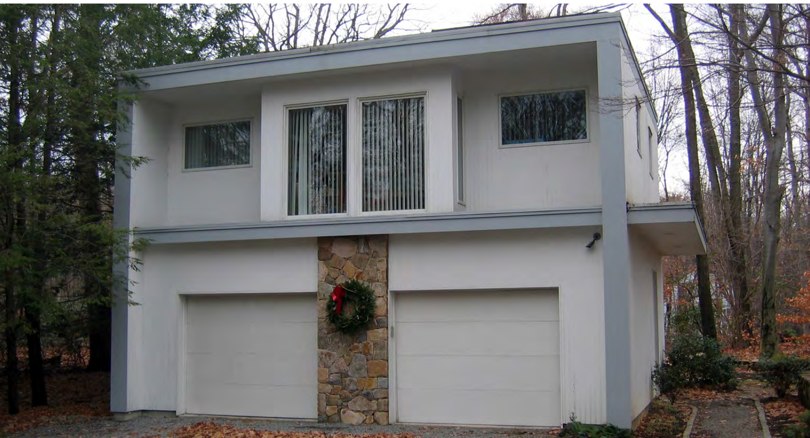
Naill House, 1993 garage/workshop, December 2007 (photographer: Eileen Brackenbury)
