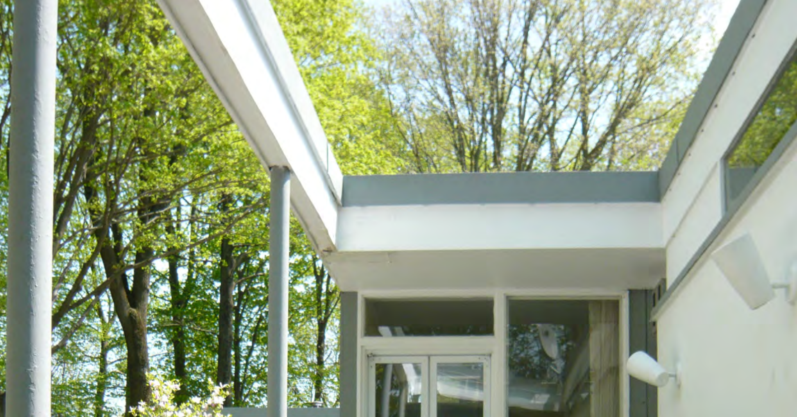
Attwood House, detail of courtyard, May 2008 (photographer: Martin Skrelunas)
