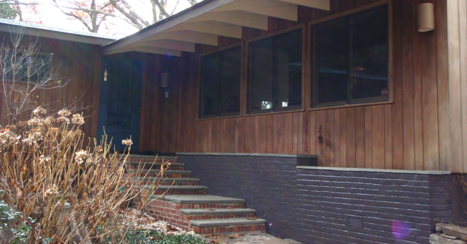
Mills House, front façade and main entrance, November 2007 (photographer: Martin Skrelunas)
