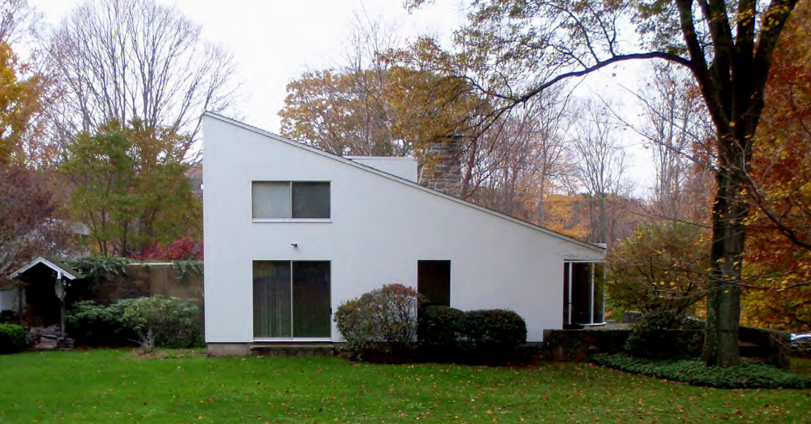
Weeks House, rear façade, November 2007 (photographer: Martin Skrelunas)
