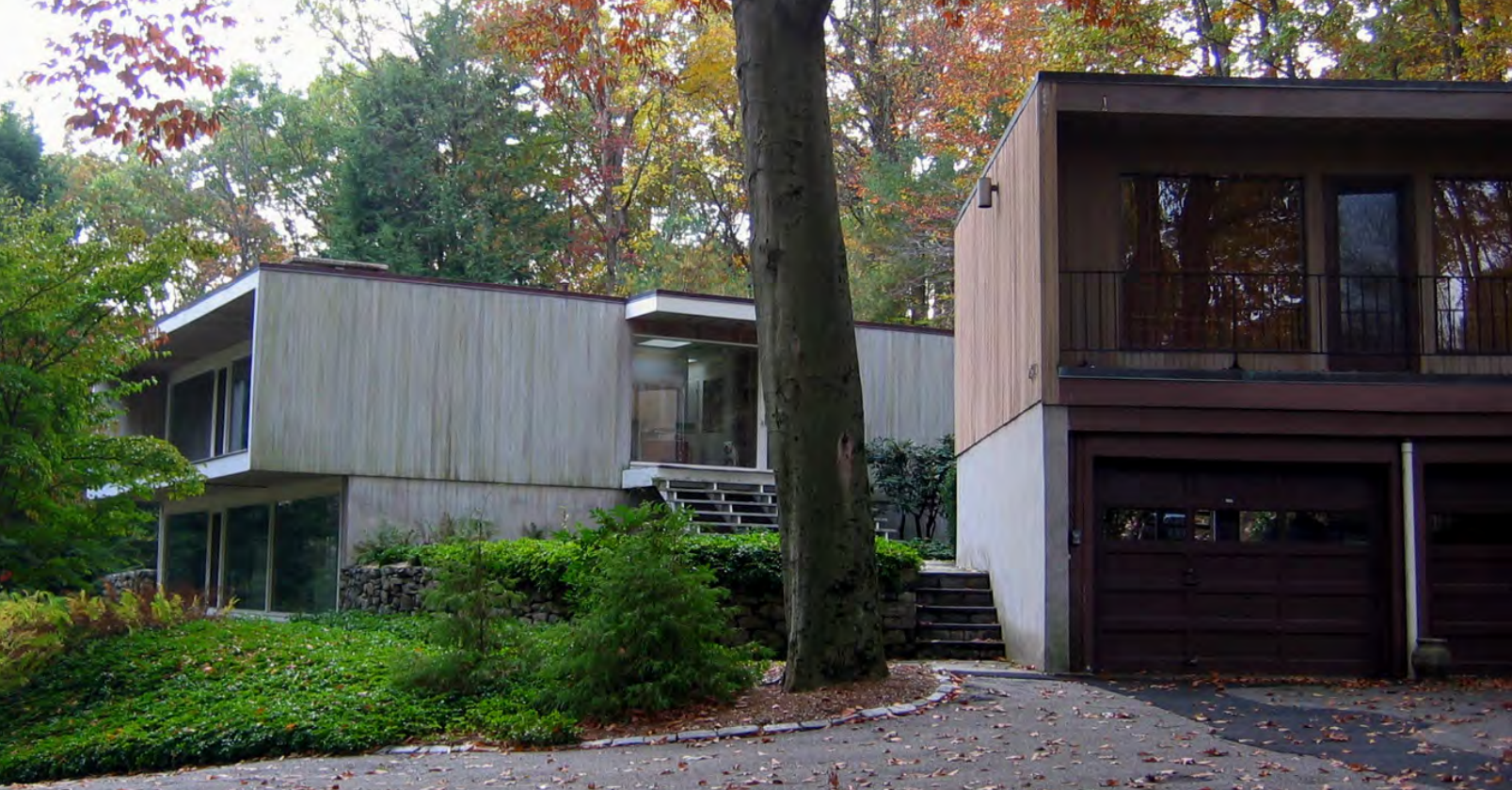
Irwin House, rear façade and garage/studio, November 2007 (photographer: Allyson Mehley)
