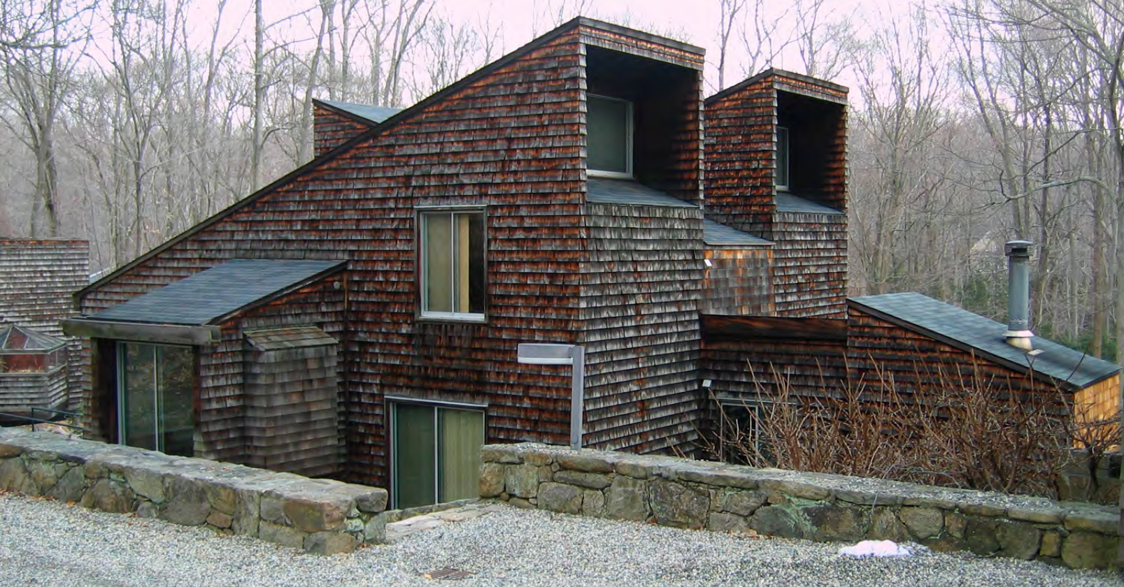
Lindstrom House, front and side façades, March 2008 (photographer: Eileen Brackenbury)
