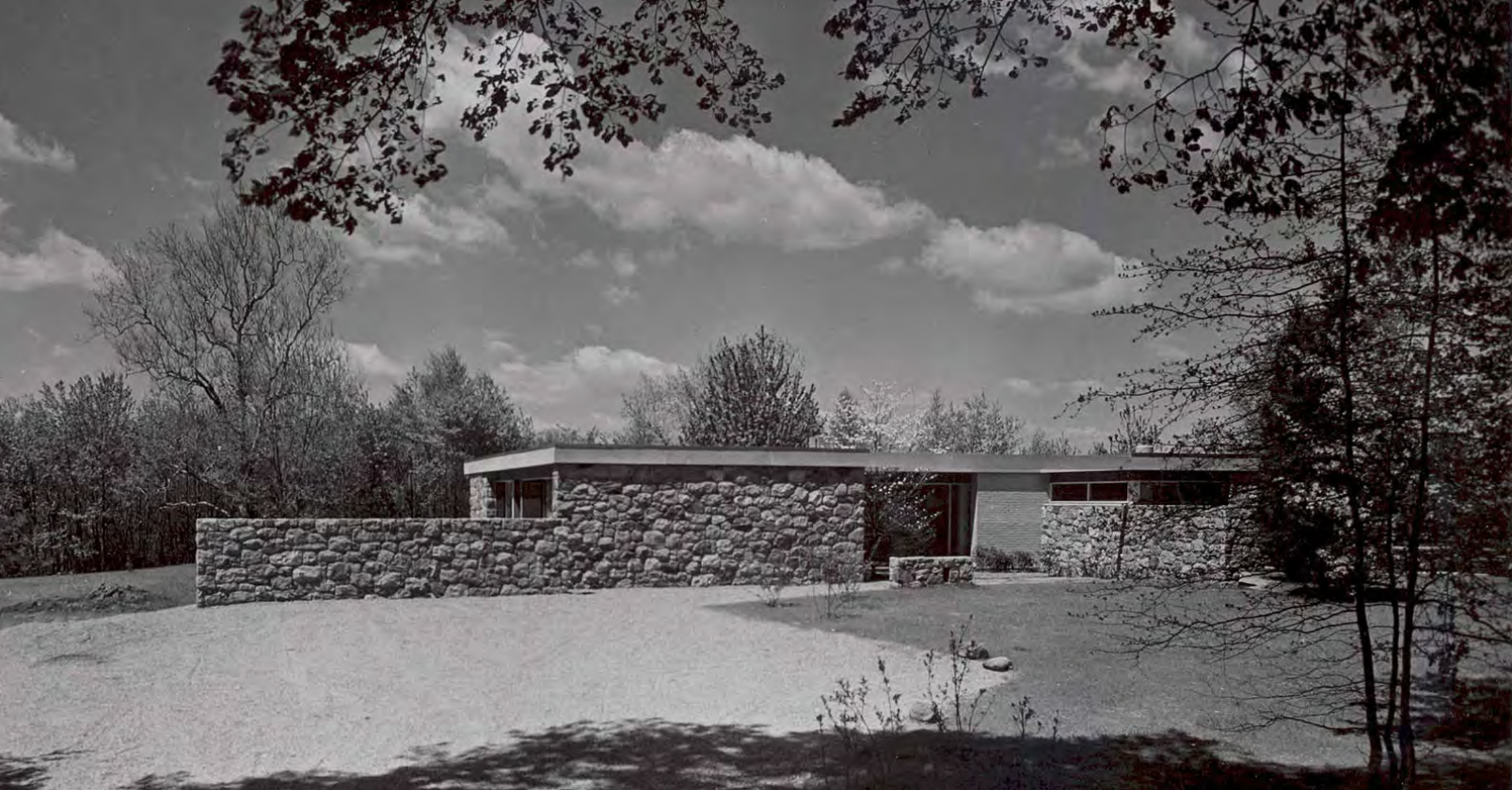
Breuer House 2, historic view, ca. 1956 (photographer: E.J. Cyr, source: New Canaan Historical Society)
