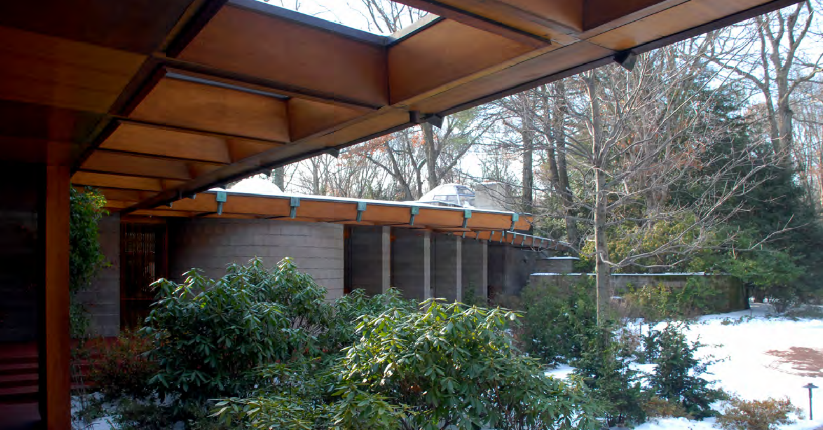
Tirranna/Rayward House, front façade, December 2007 (photographer: Ray Pepi)
