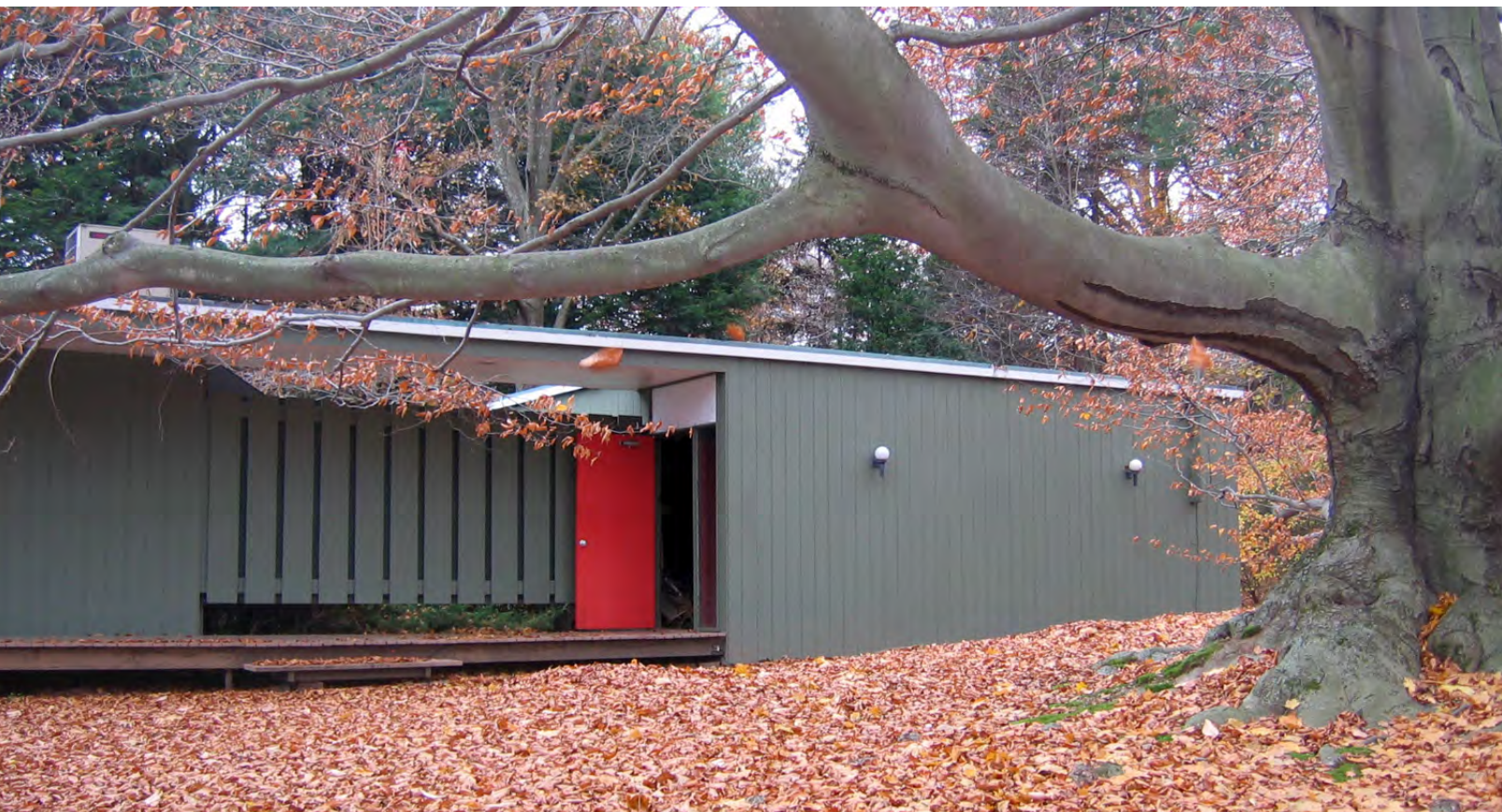
Hall House, side façade, looking towards garage and hidden courtyard, November 2007 (photographer: Eileen Brackenbury)
