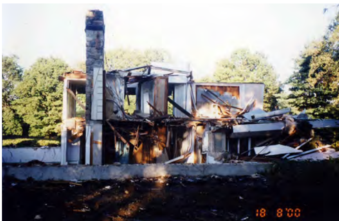
Figure 14. Dickinson House (1953) being demolished in August 2000 (source: New Canaan Historical Society)
