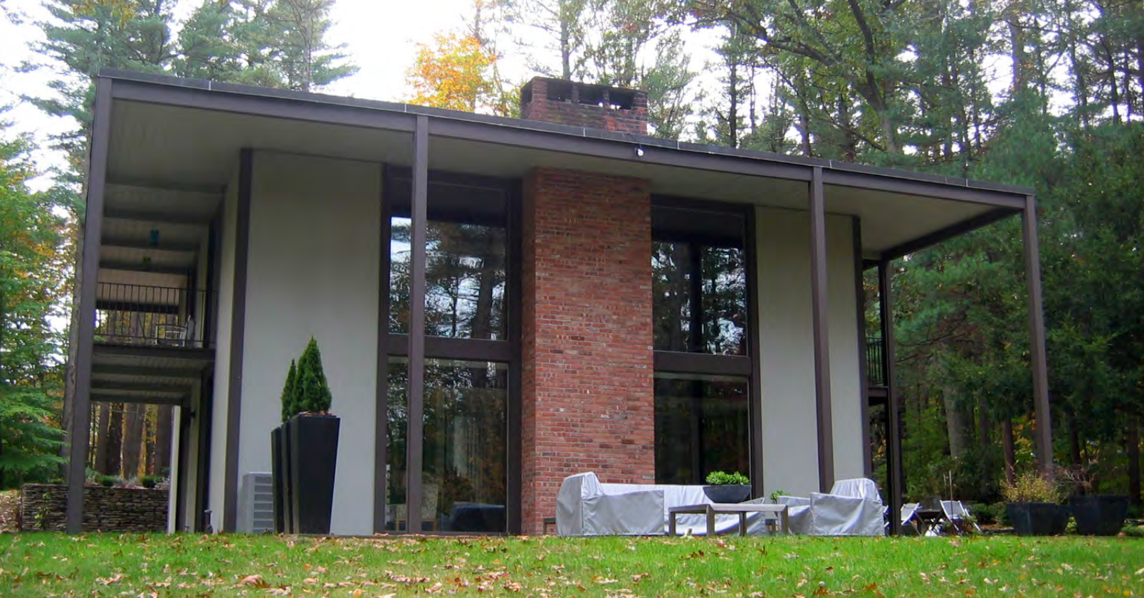
System House, rear façade, November 2007 (photographer: Allyson Mehley)
