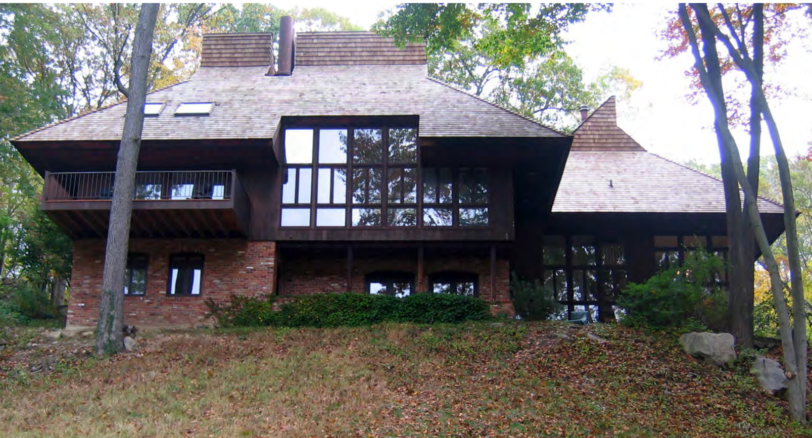
Latham House, rear façade, November 2007 (photographer: Allyson Mehley)
