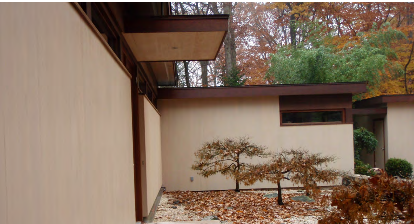
Teaze House, detail of main entrance, November 2007 (photographer: Martin Skrelunas)
