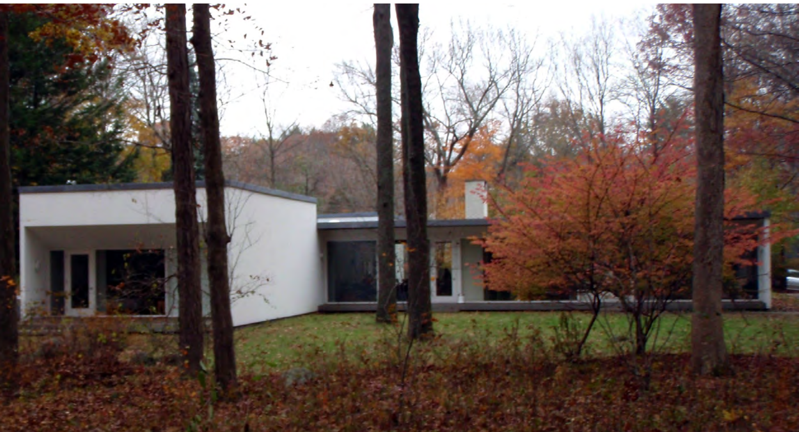
Tatum House, rear façade, November 2007 (photographer: Martin Skrelunas)
