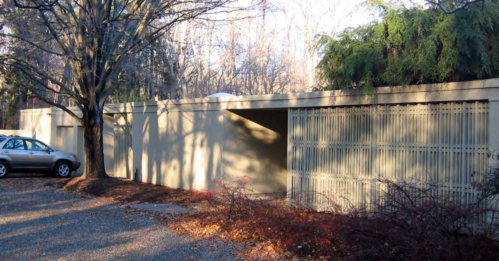
Ford House/Edward Winter House, front façade, November 2007 (photographer: Eileen Brackenbury)
