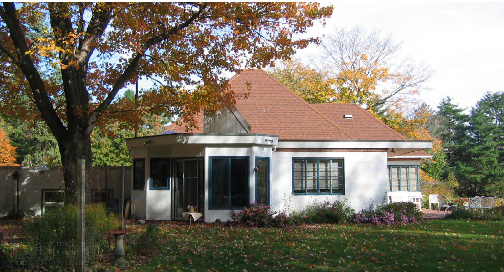
Goldmark House/Salant House, side façade, November 2007 (photographer: Eileen Brackenbury)
