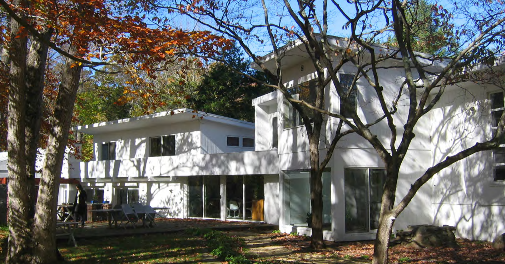
Kehm House, rear façades of original house and 1962 addition, November 2007 (photographer: Eileen Brackenbury)
