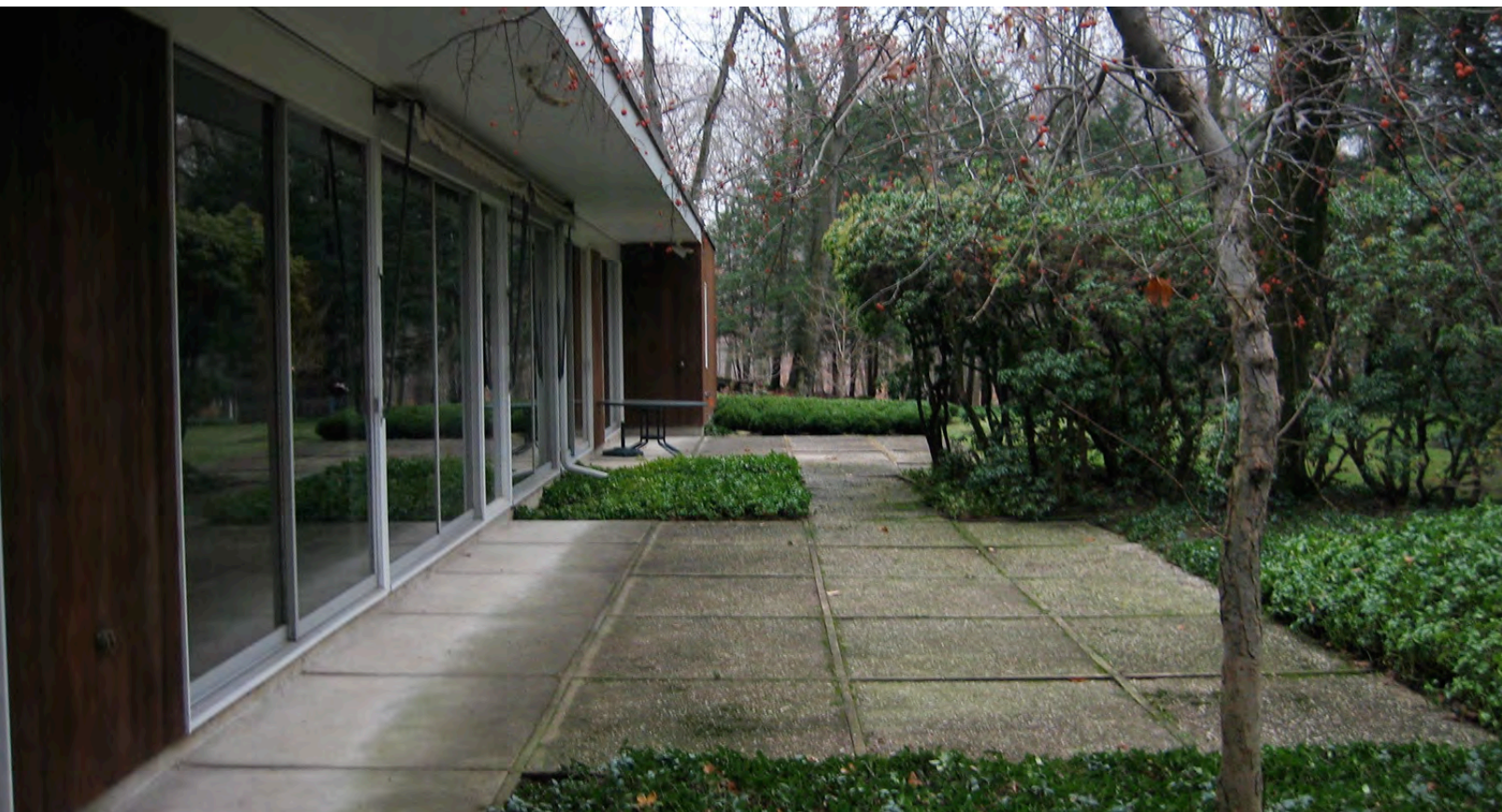
Crichton House, rear façade, December 2007 (photographer: Heather McGrath)
