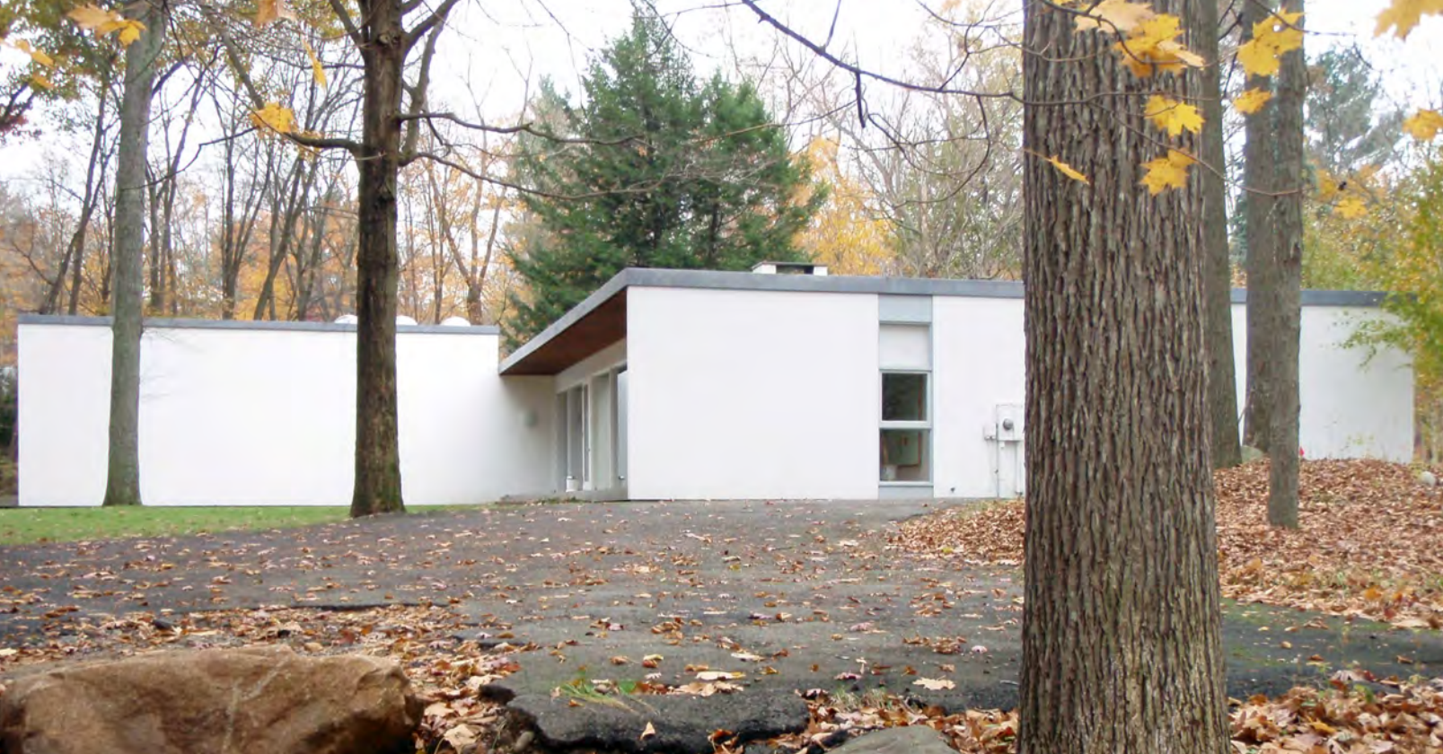
Tatum House, side façade, November 2007 (photographer: Martin Skrelunas)
