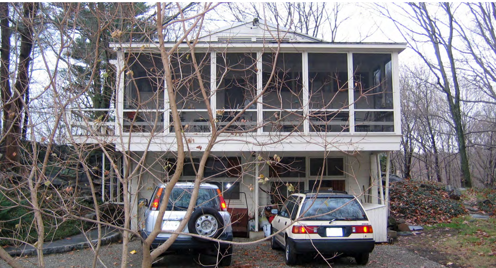
Talbert House, side façade showing original garage entrances at ground level, December 2007 (photographer: Eileen Brackenbury)
