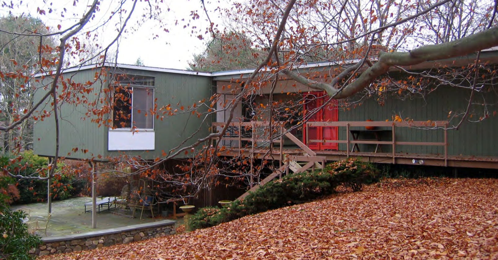
Hall House, side façade, looking towards main entrance and ca.1975 addition, November 2007 (photographer: Eileen Brackenbury)
