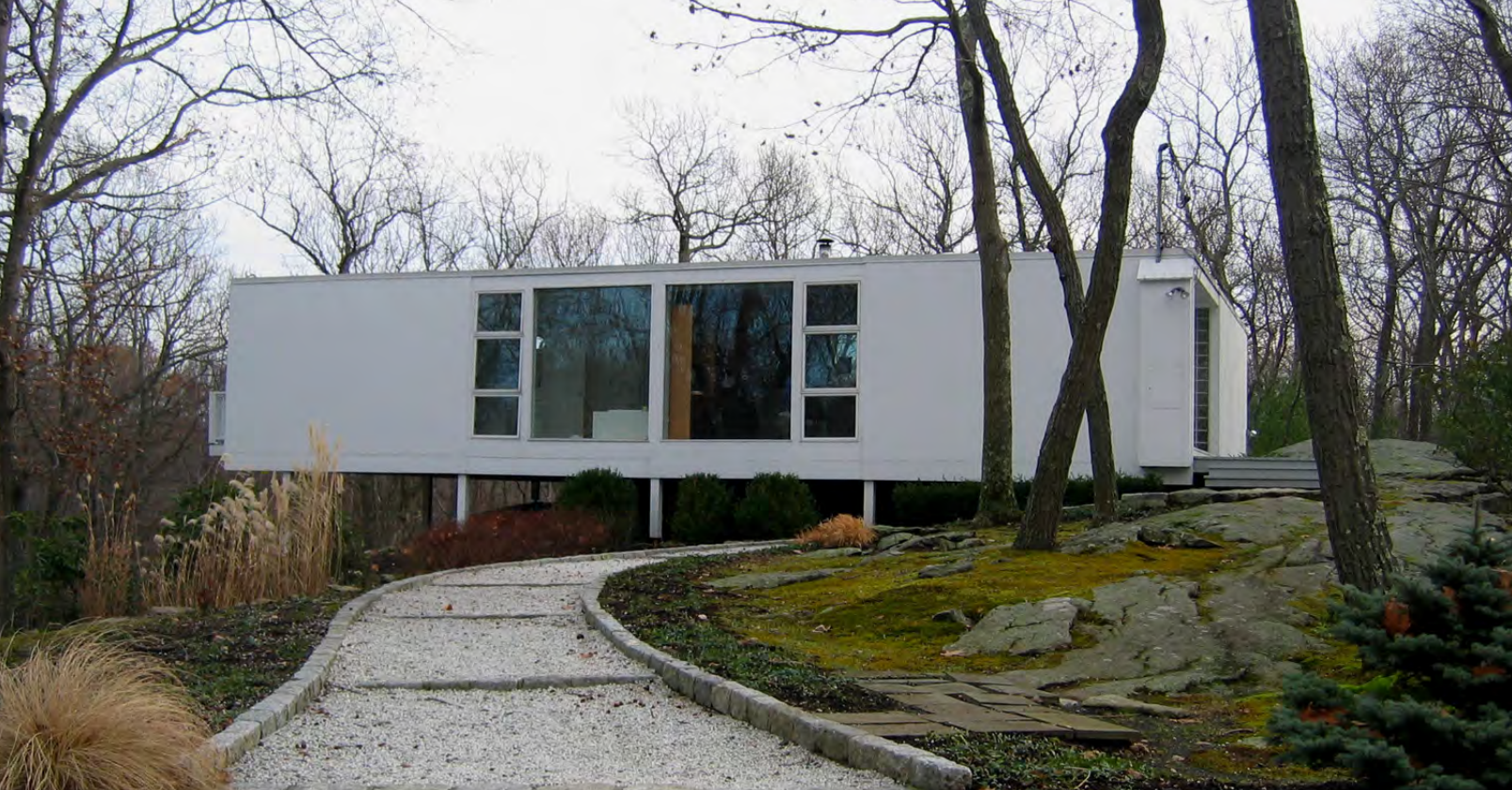
Lee House 1, north façade, December 2007 (photographer: Eileen Brackenbury)
