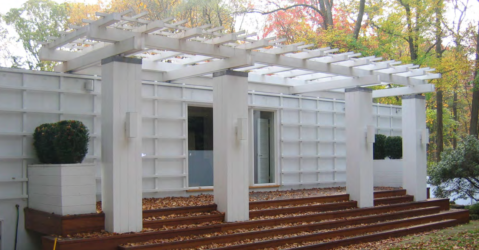
Gratwick House, front façade showing altered main entrance, November 2007 (photographer: Allyson Mehley)
