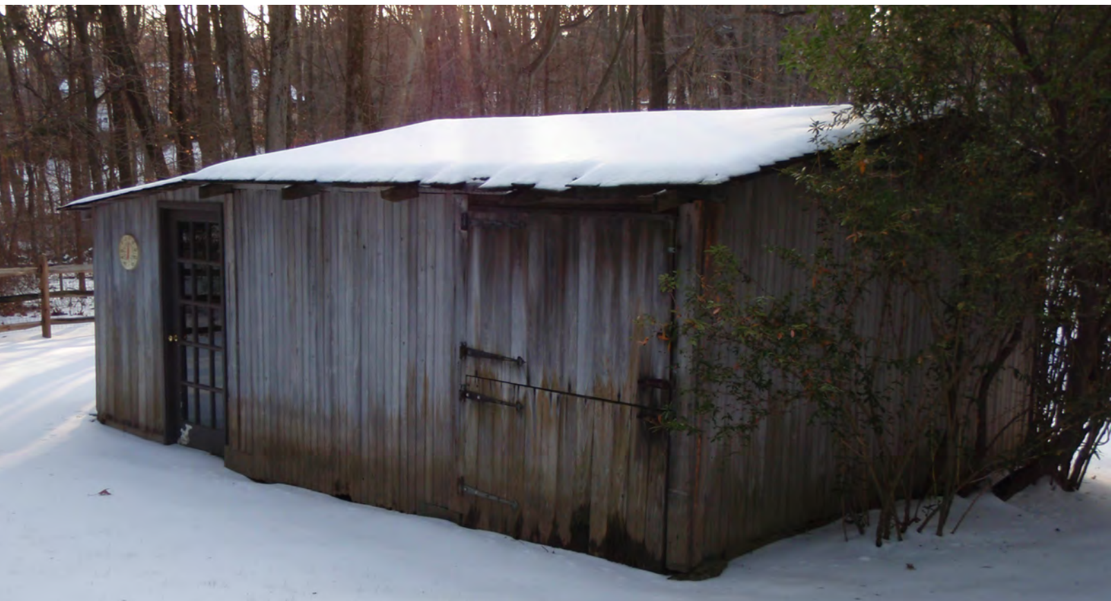
Daine House, stable, December 2007 (photographer: Martin Skrelunas)
