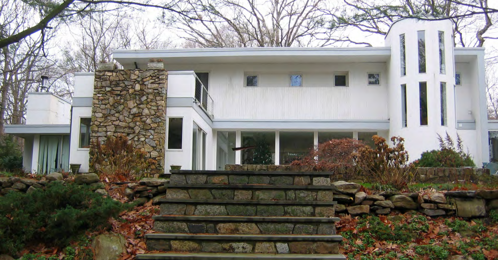
Naill House, rear façade, December 2007 (photographer: Eileen Brackenbury)
