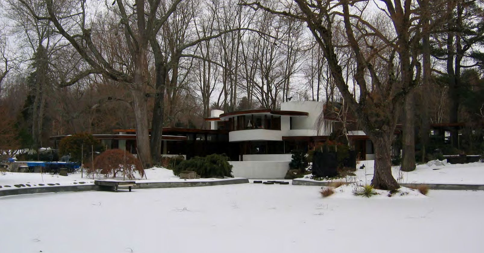
Leuthold House, front façade, December 2007 (photographer: Eileen Brackenbury)
