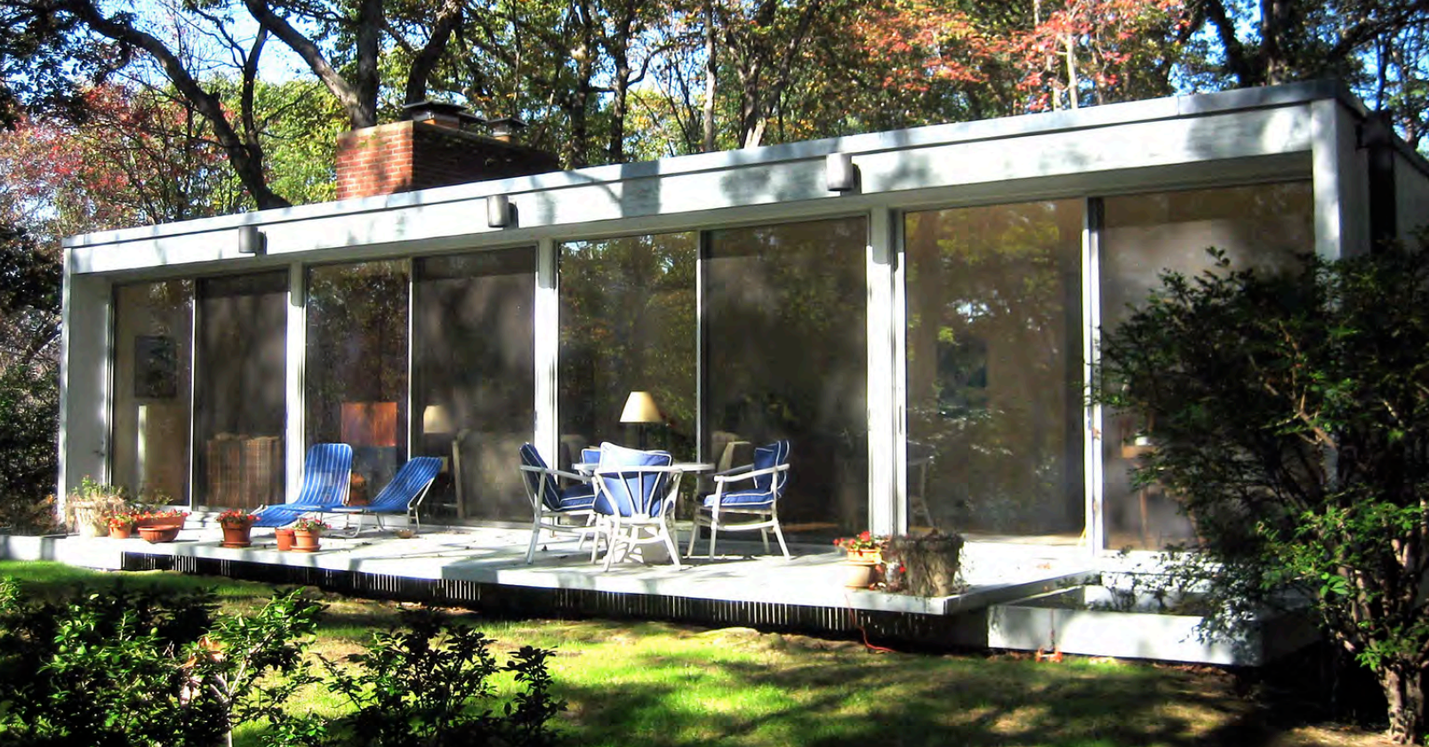
Parsons House, rear façade, October 2007 (photographer: Eileen Brackenbury)
