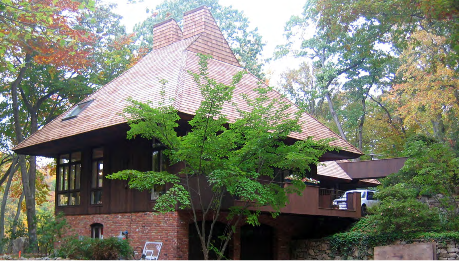
Latham House, front façade, November 2007 (photographer: Allyson Mehley).
