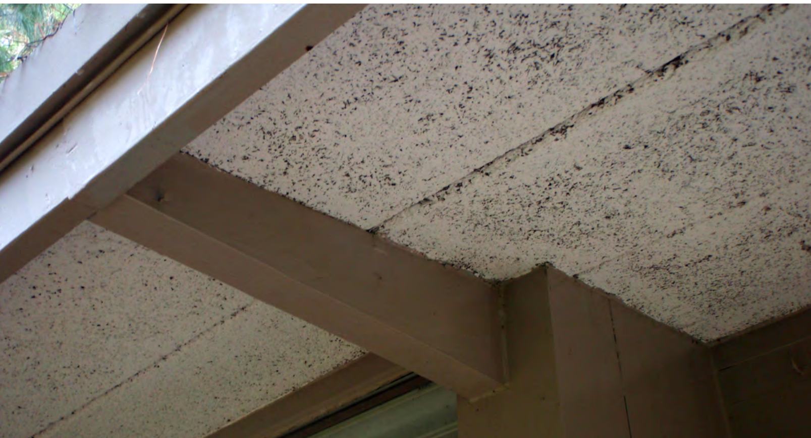
Risom House, detail of Durisol material, November 2007 (photographer: Martin Skrelunas)
