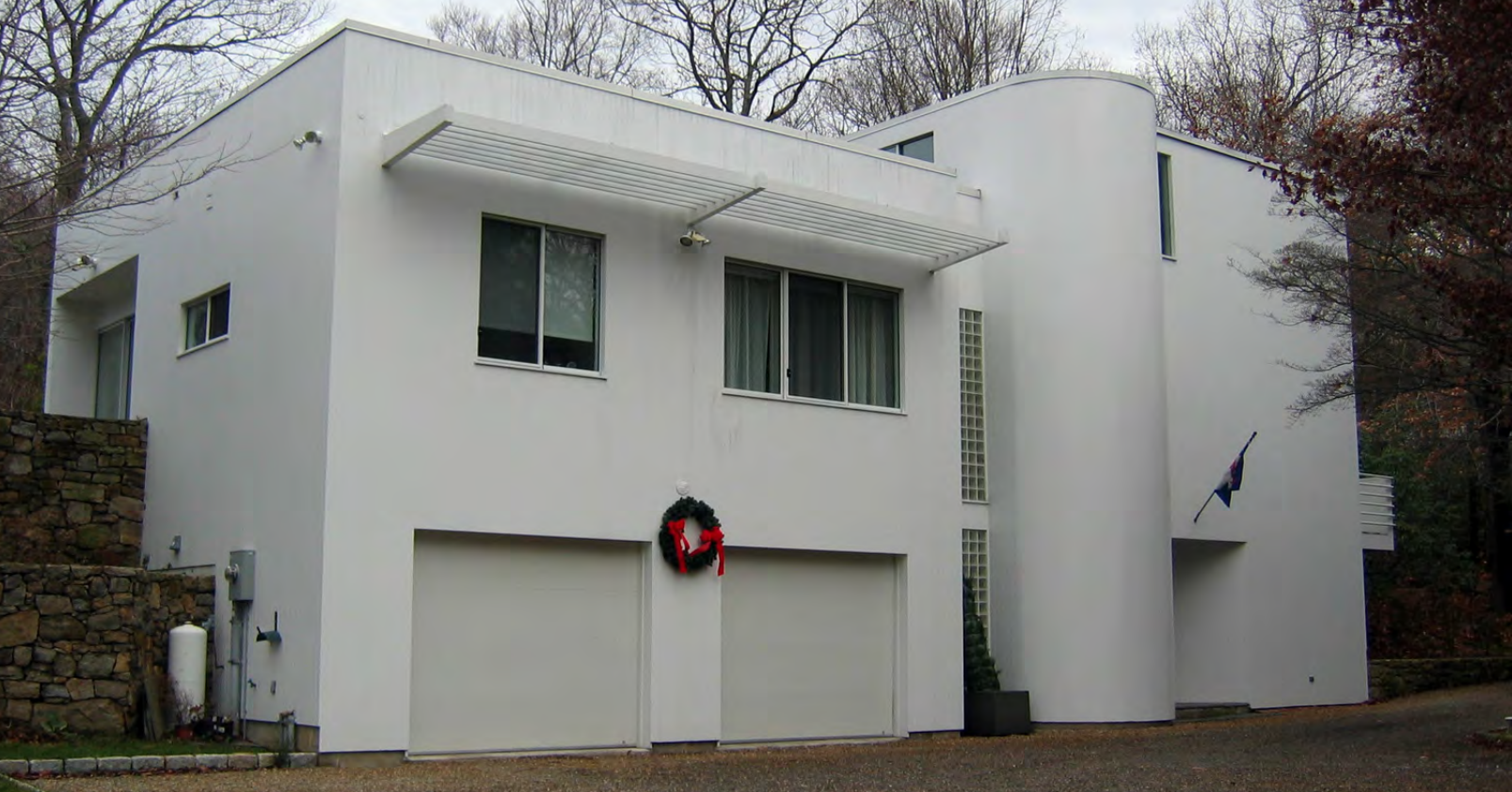
Arit House, front façade, December 2007 (photographer: Eileen Brackenbury)
