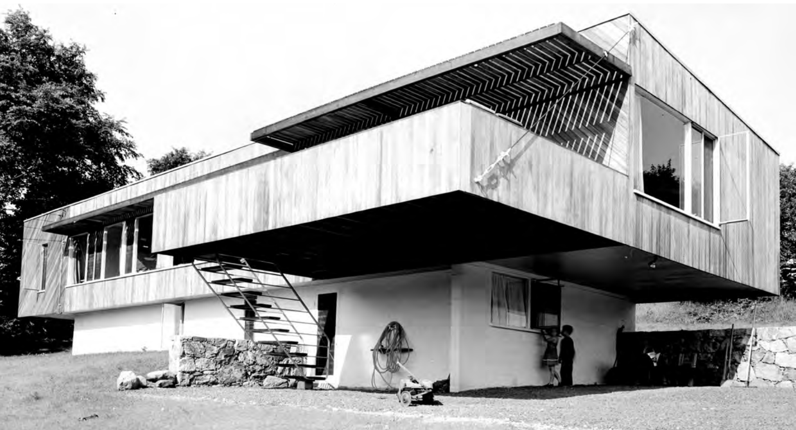
Breuer House 1, historic photograph showing original cantilevers, unknown date (photographer: Pedro Guerrero, source: Philip Johnson Glass House)
