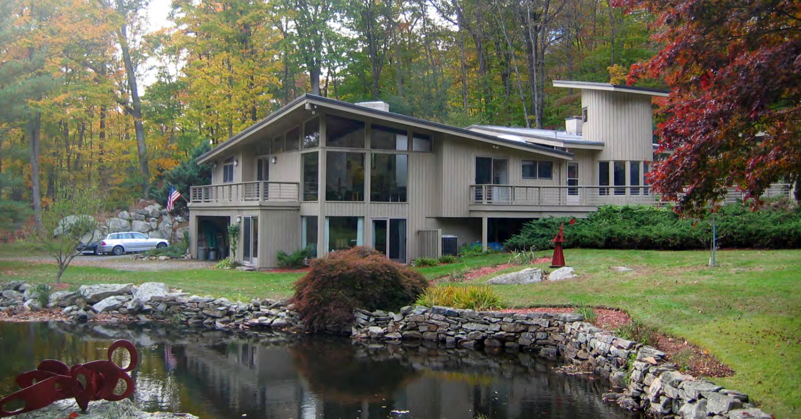
James House, front and side façades, November 2007 (photographer: Eileen Brackenbury)
