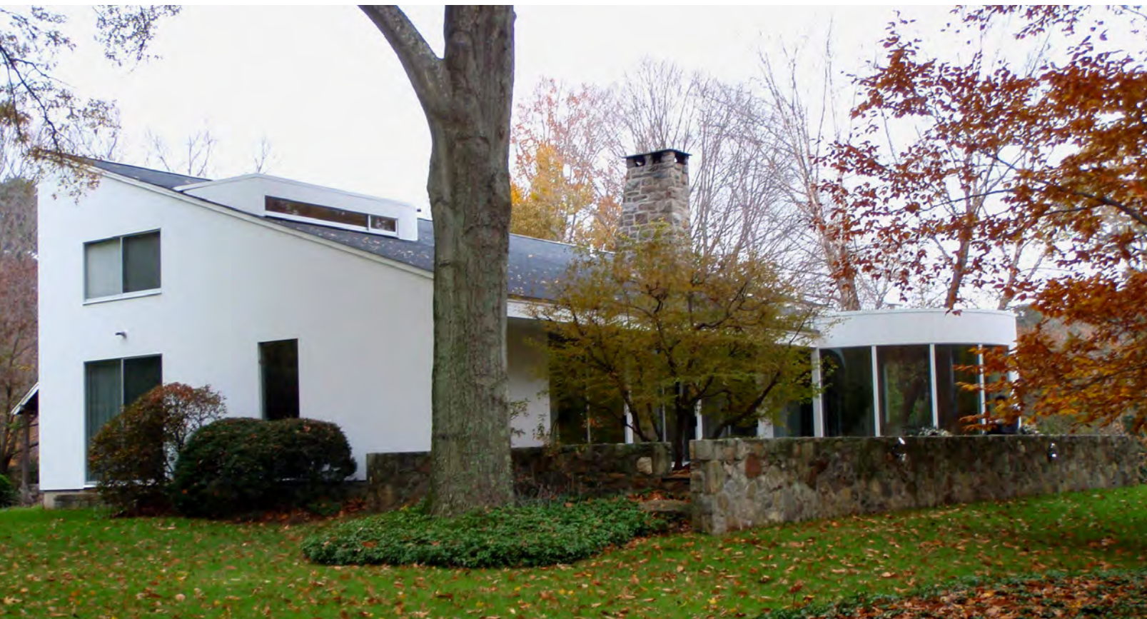
Weeks House, side façade, November 2007 (photographer: Martin Skrelunas)
