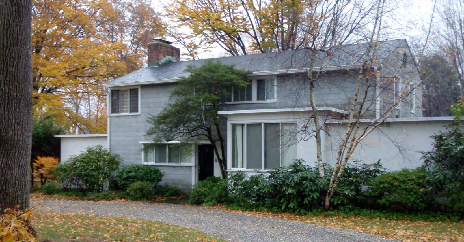
Mills House 1, view from street, November 2007 (photographer: Martin Skrelunas)
