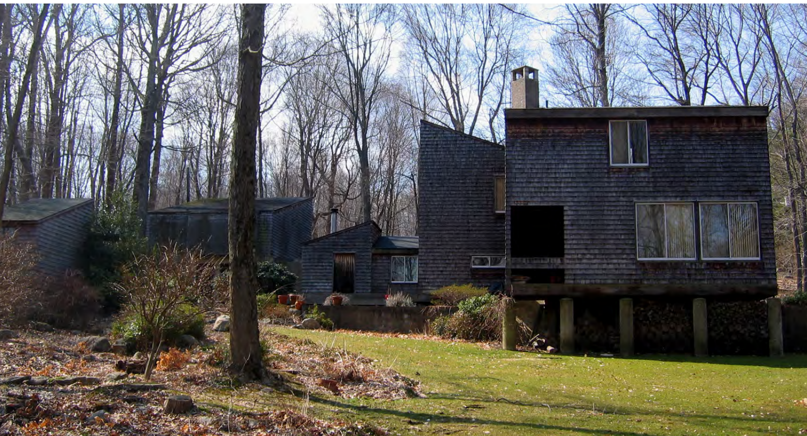
Lindstrom House, rear façade, March 2008 (photographer: Eileen Brackenbury)
