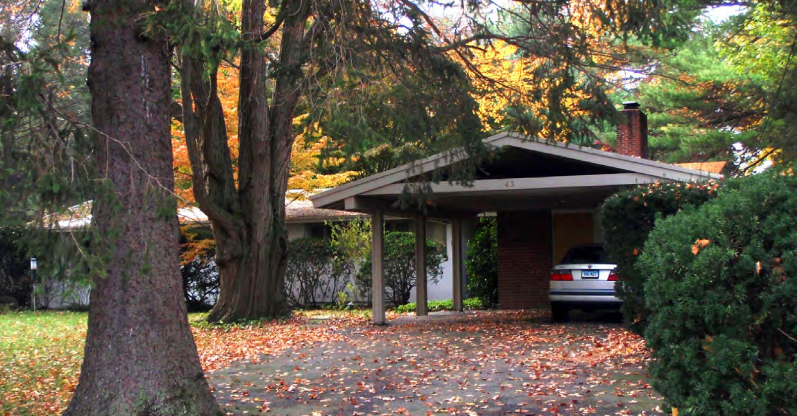
Risom House, front façade, November 2007 (photographer: Martin Skrelunas)
