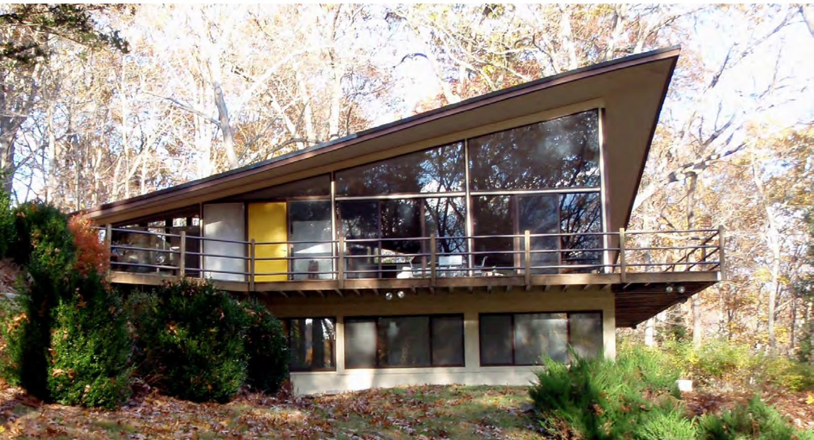
Evans House, side façade, November 2007 (photographer: Heather McGrath)
