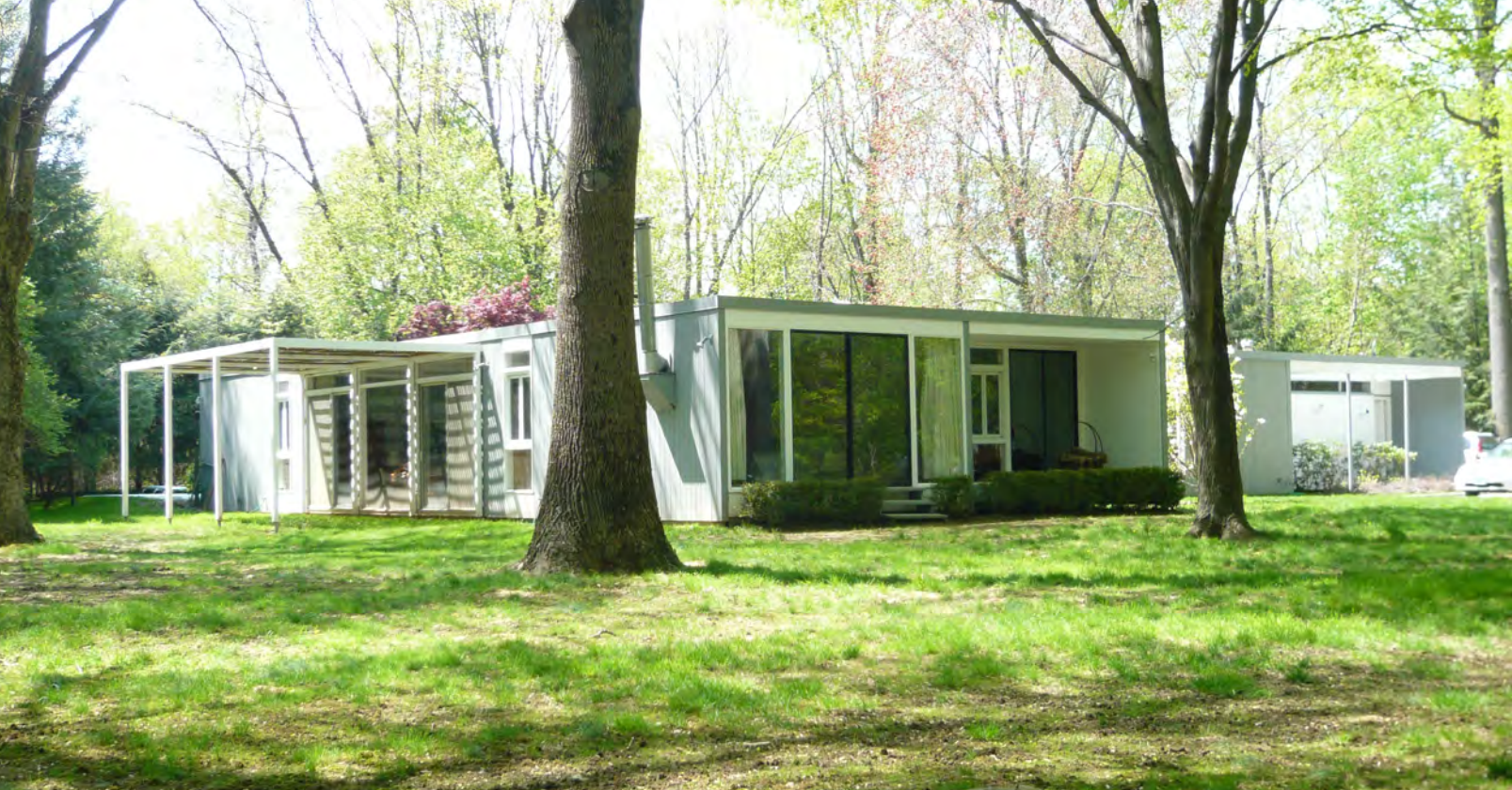
Attwood House, front and side façades, May 2008 (photographer: Martin Skrelunas)
