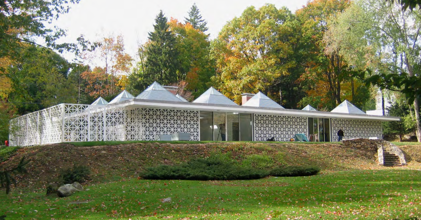
Celanese House, rear façade, October 2007 (photographer: Eileen Brackenbury)
