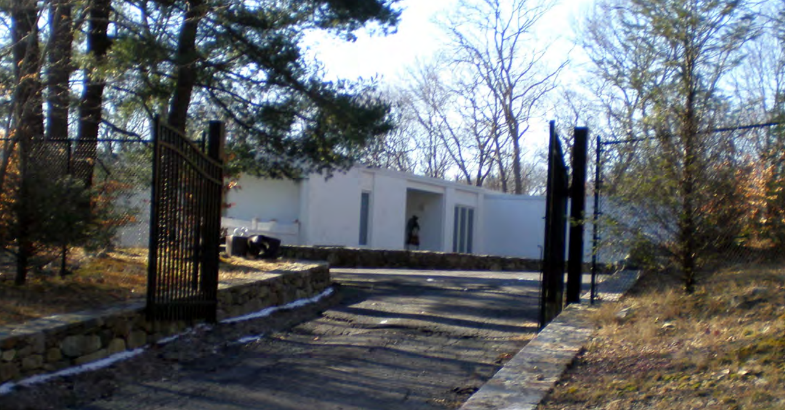
Fiore House, view from street, February 2008 (photographer: Allyson Mehley)
