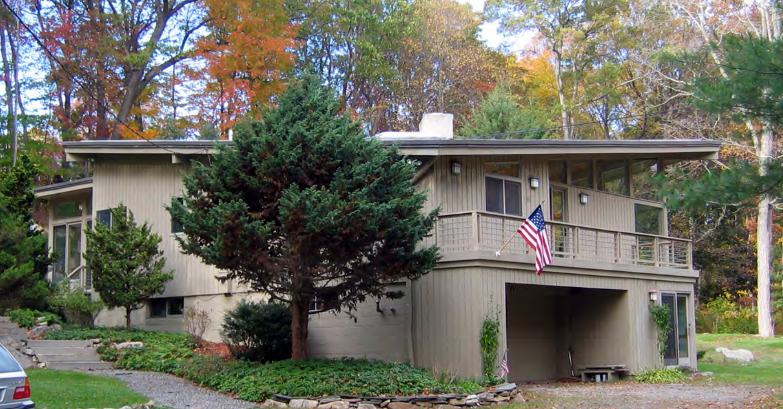
James House, front façade, November 2007 (photographer: Eileen Brackenbury)
