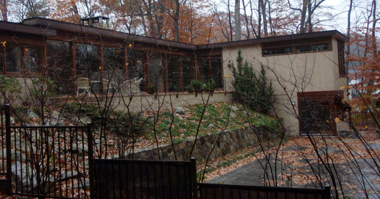
Teaze House, rear façade, November 2007 (photographer: Martin Skrelunas)
