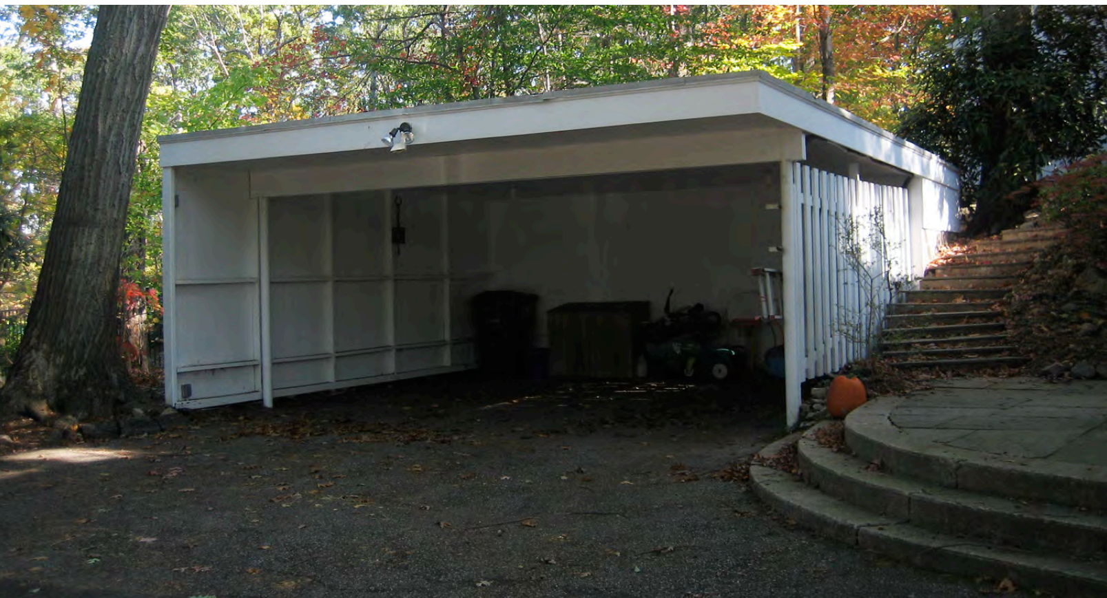
Beaven Mills House, carport, October 2007 (photographer: Eileen Brackenbury)
