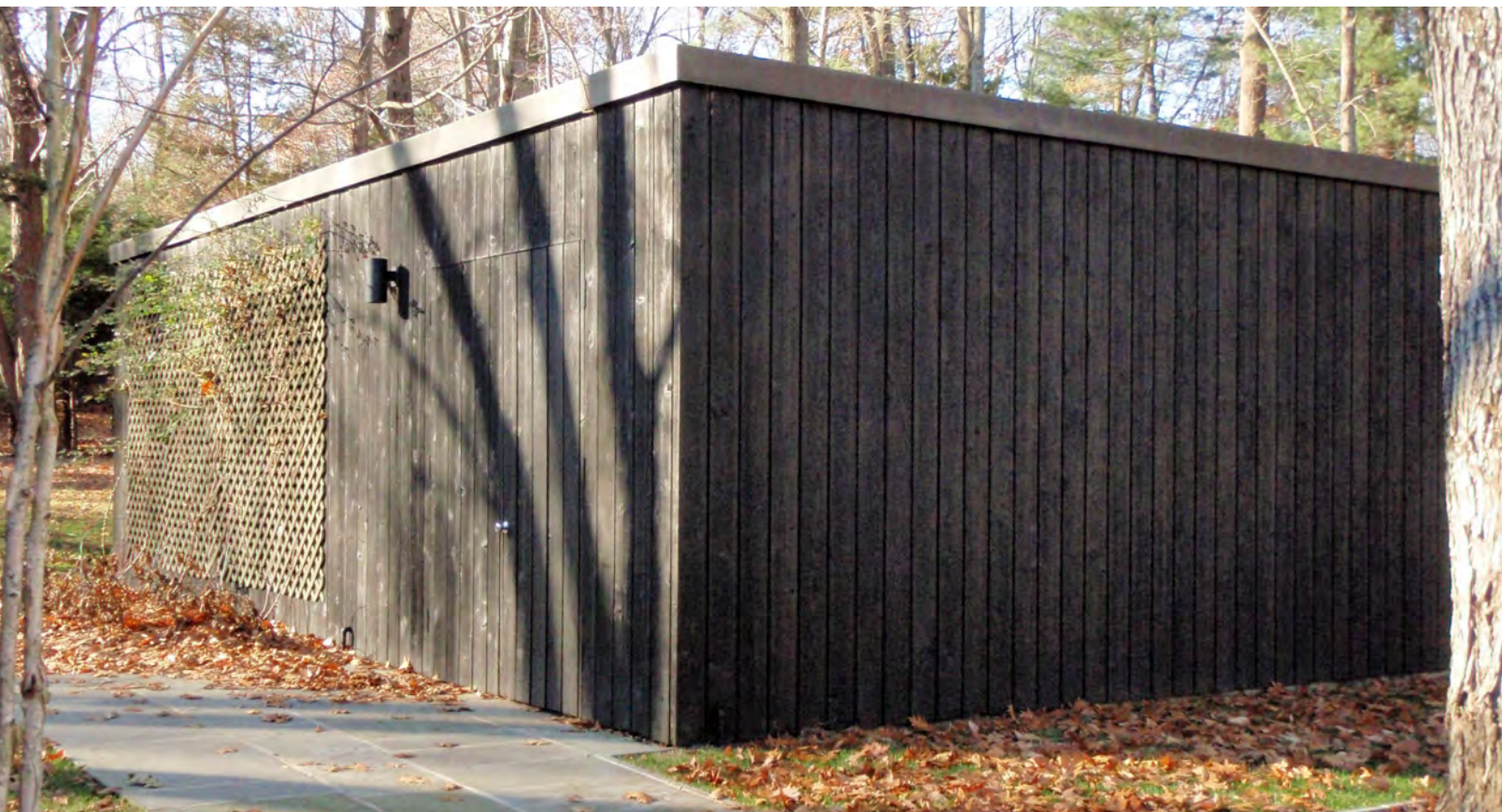
Chivis House, side façade of garage, November 2007 (photographer: Martin Skrelunas)
