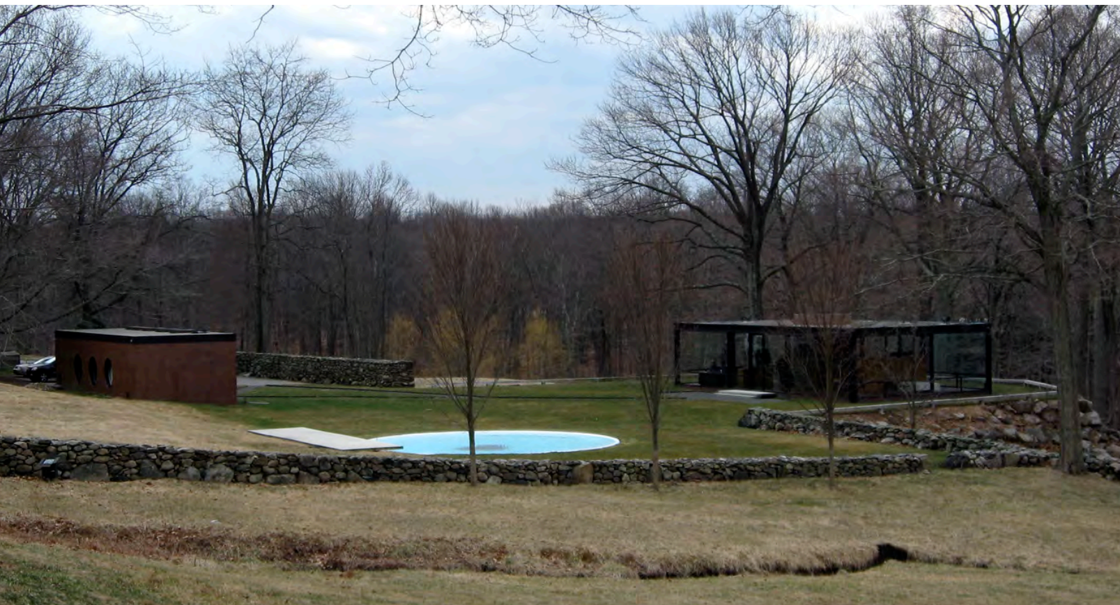
Philip Johnson Glass House, view of Brick House, Glass House, and swimming pool, March 2008 (photographer: Eileen Brackenbury)
