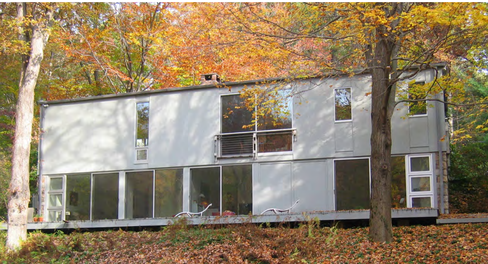
Becker House, rear façade, November 2007 (photographer: Eileen Brackenbury)
