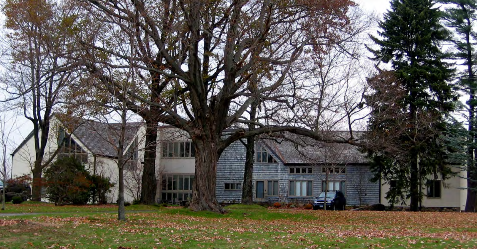
Brandon House, view from street, November 2007 (photographer: Martin Skrelunas)
