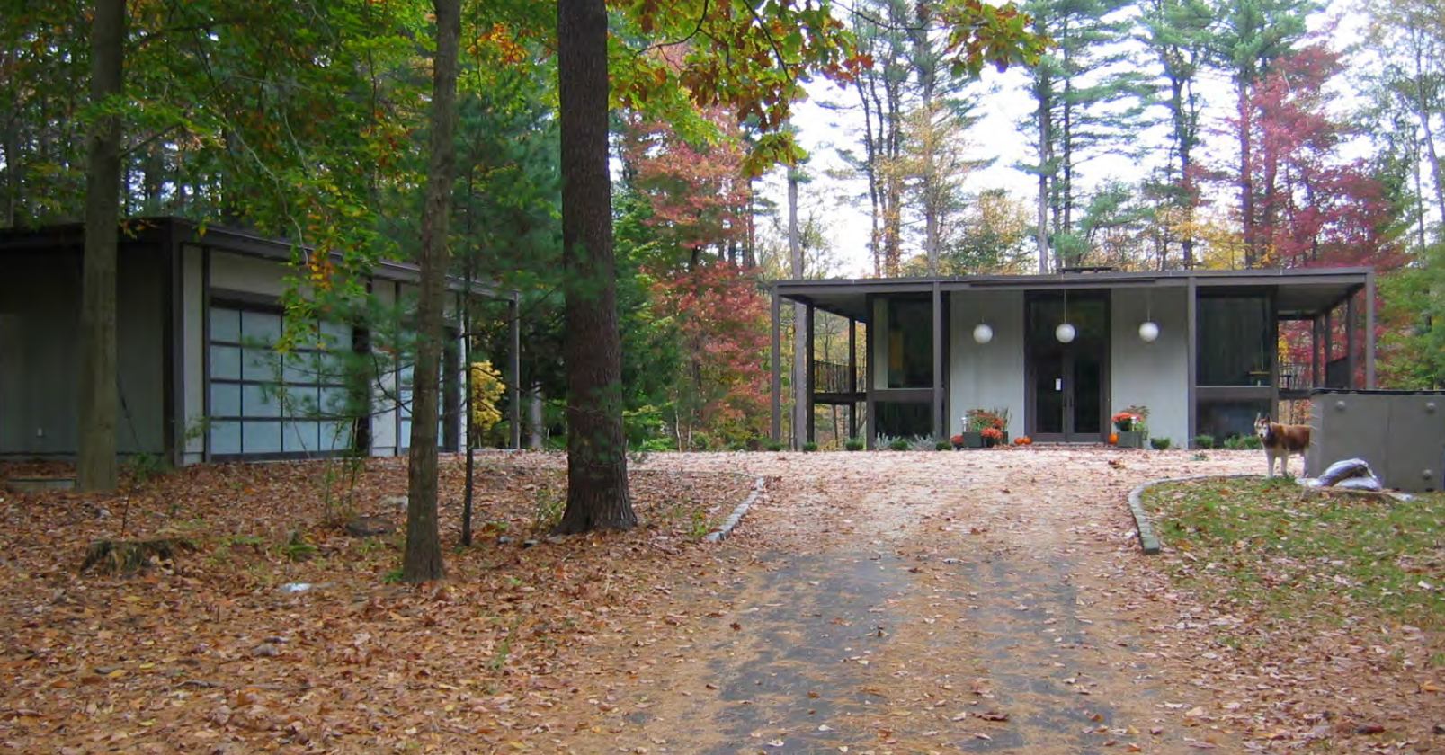
System House, front façade and garage, November 2007 (photographer: Allyson Mehley)
