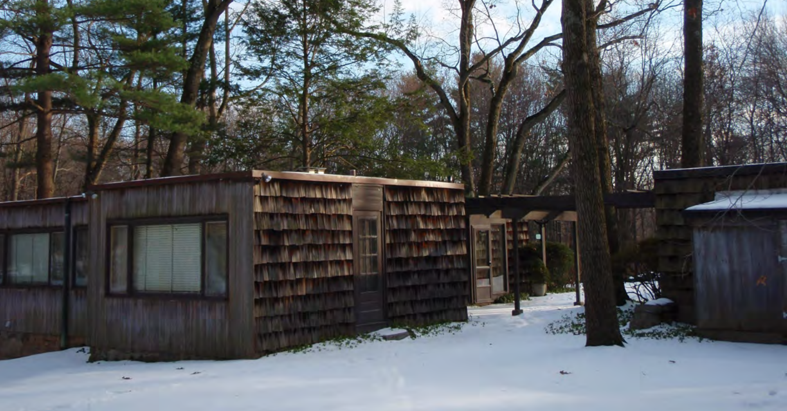
Daine House, rear and side façades, December 2007 (photographer: Martin Skrelunas)
