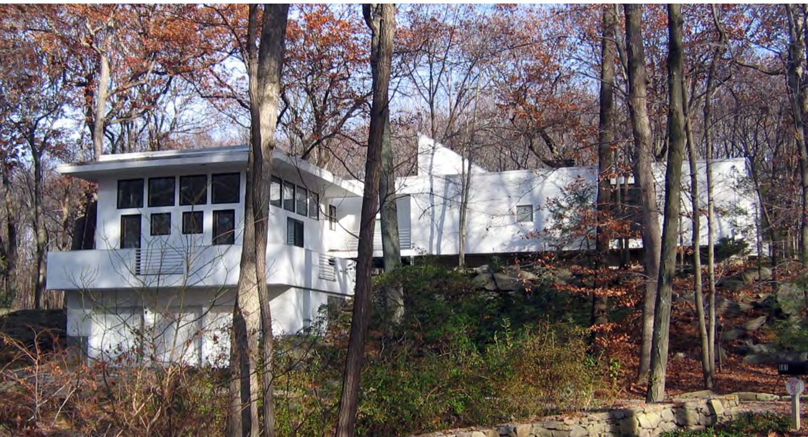
Spotts House, front façade of additions, November 2007 (photographer: Eileen Brackenbury)
