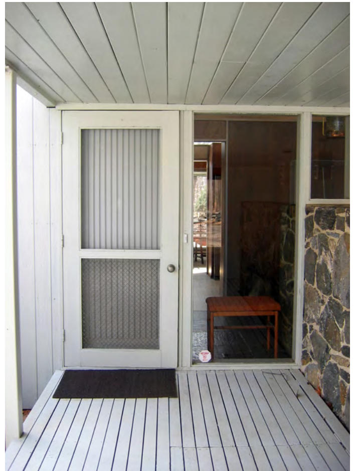
Figure 11. Melville House, service entry, 2008. Architects Gates and Ford used extended end walls of fieldstone at the entry and living room to create a connection between interior and exterior spaces. Note how the fieldstone wall extends through the glass wall into the entry (photographer: Eileen Brackenbury)
