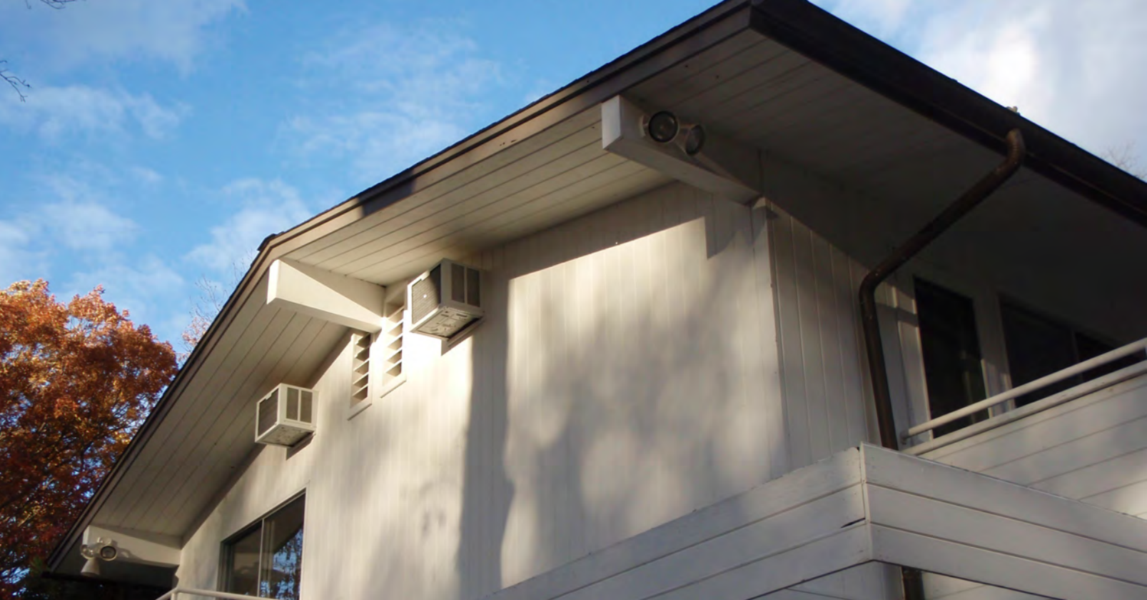
McKay House, detail of soffit, November 2007 (photographer: Heather McGrath)
