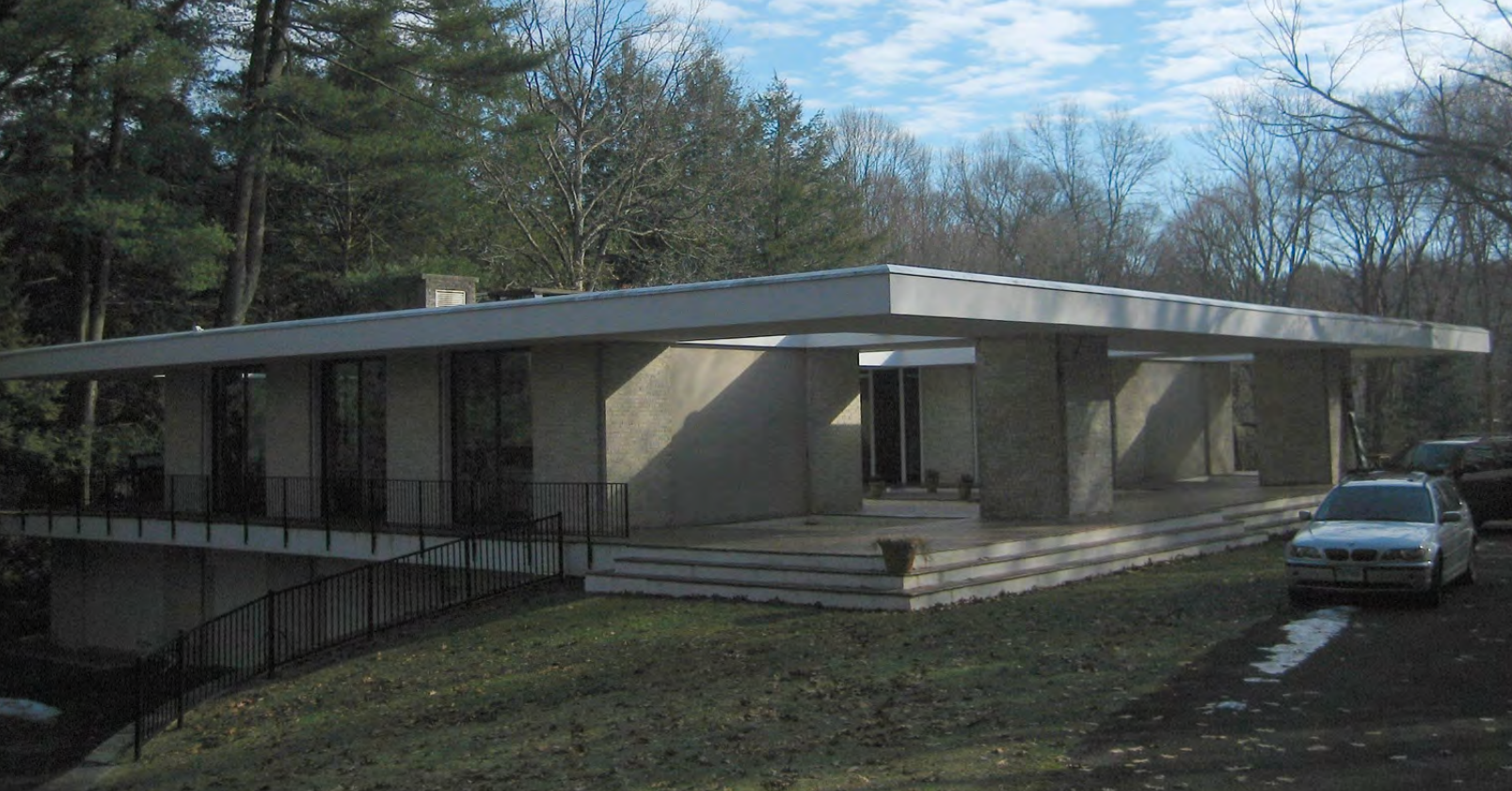
Day House, oblique view of the front and side façades, January 2008 (photographer: Heather McGrath)
