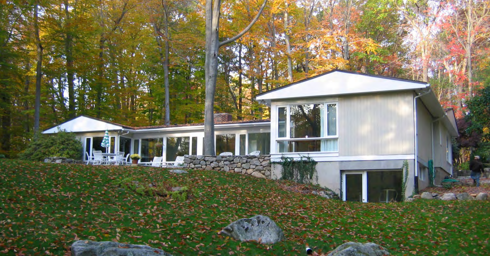
Barlow House, rear façade, November 2007 (photographer: Eileen Brackenbury)
