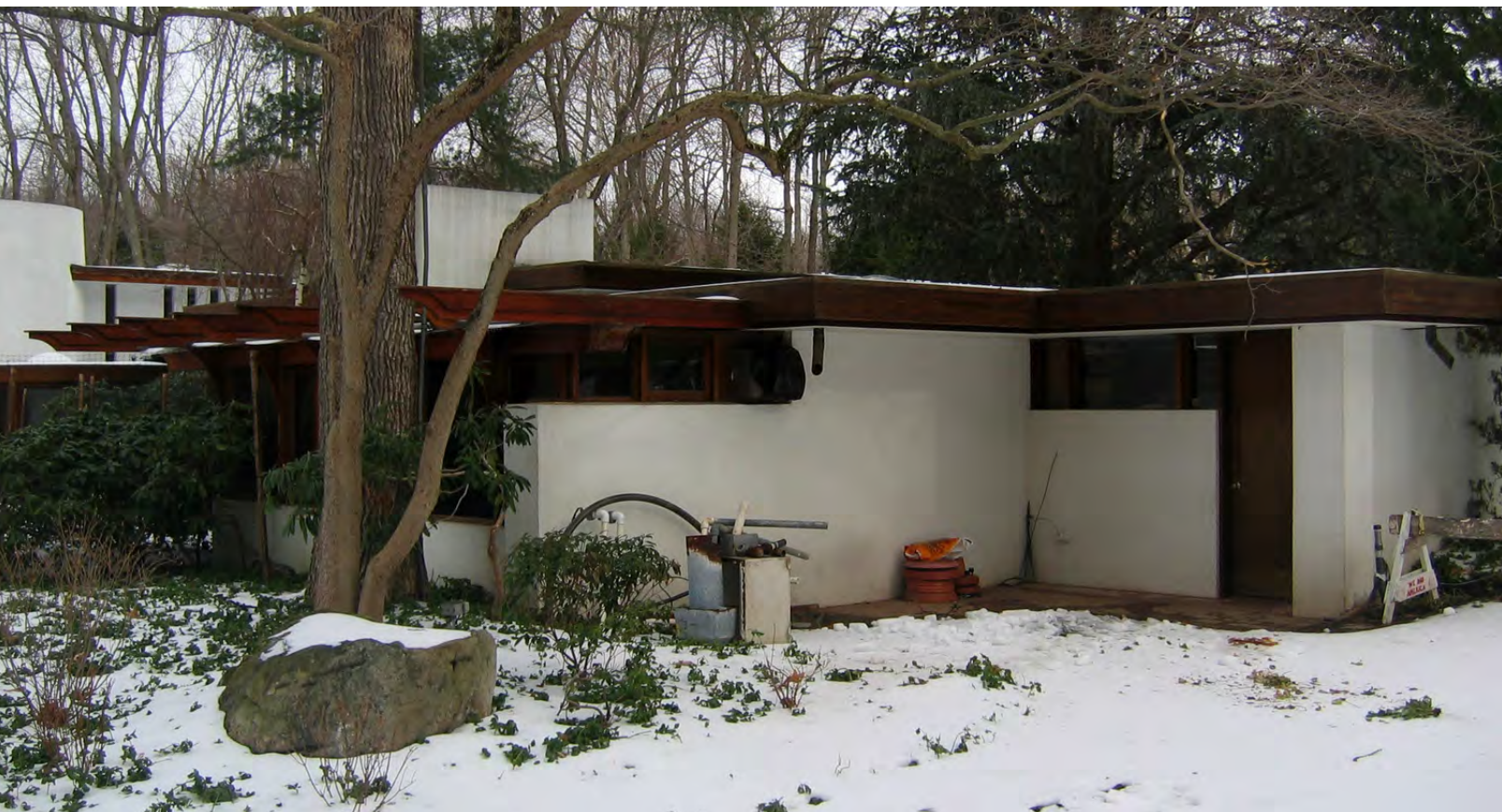
Leuthold House, guesthouse, December 2007 (photographer: Eileen Brackenbury)
