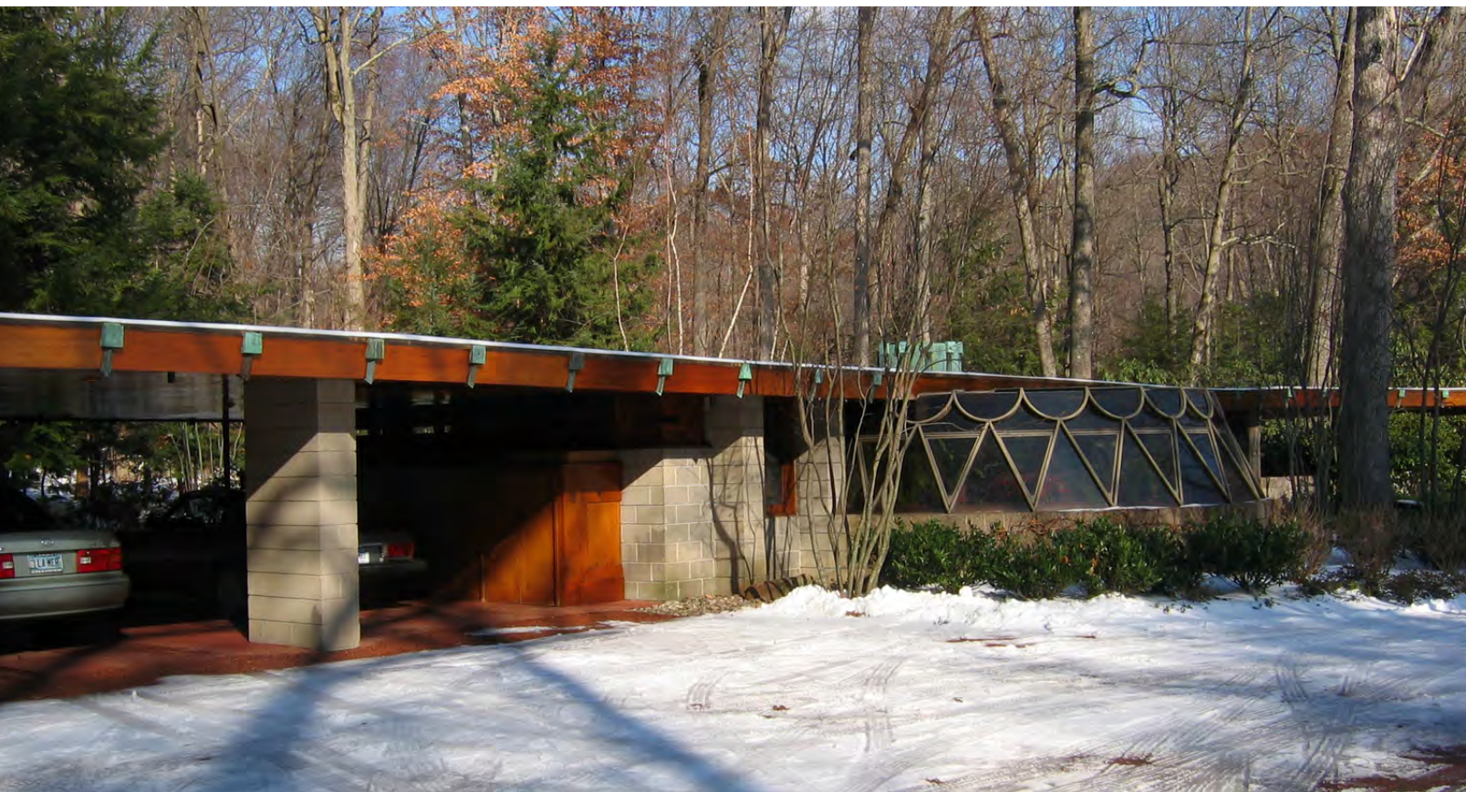
Tirranna/Rayward House, carport, staff quarters/greenhouse, and pergola, December 2007 (photographer: Eileen Brackenbury)
