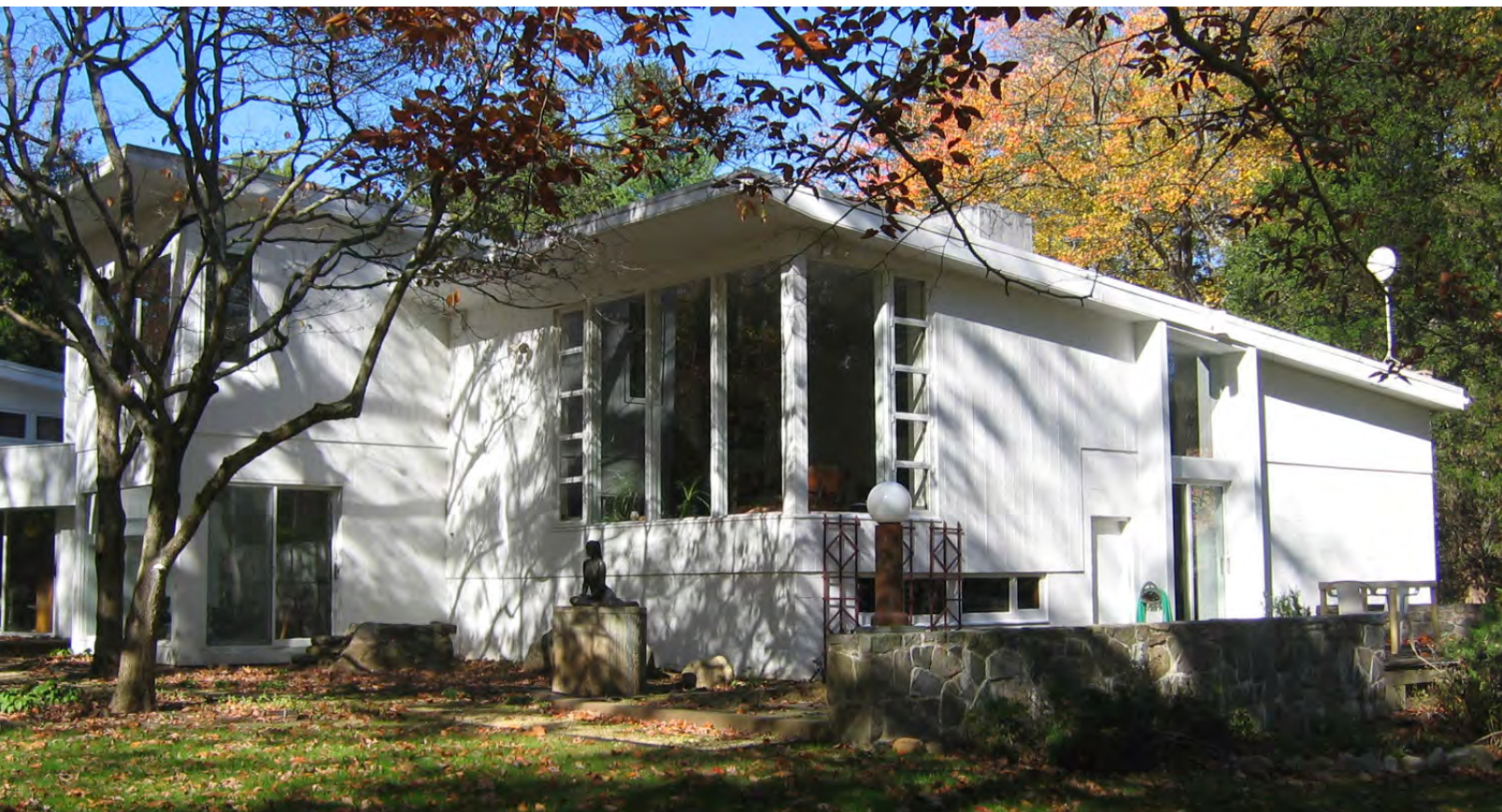
Kehm House, side and rear façades of original house, November 2007 (photographer: Eileen Brackenbury)
