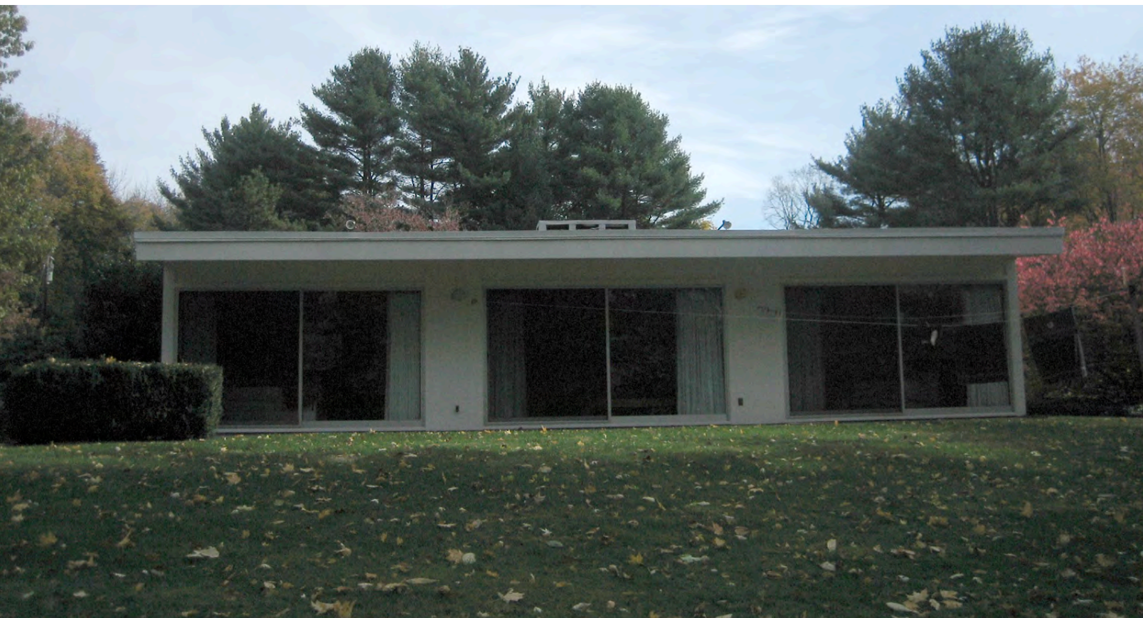
Rogers House, side façade at bedroom wing, November 2007 (photographer: Eileen Brackenbury)
