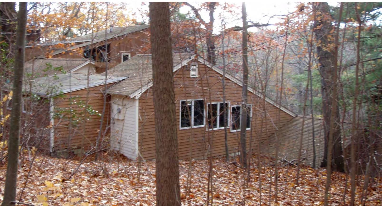
Papp House, side façades, 1959 additions, November 2007 (photographer: Martin Skrelunas)
