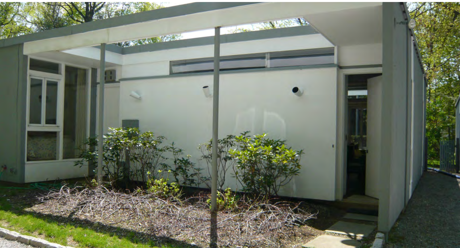
Attwood House, detail of courtyard at front façade, May 2008 (photographer: Martin Skrelunas)
