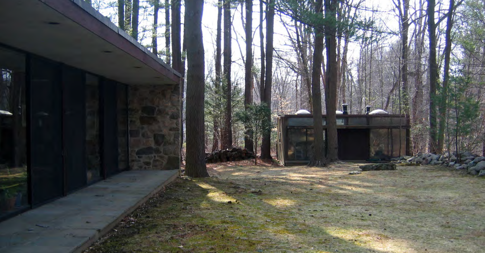
Noyes House 2, west façade and studio, October 2007 (photographer: Heather McGrath)
