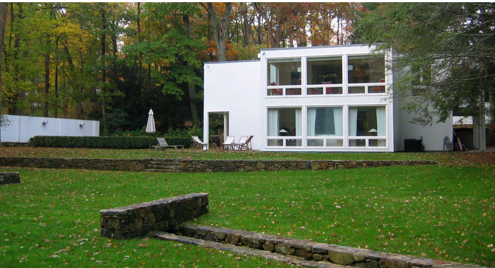
Gratwick House, rear façade showing addition and landscape features, November 2007 (photographer: Allyson Mehley)
