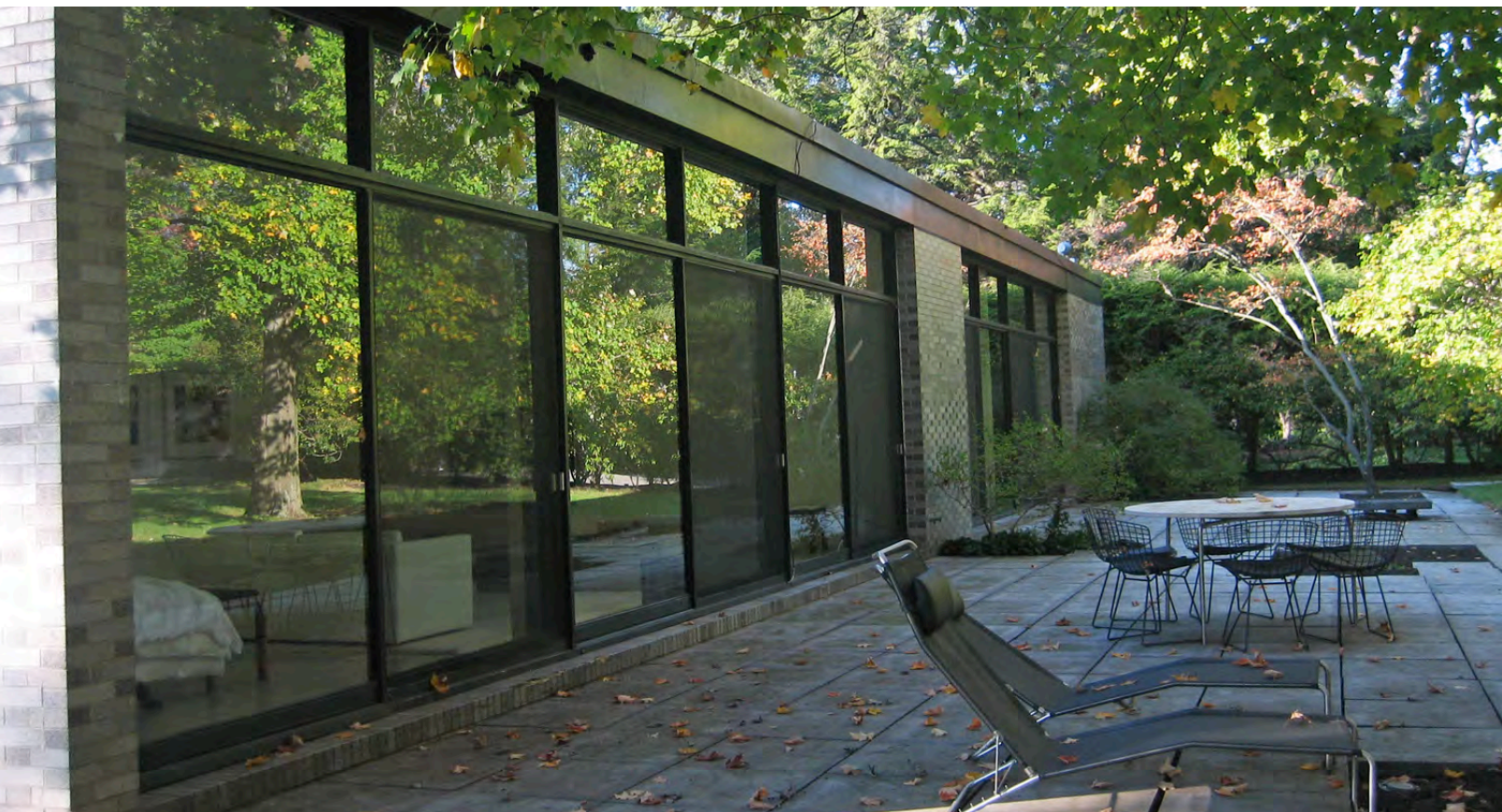
Hodgson House, bedroom wing, October 2007 (photographer: Eileen Brackenbury)
