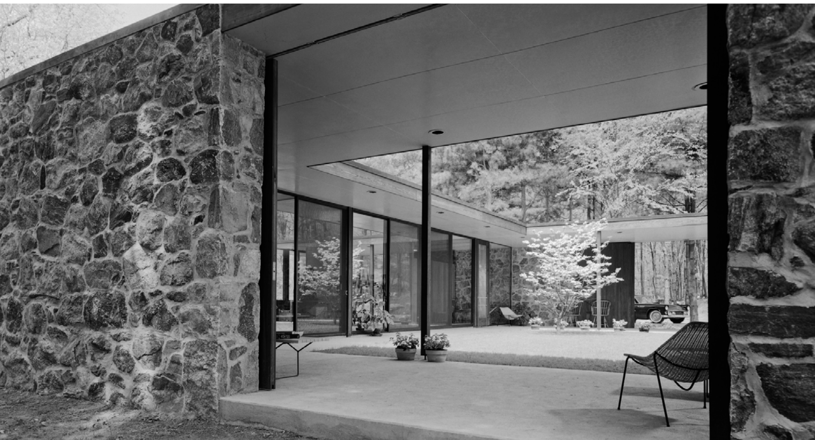
Noyes House 2, historic view of courtyard, unknown date (photographer: Ezra Stoller, source: Philip Johnson Glass House)
