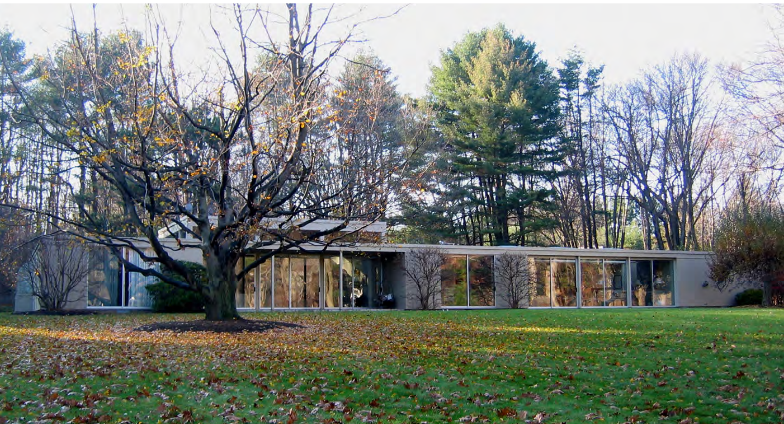
Ford House/Edward Winter House, rear façade, November 2007 (photographer: Eileen Brackenbury)
