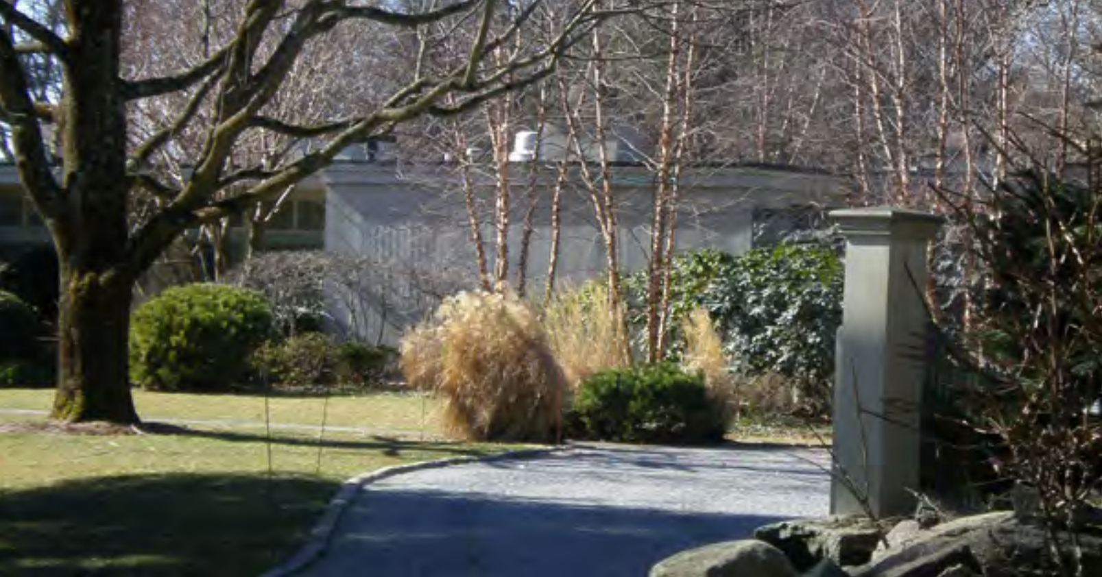
Kirkpatrick House, view from street, February 2008 (photographer: Allyson Mehley)
