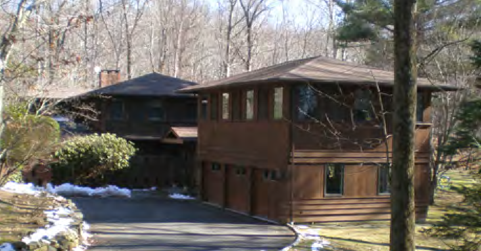
Alcoa House, view from street showing garage addition at right, February 2008 (photographer: Allyson Mehley)
