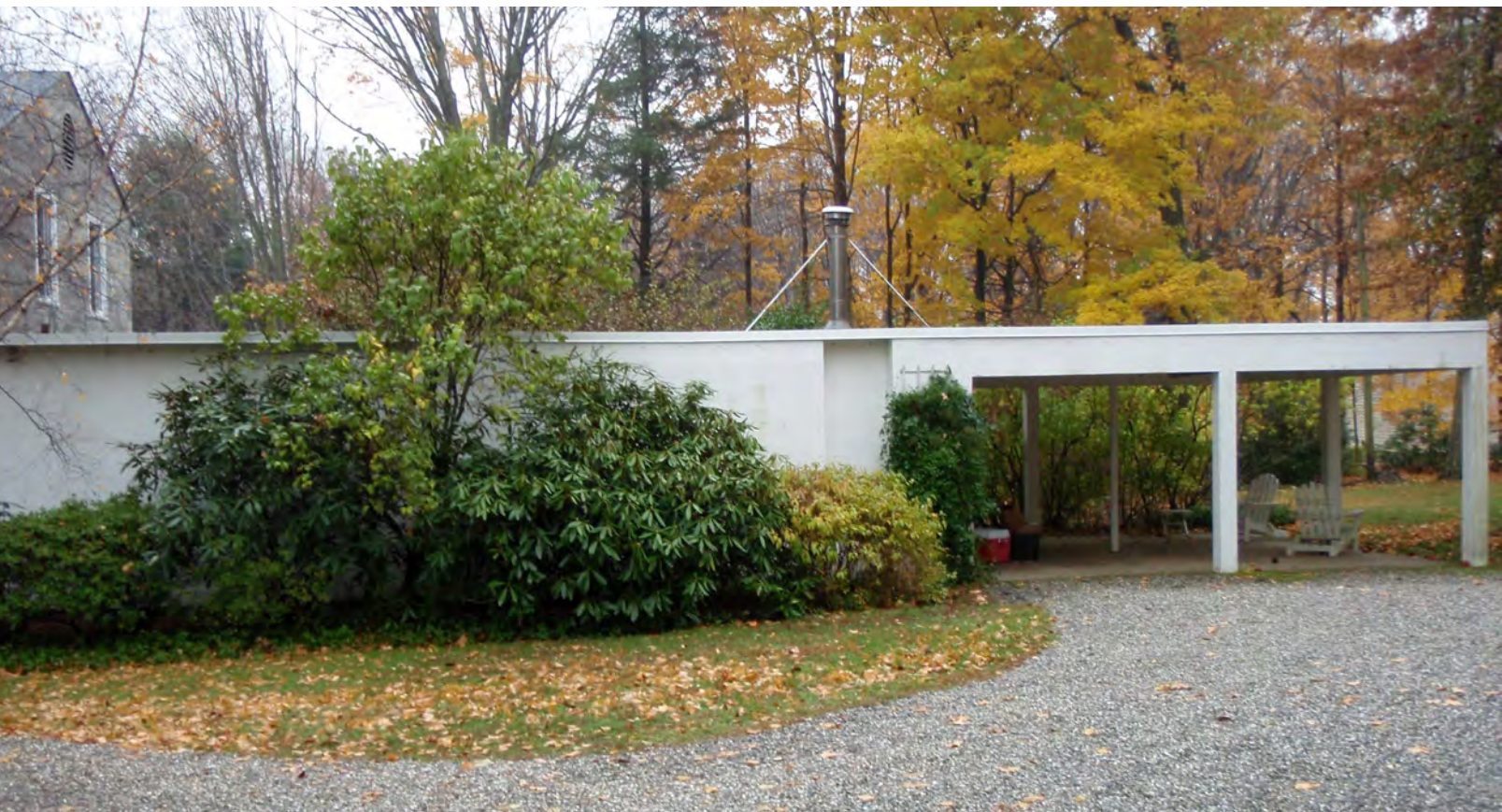
Mills House 1, view of carport from street, November 2007 (photographer: Martin Skrelunas)
