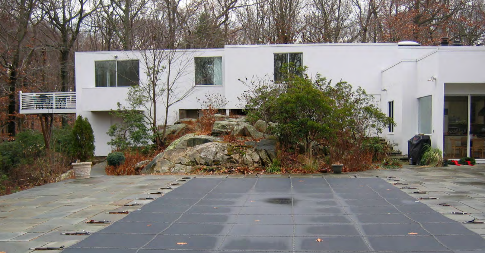
Arlt House, side façade, December 2007 (photographer: Eileen Brackenbury)
