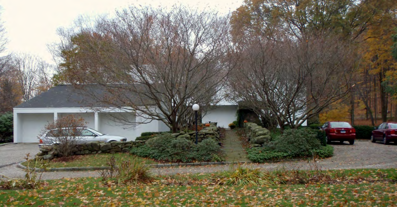
Weeks House, entry walkway and garage addition, November 2007 (photographer: Martin Skrelunas)
