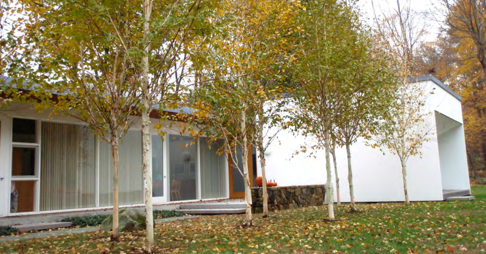
Tatum House, primary façade, November 2007 (photographer: Martin Skrelunas)
