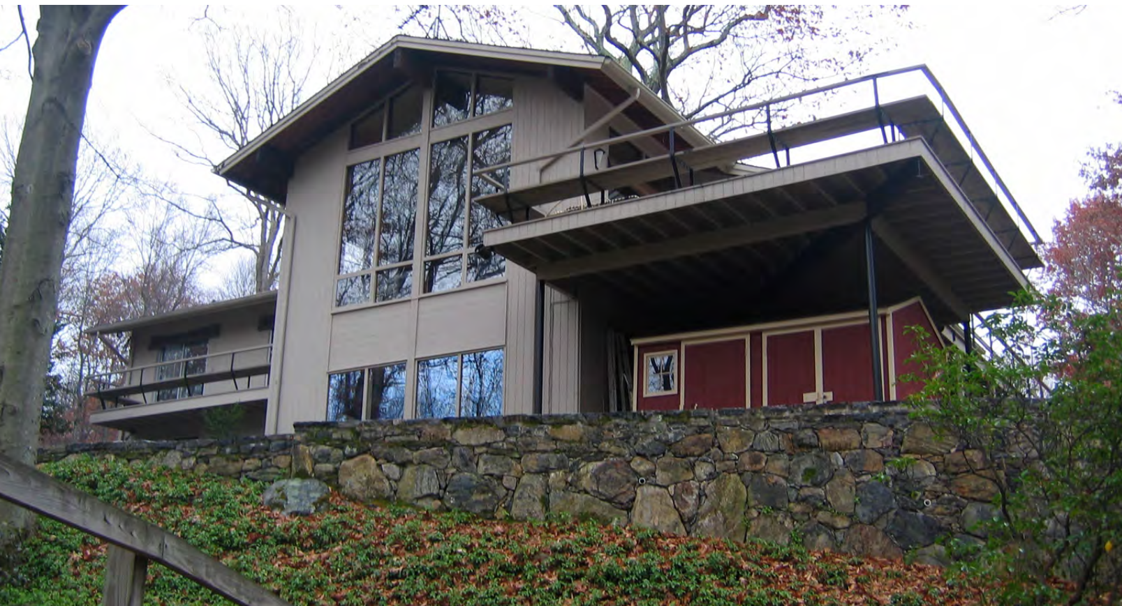
Amato House, rear façade, November 2007 (photographer: Eileen Brackenbury)
