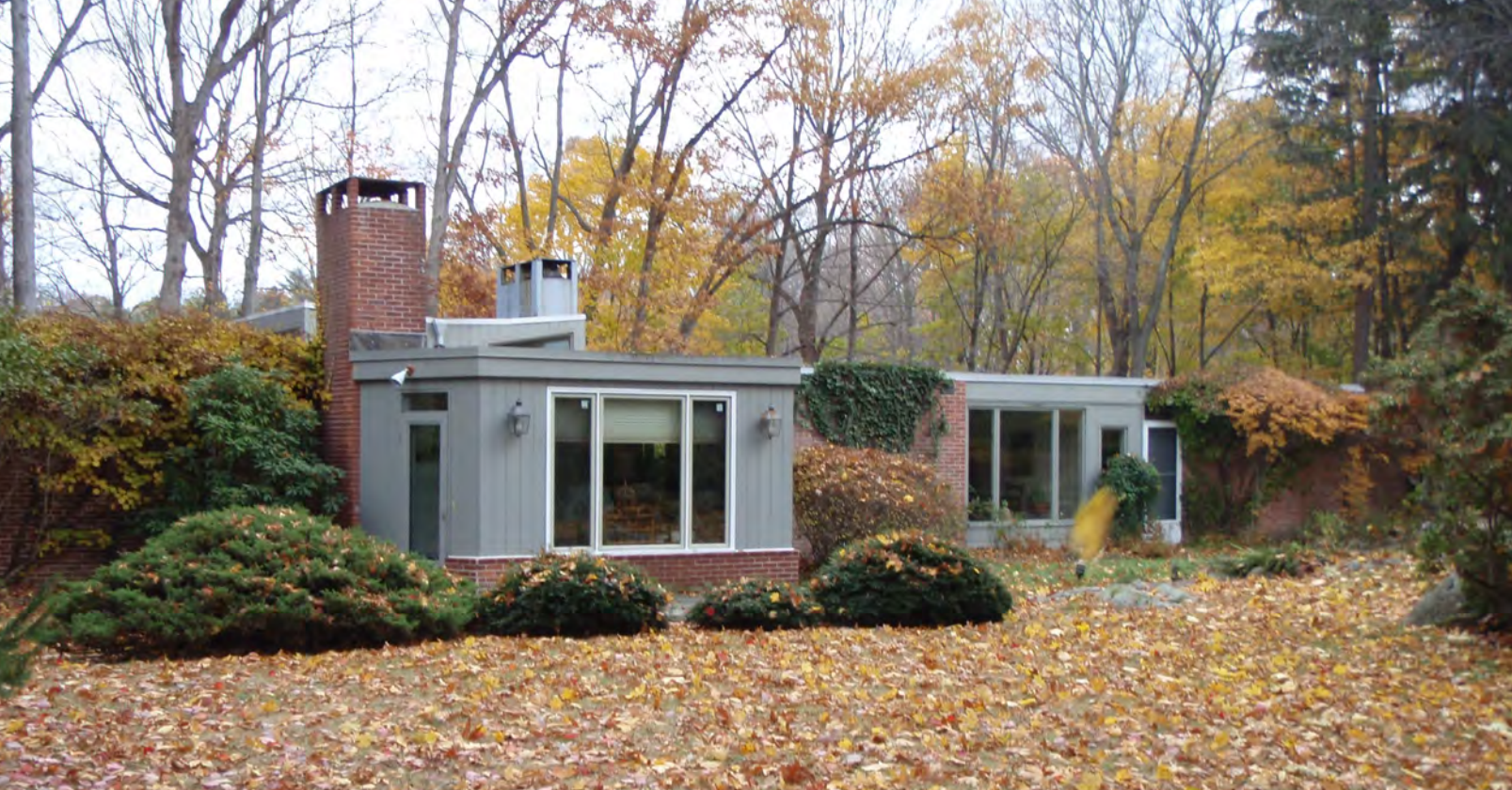
Roles House, side façade, November 2007 (photographer: Heather McGrath)
