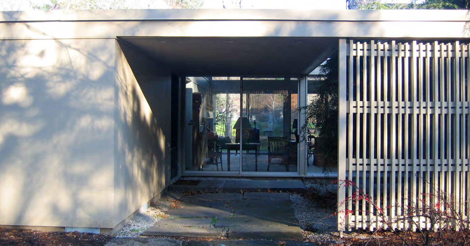
Ford House/Edward Winter House, detail of entry courtyard, November 2007 (photographer: Eileen Brackenbury)
