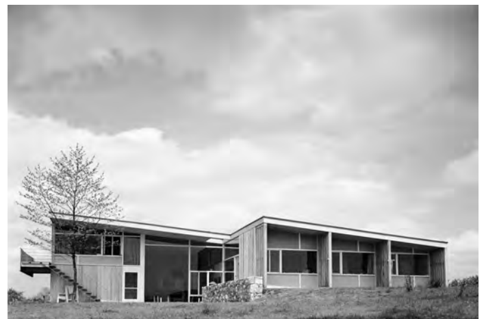
Figure 7. Kniffen House (1949, no longer extant), designed by Marcel Breuer and Eliot Noyes (photographer: Wayne Andrews, source: Philip Johnson Glass House)
