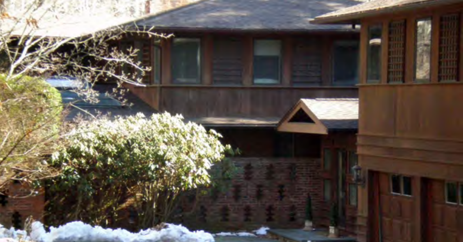
Alcoa House, view from street, February 2008 (photographer: Allyson Mehley)
