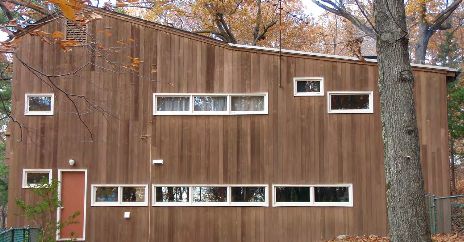
Papp House, side façade, 1964 addition, November 2007 (photographer: Martin Skrelunas)
