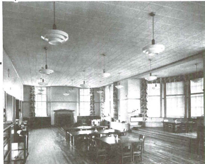
Ultra-modern kindergarten, Meeker Grade School, Puyallup, Washington, showing Simpson Acoustical Tile installation. Similar installations were also made in all other classrooms and corridors in the new school addition.
