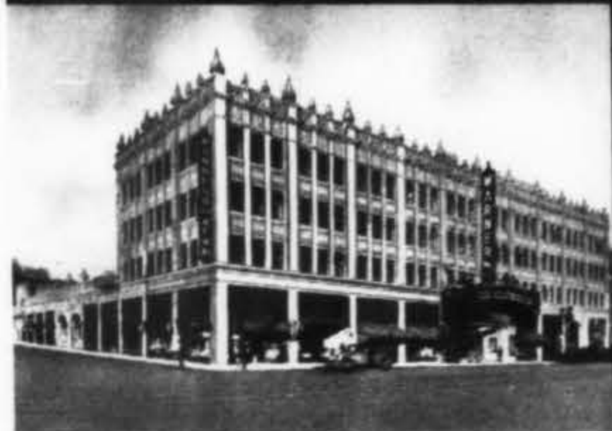
In Warner Brothers Theater, Los Angeles, Calif., both the elevator and metal swing doors are by Dahlstrom.
