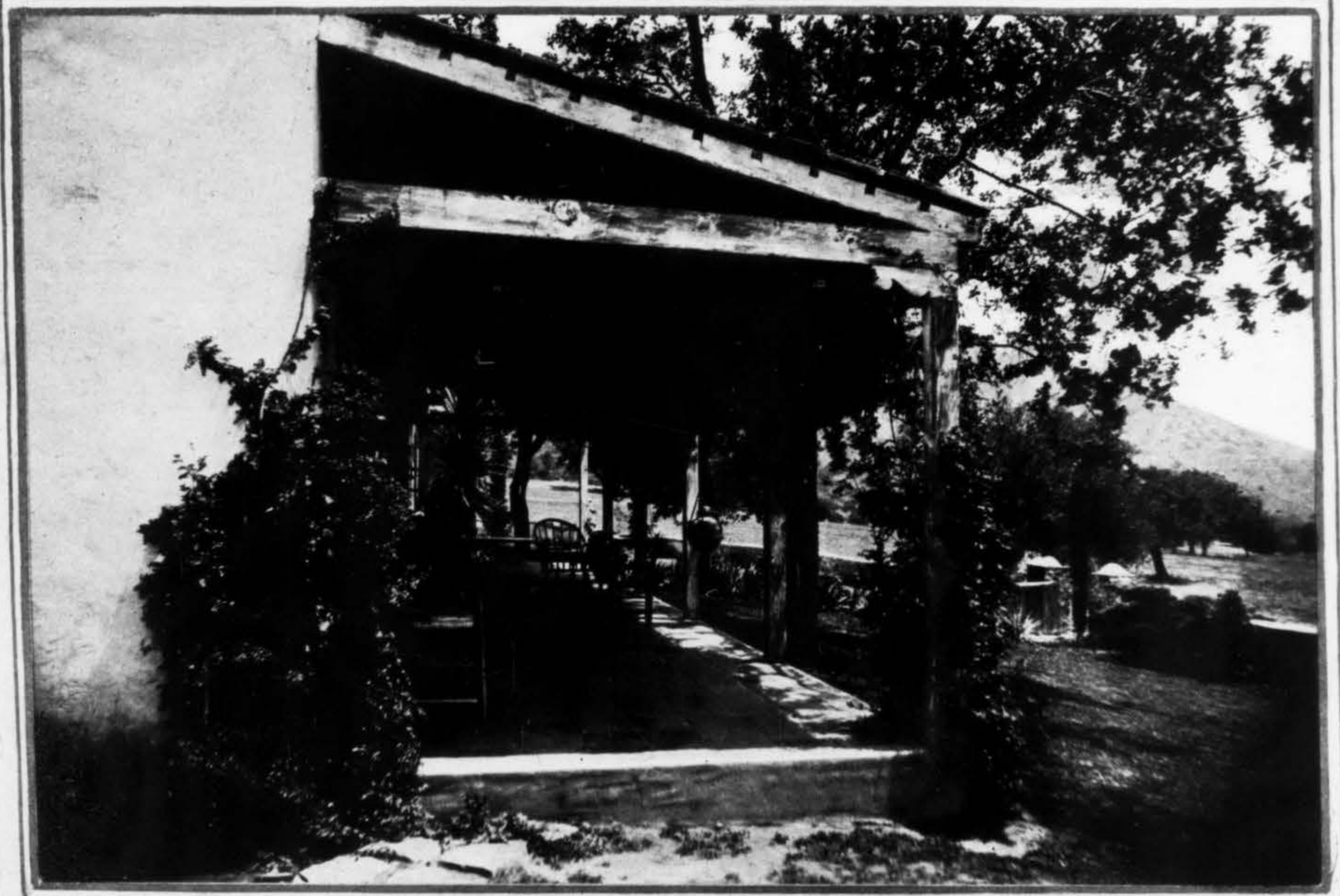
An Adobe Ranch House for Major French at Las Turas Lake. John Byers, Architect
