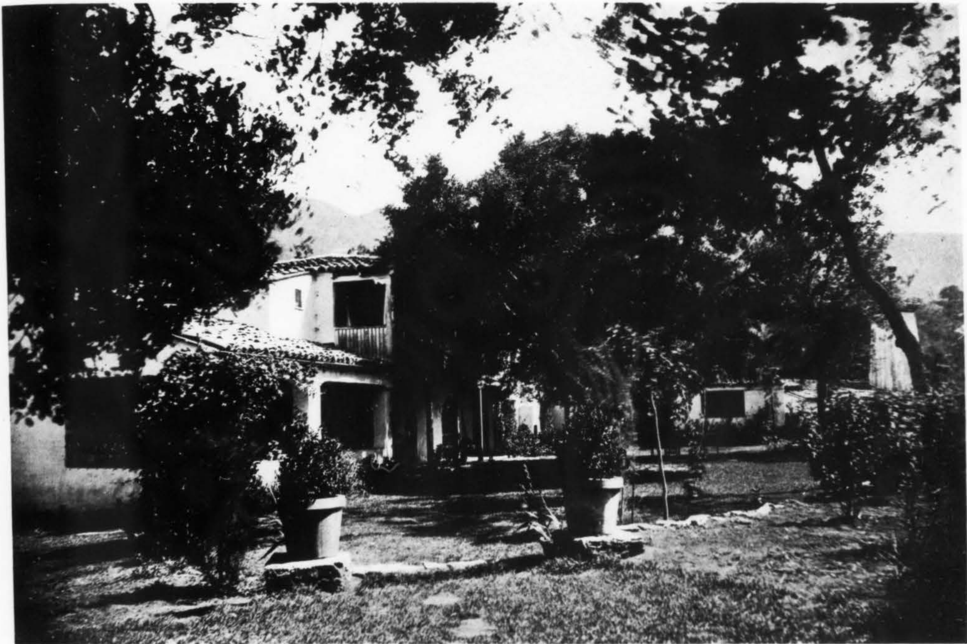
The walled garden behind the ranch house of Major French has been treated by his architect, John Byers, as a definite part of the family living quarters.
