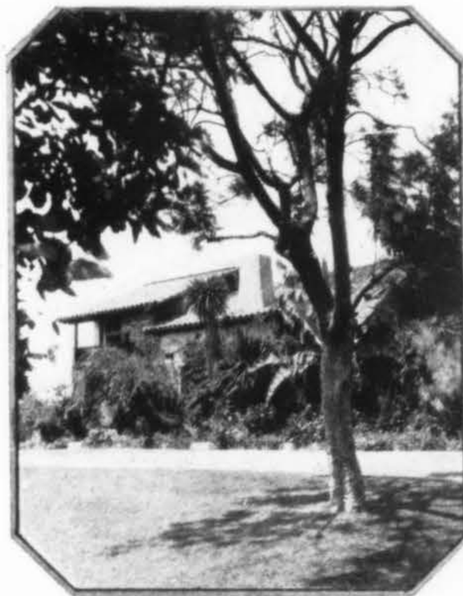
An adobe house for Mr. H. R. Johnson, at Brentwood Park. John Byers, Architect
