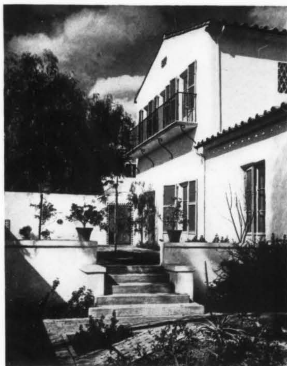
The Living Room Terrace, Clark Hall
