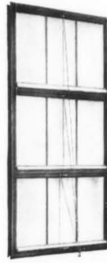
All three sash closed and weathertight.
