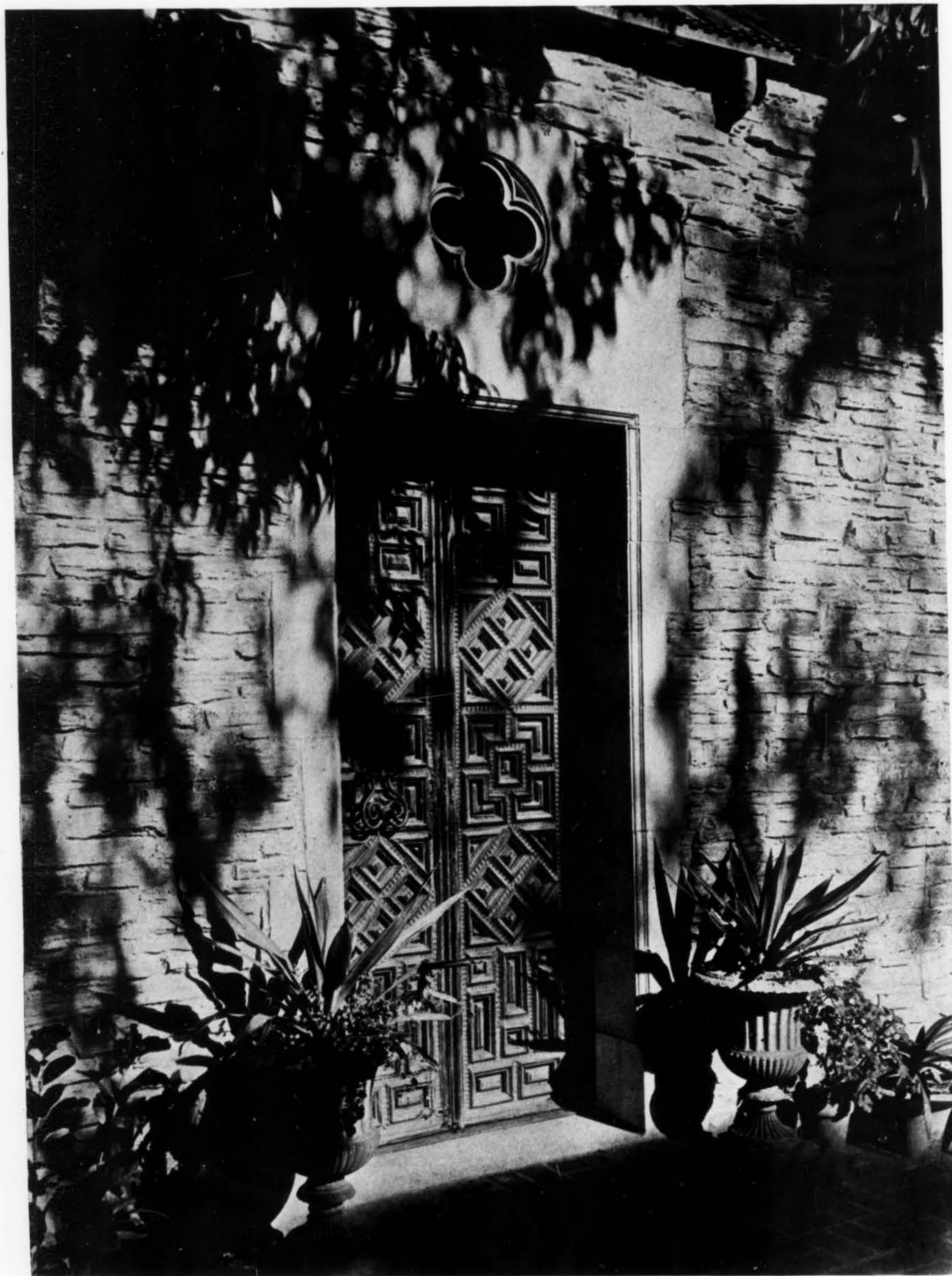
A close view of the main doorway to the home of Garrett Van Pelt, Jr., architect; this shows not only the exceedingly lovely door itself, with its richly molded panels and wrought iron knocker, but also the texture and scale of the stonework, the skillful use of long narrow slabs with not too much variation for the size of the house.
