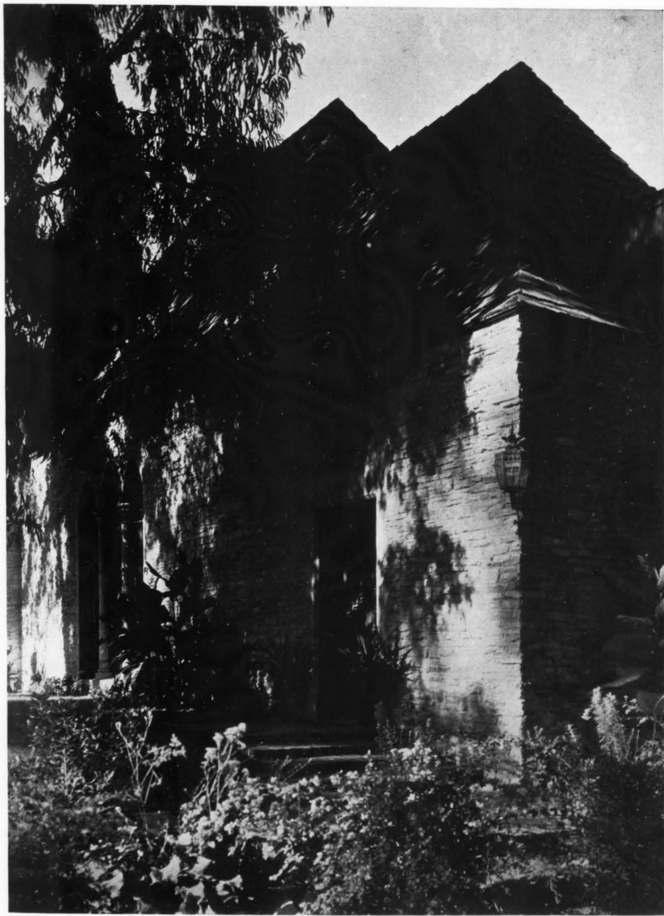
The relation of wall and roof has been studied carefully in the home Garrett Van Pelt, Jr., has built for himself in Pasadena. Noteworthy also is the treatment of brick terrace and steps at the entrance, and the part played by two urn-shaped flower pots in the composition of the doorway, with its quatre-foil opening overhead. The corner lantern is congruous, useful, and a thing of lovely craftsmanship.
