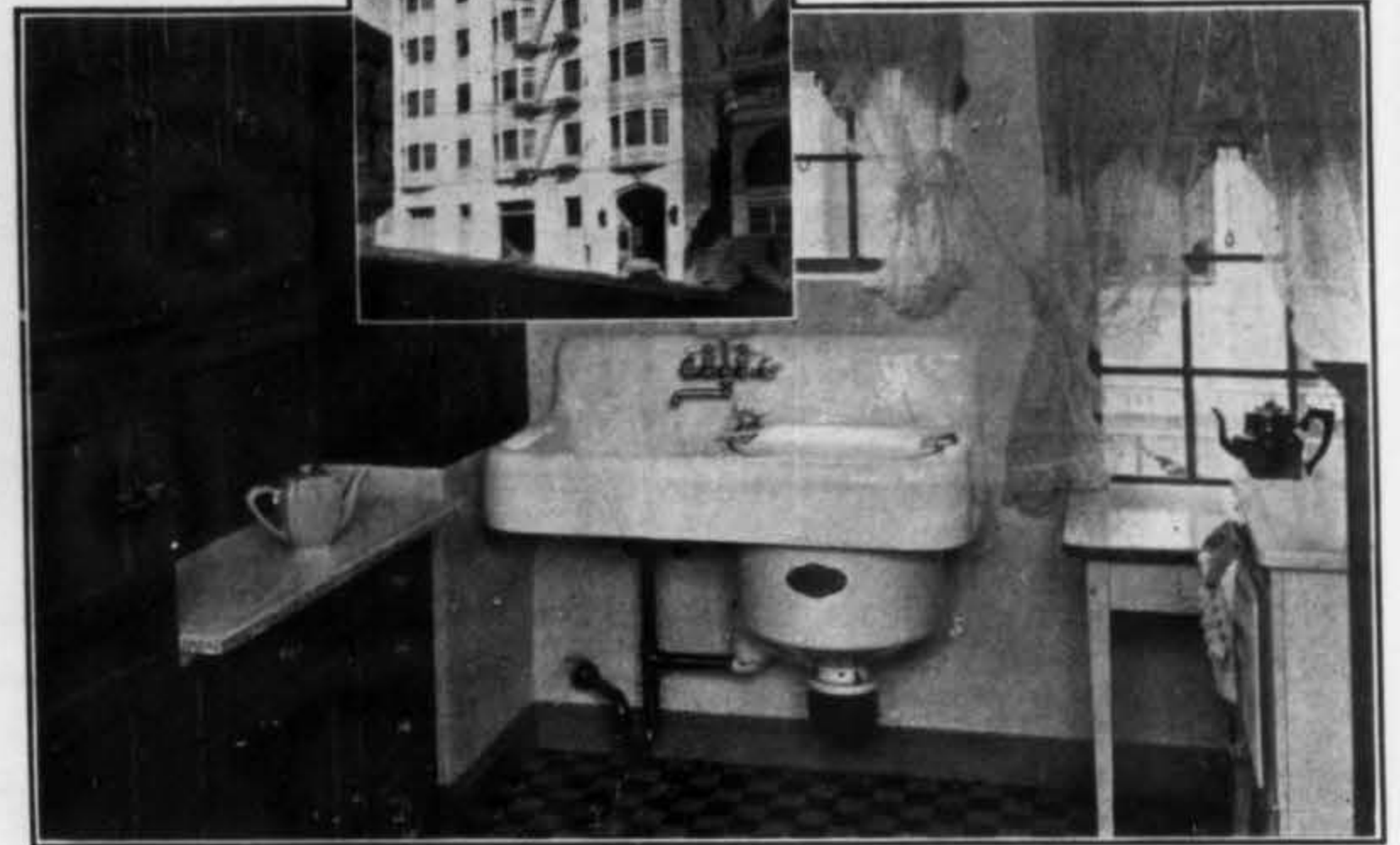
WALKER Electric Dishwasher Sink, Model 114-R, installed in the kitchens of the Pine-Grove Apartments, San Francisco.
