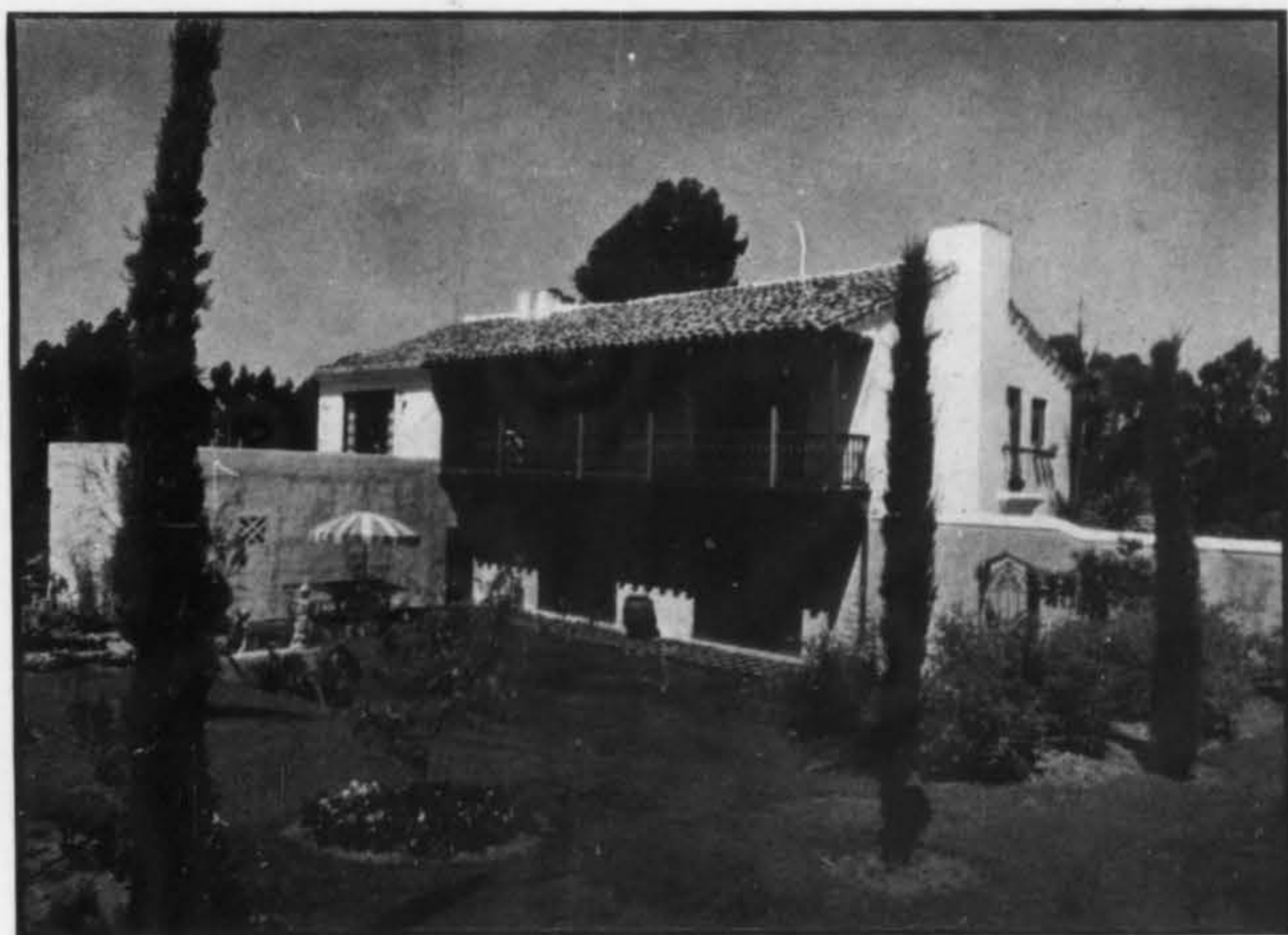
Views of the fore-court and central garden, residence of Mr. and Mrs. Dean S. Arnold, Hillsboro, California; Gardner Dailey, architect. A free, vigorous treatment has been used, drawing upon both early Californian and Hispanic sources for inspiration, and clearly suited to the life and climate of its location
