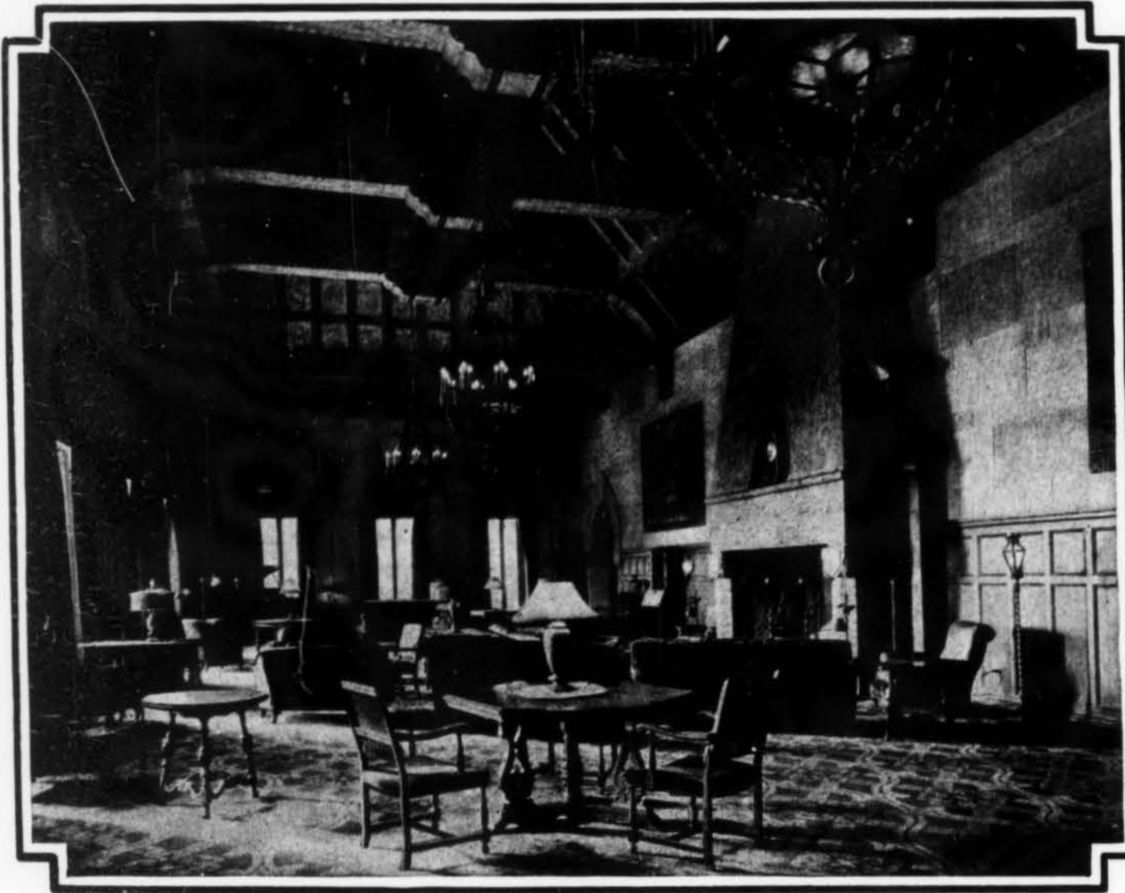
Trusses of reinforced concrete, richly decorated, provide a picturesque and traditional beauty in the lounge of the Pacific Coast Club, Los Angeles.
