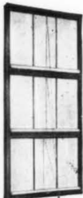
All three sash closed and weather-tight.
