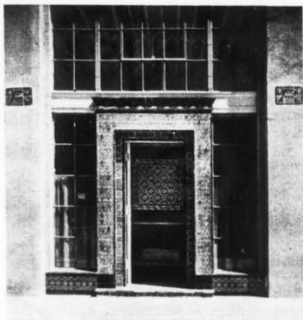
Entrance Detail, San Francisco Rossman Warehouse
