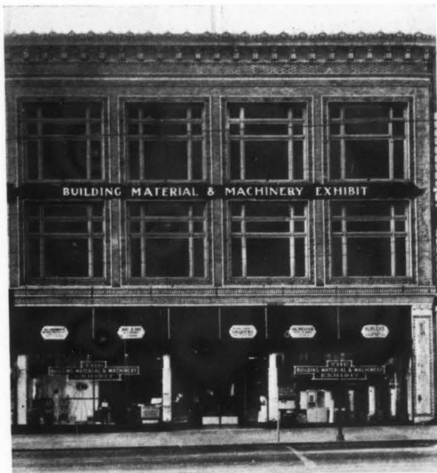
An entire three-story building of 40,000 square feet devoted to displays of modern building materials
