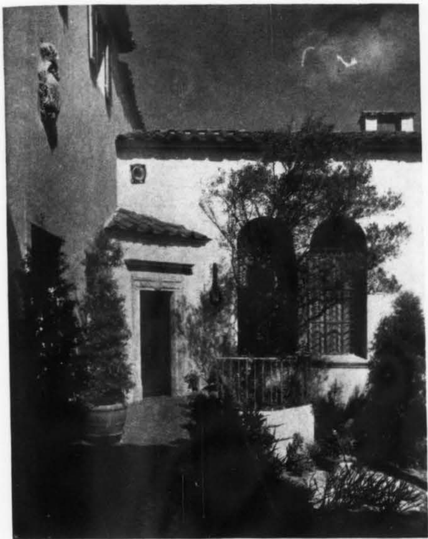
Above is a corner of the central court in Mr. Eisner's residence, showing a door and one of the mullioned windows of the great banquet hall.
