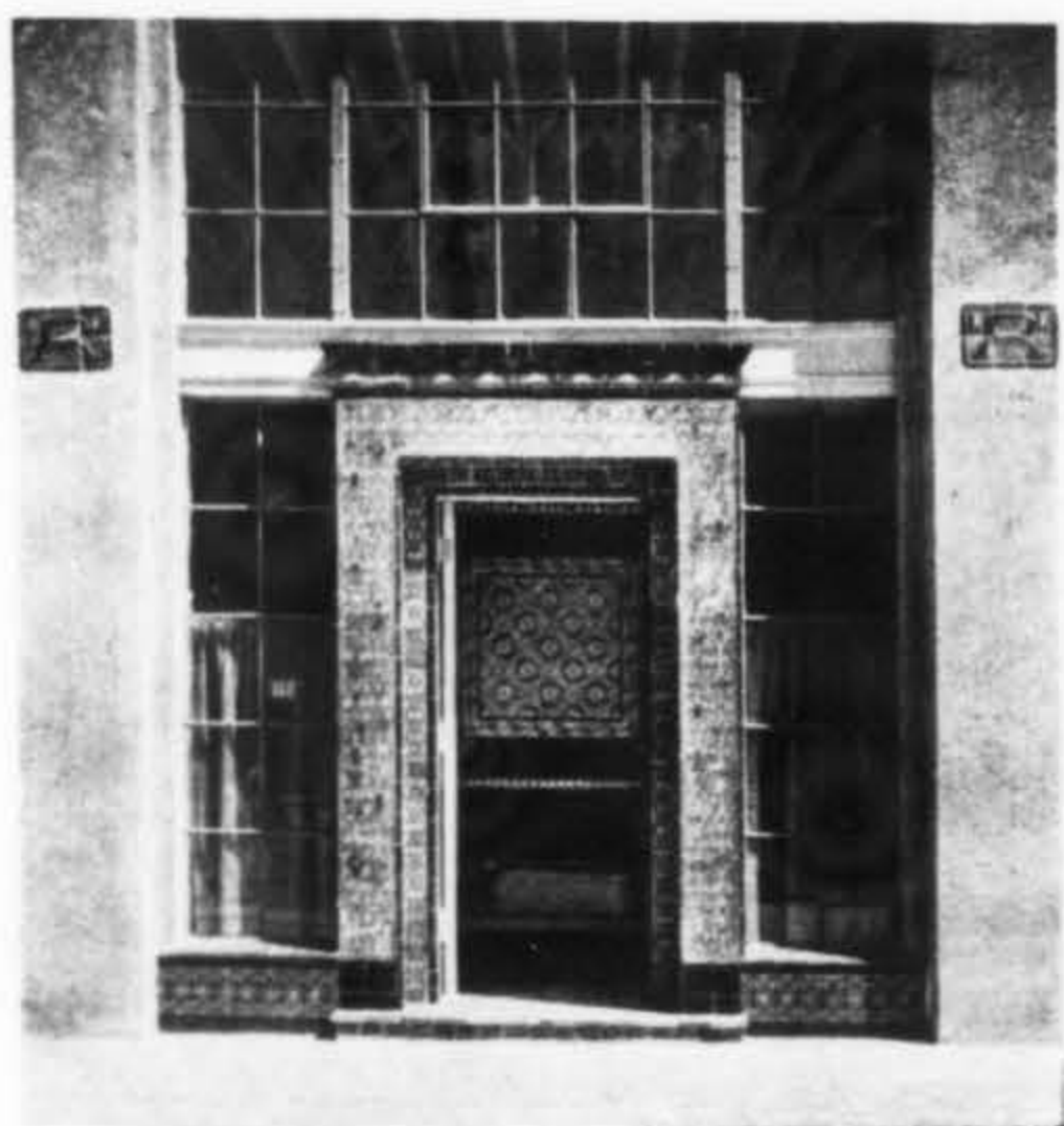
Entrance Detail, San Francisco Rossman Warehouse
