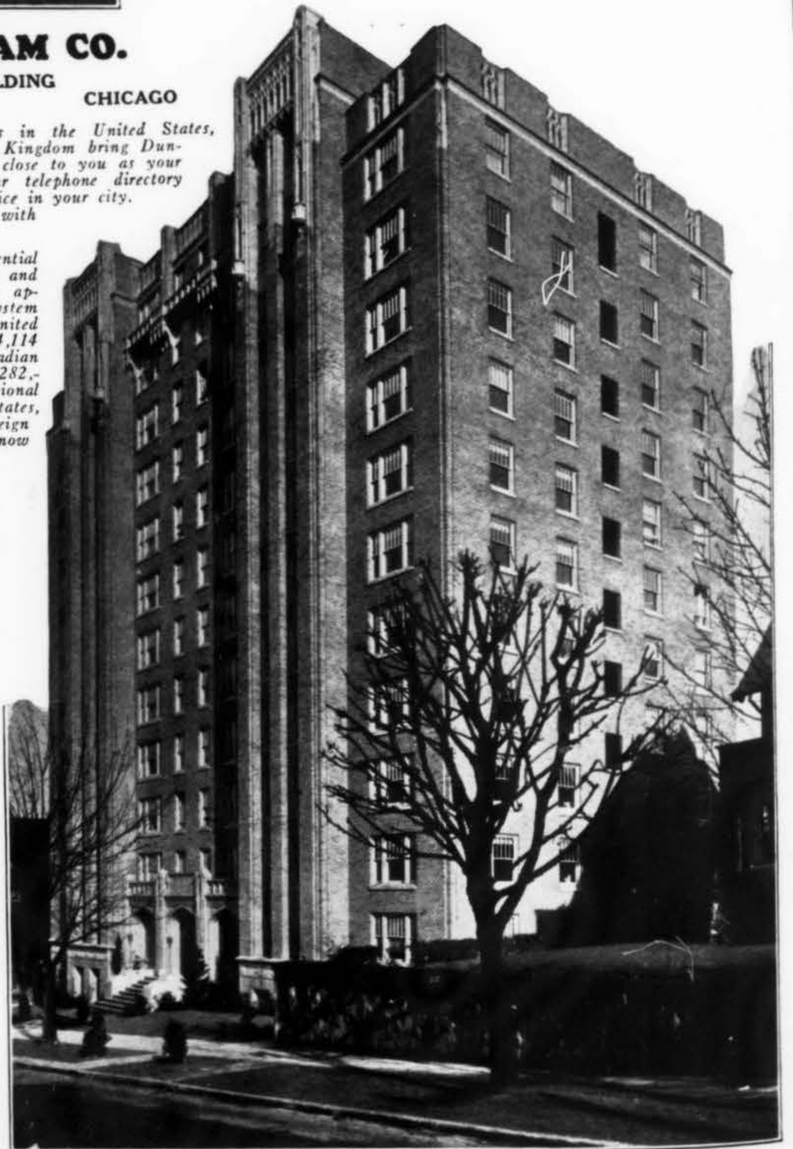
MARLBOROUGH HOUSE, SEATTLE
