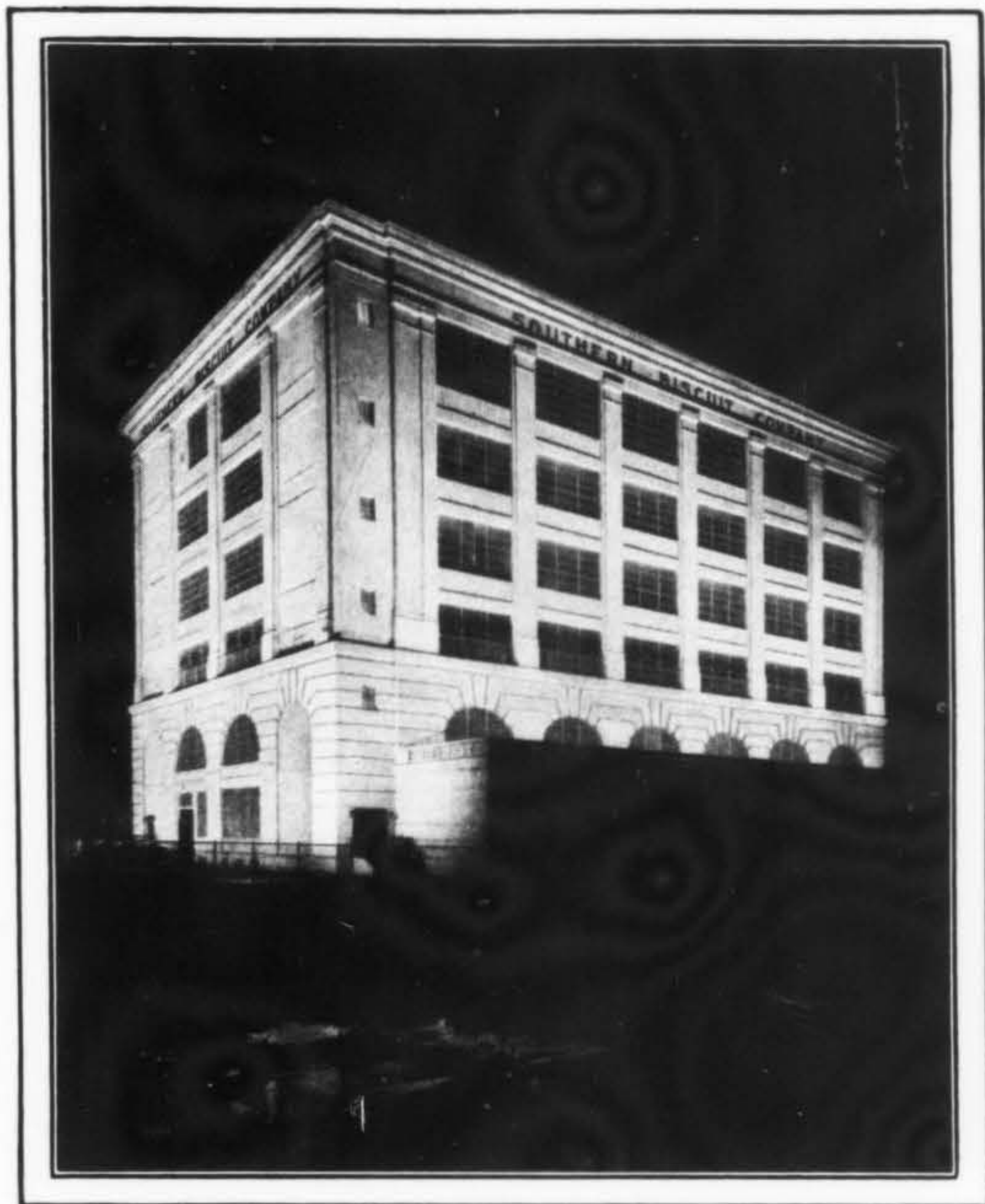
This modern factory building, the plant of the Southern Biscuit Works at Richmond, Va., demonstrates the combination of true beauty with the purely practical in reinforced concrete construction. The picture at the left shows also how splendidly a concrete exterior lends itself to flood lighting. Francisco and Jacobus, Architects, New York City
