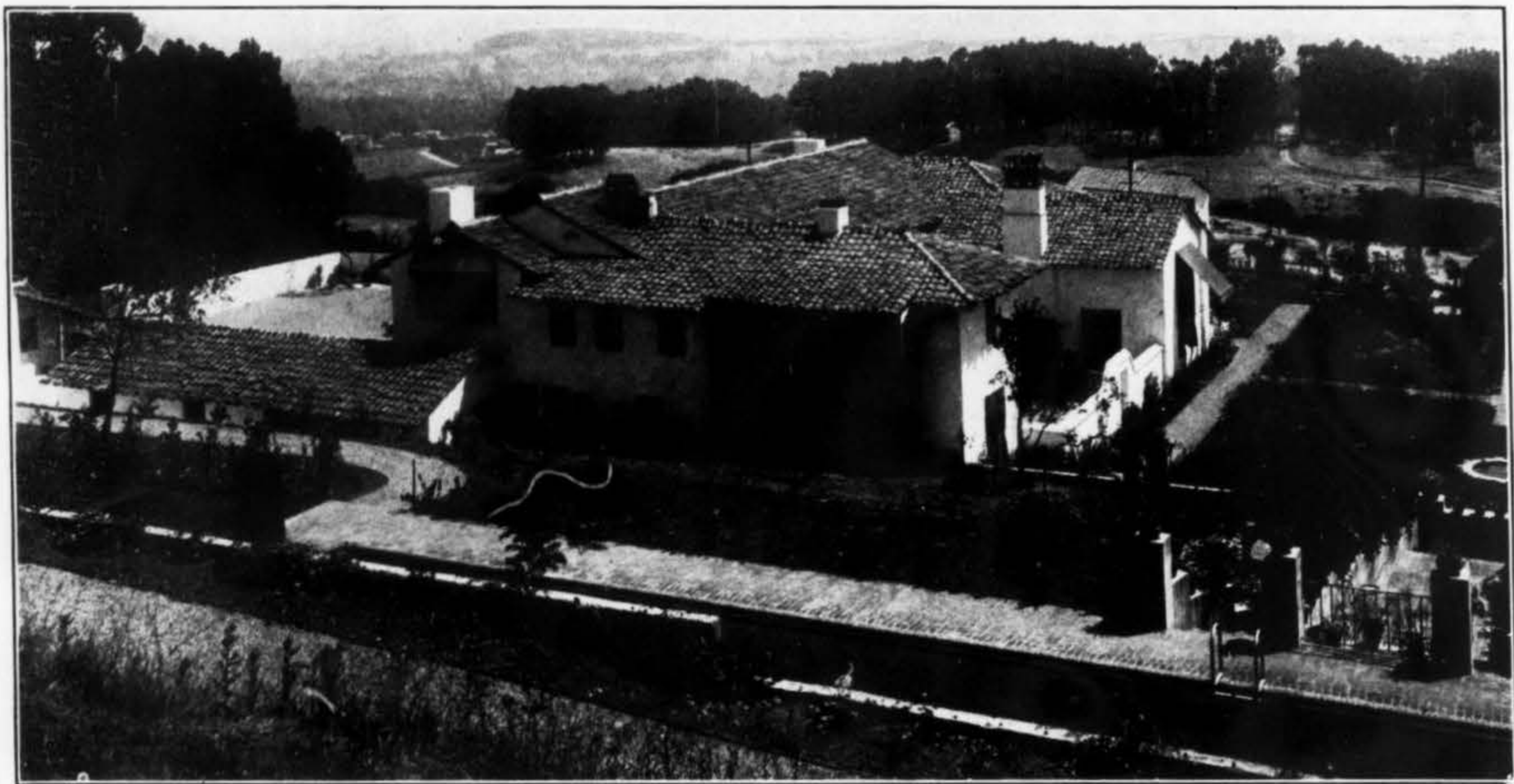
The residence of Mr. and Mrs. Walter B. Brandt, in Hillsborough Park, Clarence A. Tantau, Architect, commands a superb view of the bay and surrounding country.
