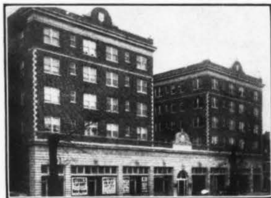
80,000 sq. ft. of STEELTEX FOR FLOORS strengthen and protect this attractive apartment building, 4011 Delmar Blvd., St. Louis, Mo. STEELTEX FOR FLOORS functions as a combined reinforcing and concrete form—saving time, labor, material, and money. Shipped in rolls, it is quickly attached to any type of joist or beam, and affords safe walking surface during pouring of concrete.
