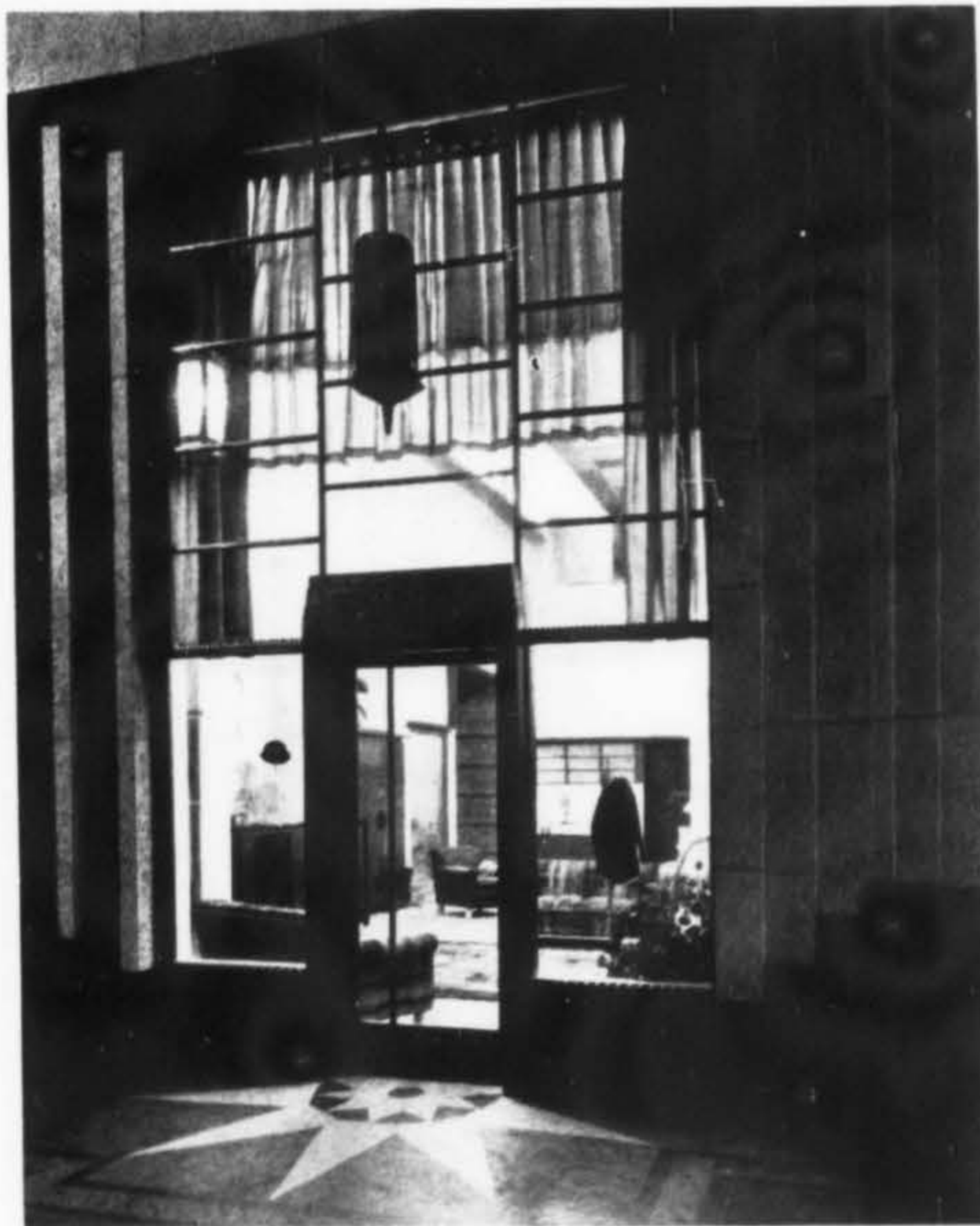
Looking into the Saddle Shop from Wilshire Boulevard
