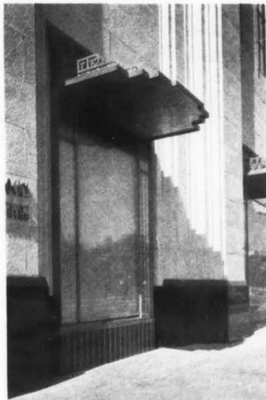
Each show window is a picture, framed and sheltered by crisply moulded and etched lines and surfaces of bronze.
