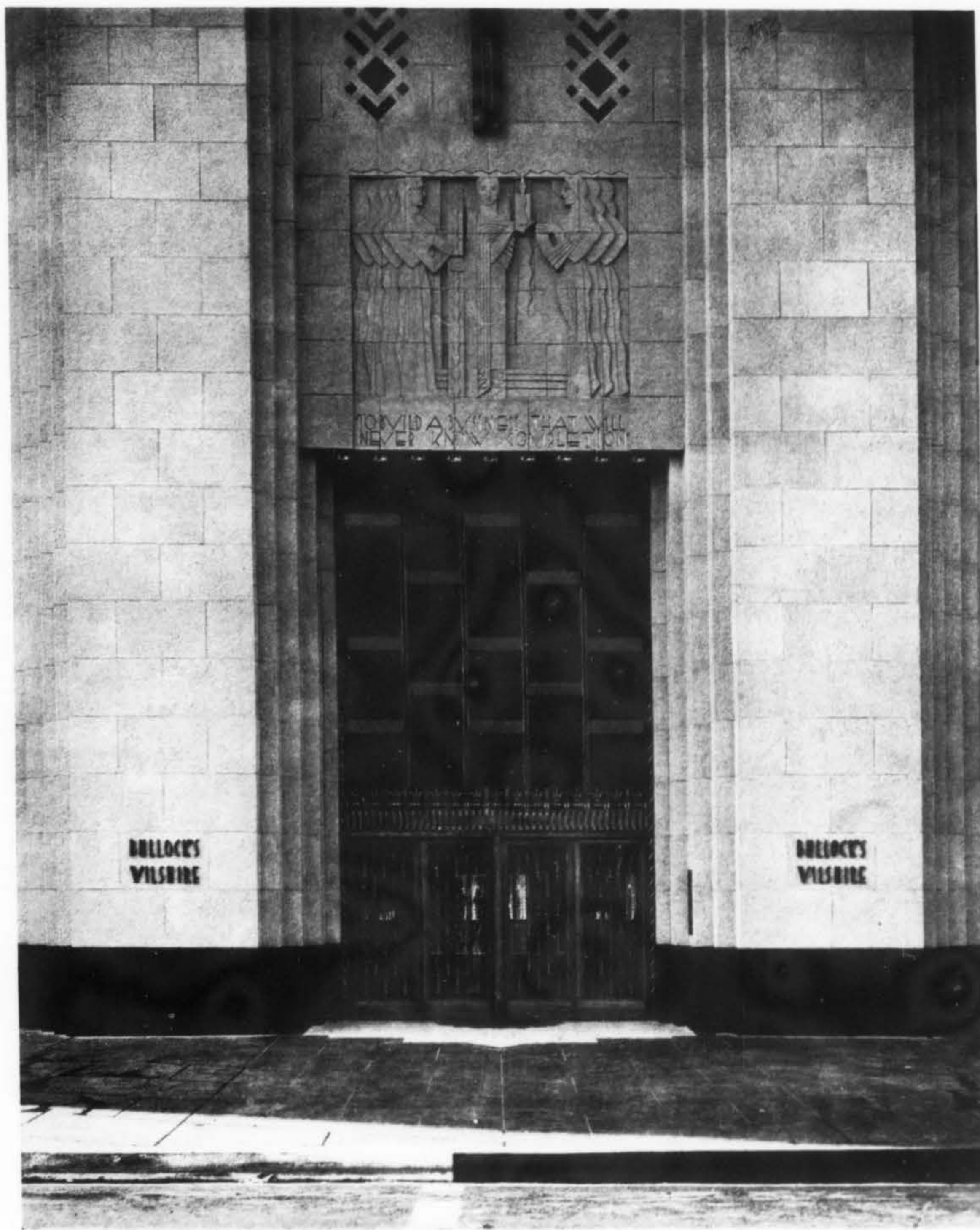
BULLOCK'S WILSHIRE STORE, Los Angeles JOHN PARKINSON AND DONALD B. PARKINSON, Architects P. J. WALKER COMPANY, Builders
