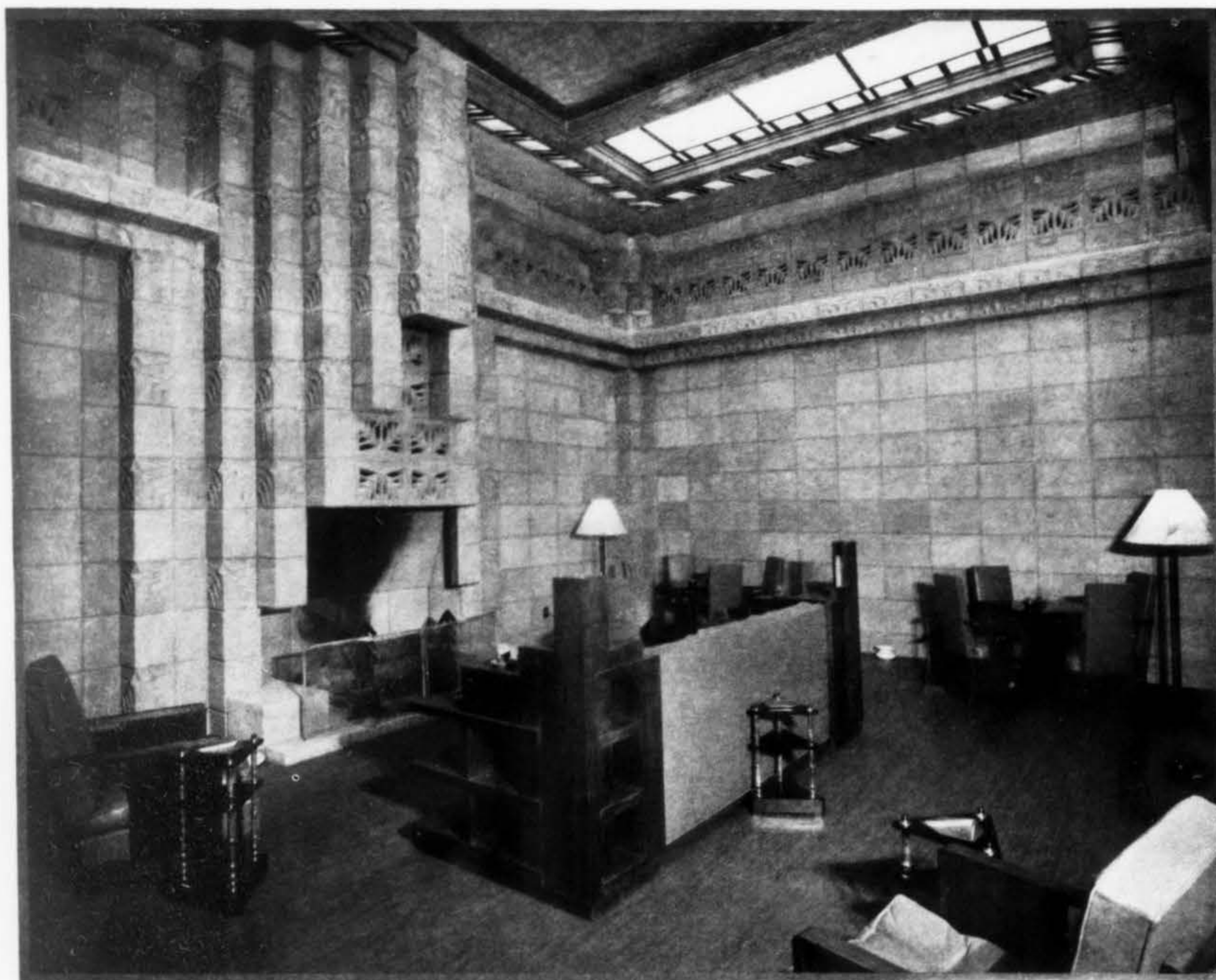
To the left, an inviting corner in the smoking room of Arizona-Biltmore Hotel, Phoenix, Arizona. Below, the unique exterior. Built of reinforced concrete, faced with cast stone blocks. Interior walls also of cast stone, in plain and conventional designs. Albert Chase MacArthur, Phoenix, Architect; Frank Lloyd Wright, Associate; S. M. Benet & Co., Beverly Hills, California, Contractors.
