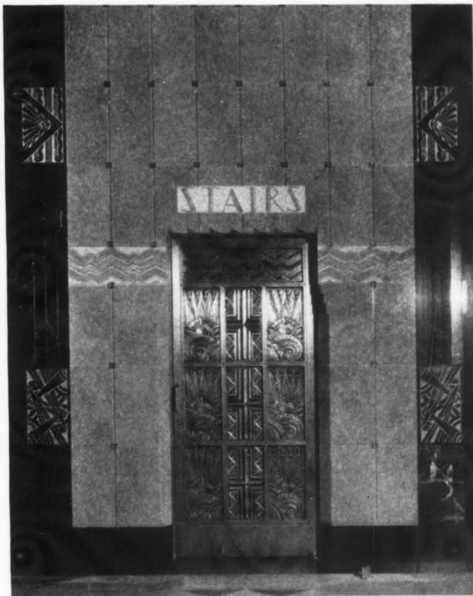
At the end of the elevator hall is a great panel of buff marble, and the inset stairway door of crisply modeled bronze.
