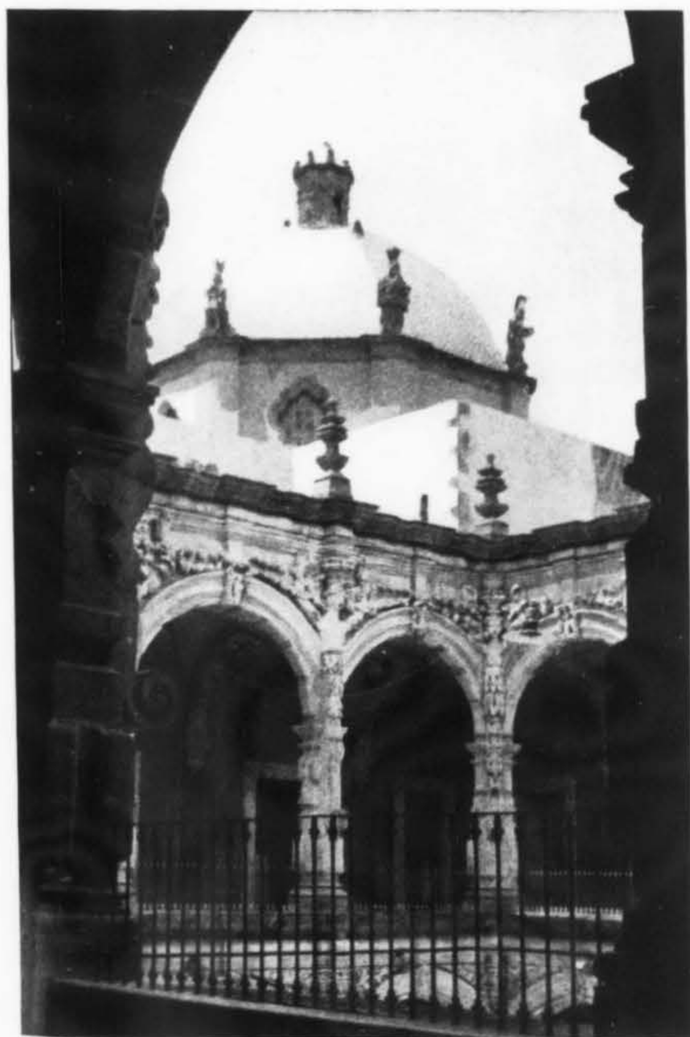
Courtyard, Municipal Palace of Queretaro, and dome of St. Augustin.
