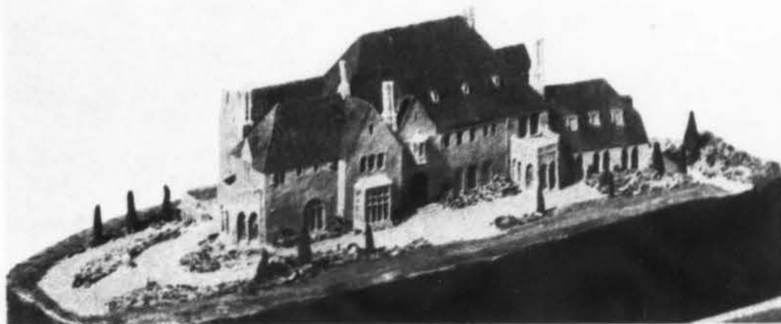
Model made by Miss Mesick for the residence of Mr. E. J. Sweetland Piedmont, California; Frederick H. Reimers, architect
