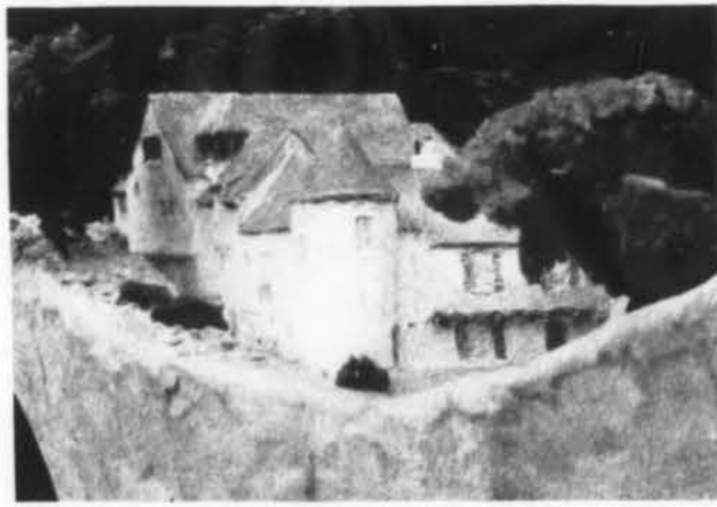
Residence of Mr. and Mrs. Milton E. Wise Piedmont, California; Leslie H. Lippiatt, architect
